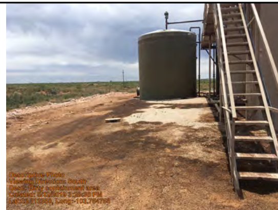
Dirty containment area
