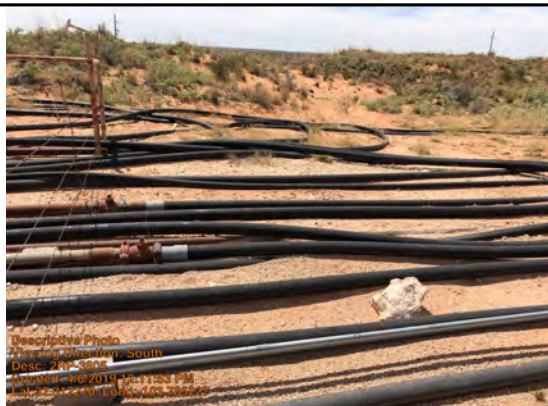
2RP-3805 and 2RP-1771 approximate spill area
