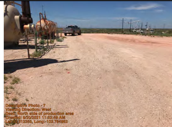
North side of production area
