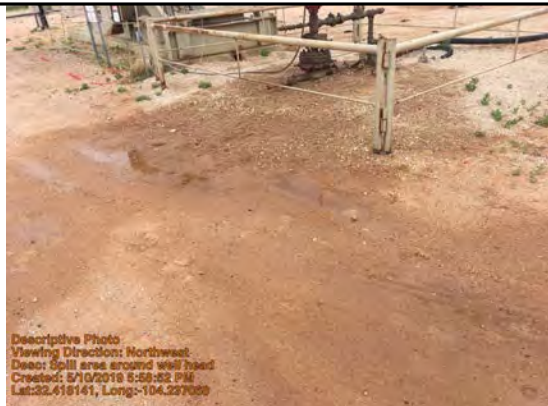
Spill area around well head
