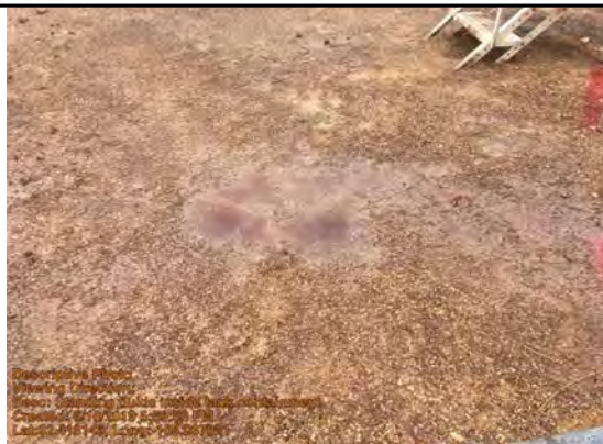
Standing fluids inside tank containment
