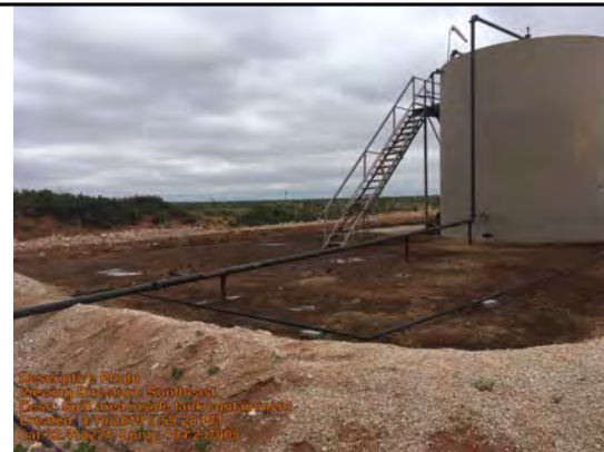
Spill area inside tank containment
