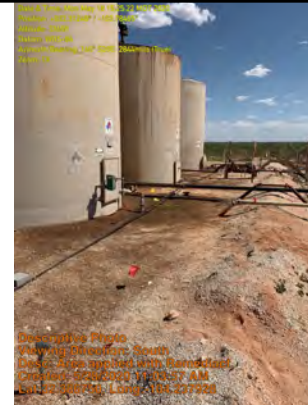
Area applied with Remediat
