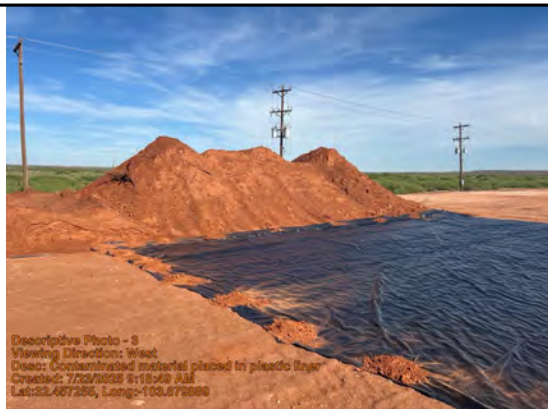
Contaminated material placed in plastic liner
