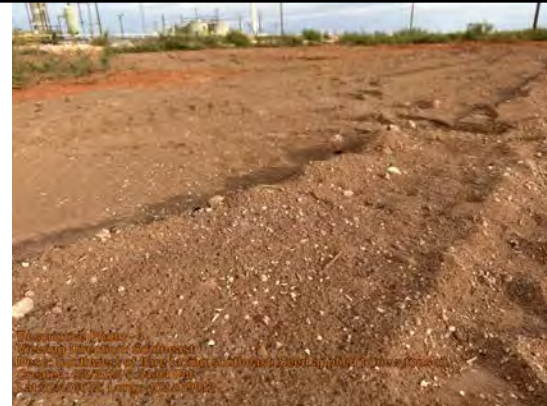
Southwest of flare facing southeast. Seed applied to new topsoil.
