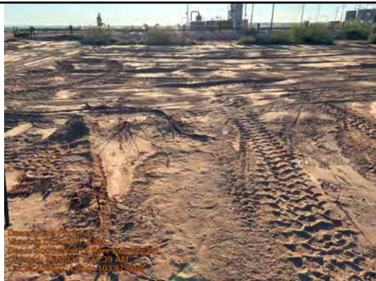
Southwest of flare facing east.
