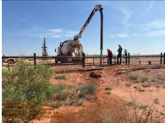
Hydrovac in progress
