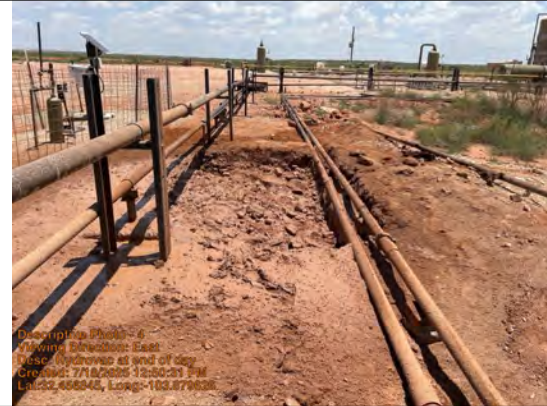
Hydrovac at end of day
