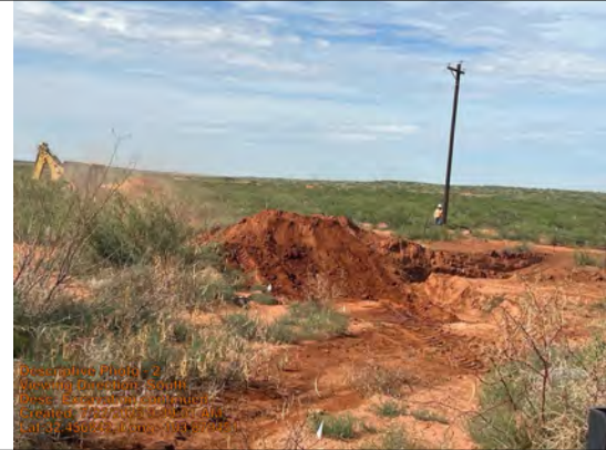
Viewing Direction: South
