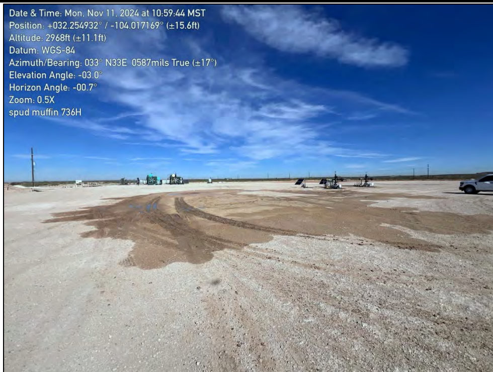
PHOTO 2: Northeastern view during initial site assessment activities. 11/11/2024
