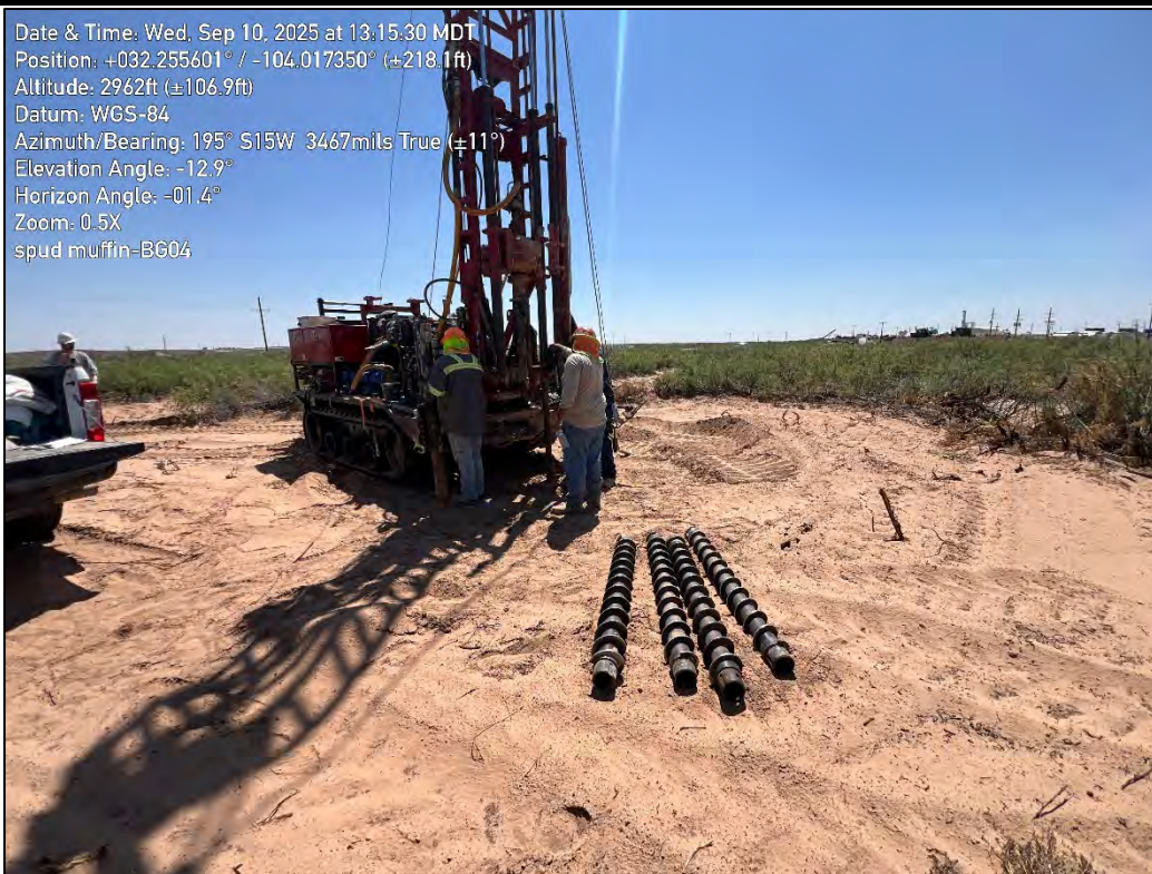
PHOTO 16: Southwestern view during background sampling activities. 9/10/2025
