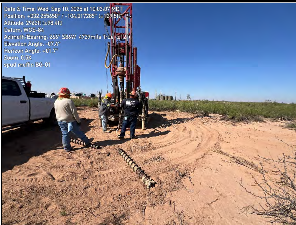
PHOTO 14: Southwestern view during background sampling activities. 9/10/2025
