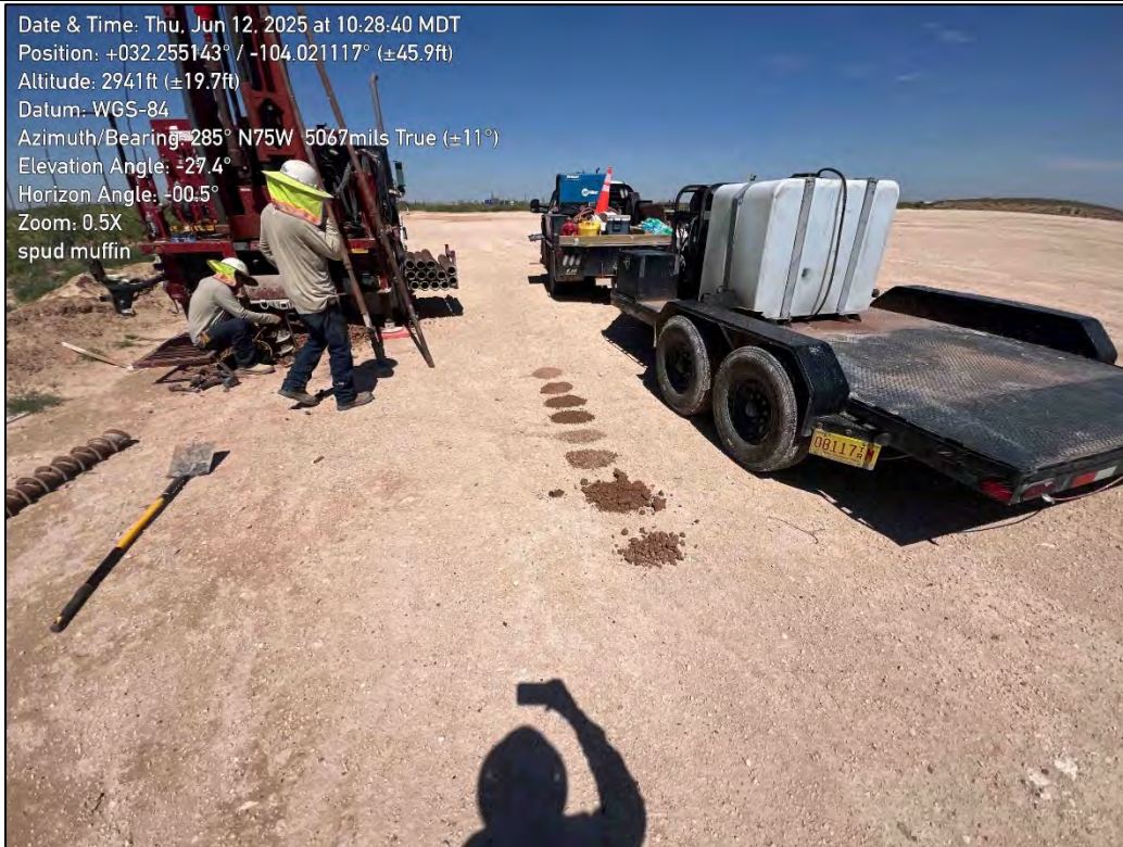
PHOTO 13: Northwestern view during DTW drilling. 6/12/2025
