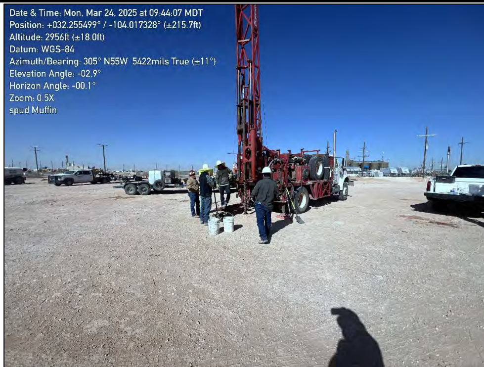
PHOTO 7: Northwestern view during additional delineation activities. 3/24/2025
