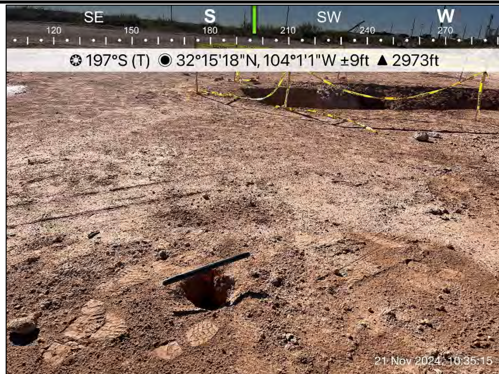
PHOTO 4: Southwestern view during initial delineation activities. 11/21/2024
