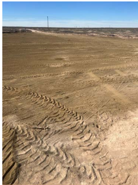
Photograph 4 Date: Feb-2025 Description: Backfilled excavation
