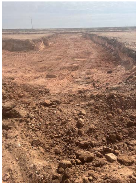
Photograph 4 Date: Feb-2025 Description: Final excavation extent
