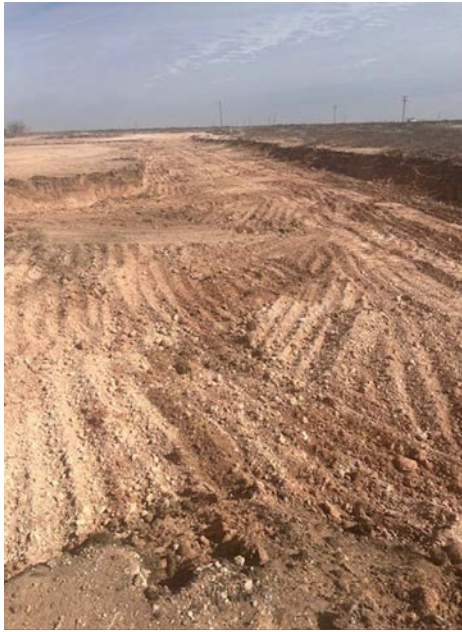
Photograph 1 Date: Feb-2025 Description: Final excavation extent
