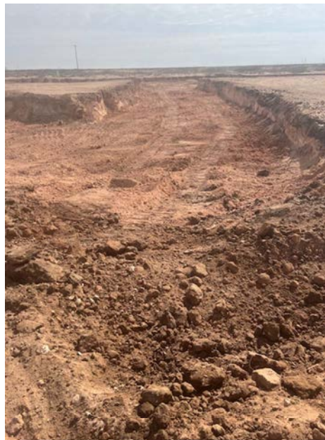
Photograph 4 Date: Feb-2025 Description: Final excavation extent
