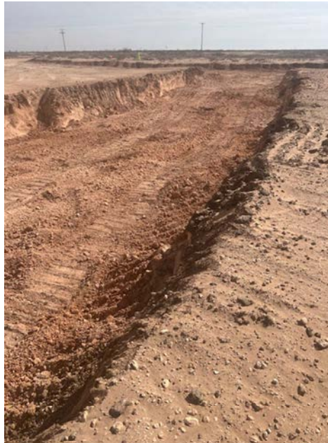
Photograph 2 Date: Feb-2025 Description: Final excavation extent
