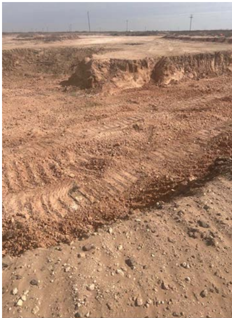
Photograph 3 Date: Feb-2025 Description: Final excavation extent
