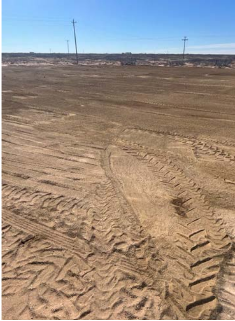
Photograph 1 Date: Feb-2025 Description: Backfilled excavation
