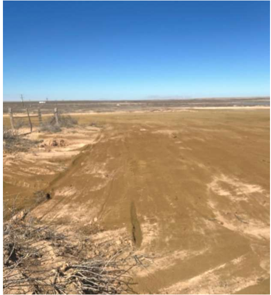
Photograph 2 Date: Feb-2025 Description: Backfilled excavation
