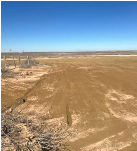
Photograph 3 Date: Feb-2025 Description: Backfilled excavation
