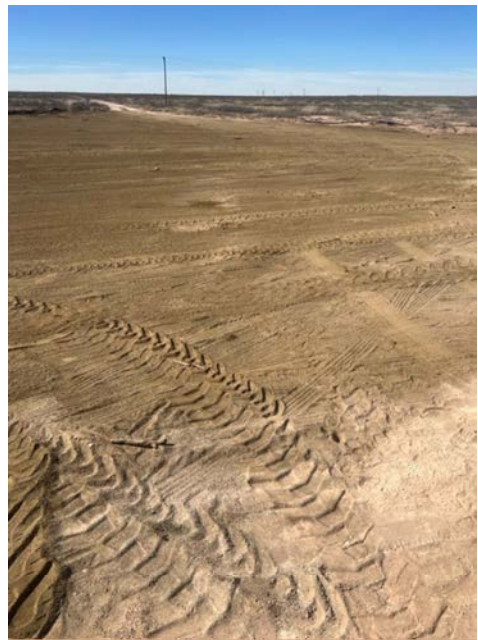
Photograph 4 Date: Feb-2025 Description: Backfilled excavation
