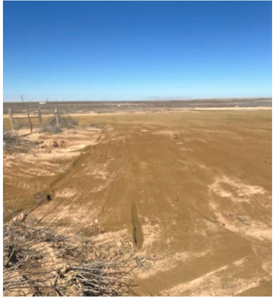
Photograph 2 Date: Feb-2025 Description: Backfilled excavation
