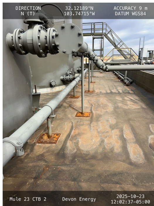
Photo 12 View of east side of containment towards north.
