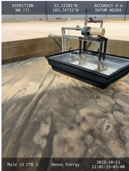
Photo 5 View of northwest corner of containment.
