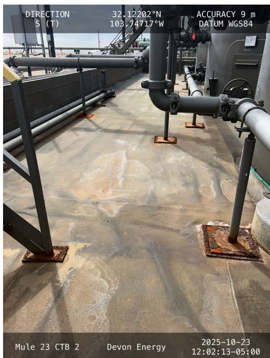
Photo 11 View of east side secondary containment towards south.
