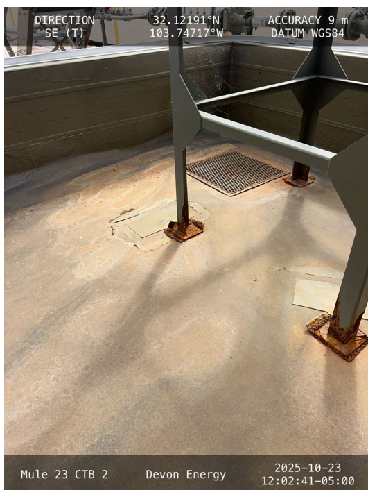
Photo 13 View of southeast corner of secondary containment.
