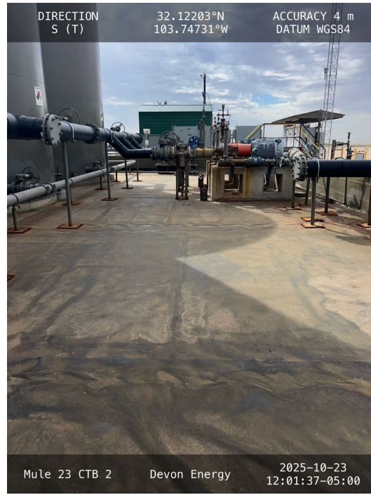
Photo 6 View of west side containment facing south.
