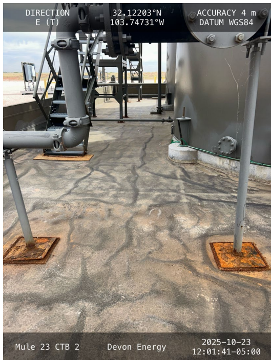
Photo 7 View of north side of containment towards east.
