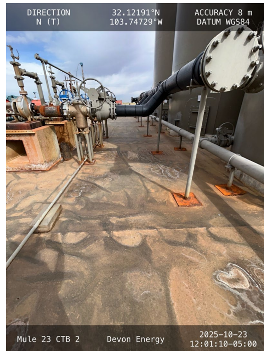
Photo 4 View of west side of containment towards north.
