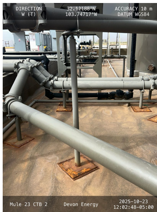
Photo 14 View of south side of containment towards west.
