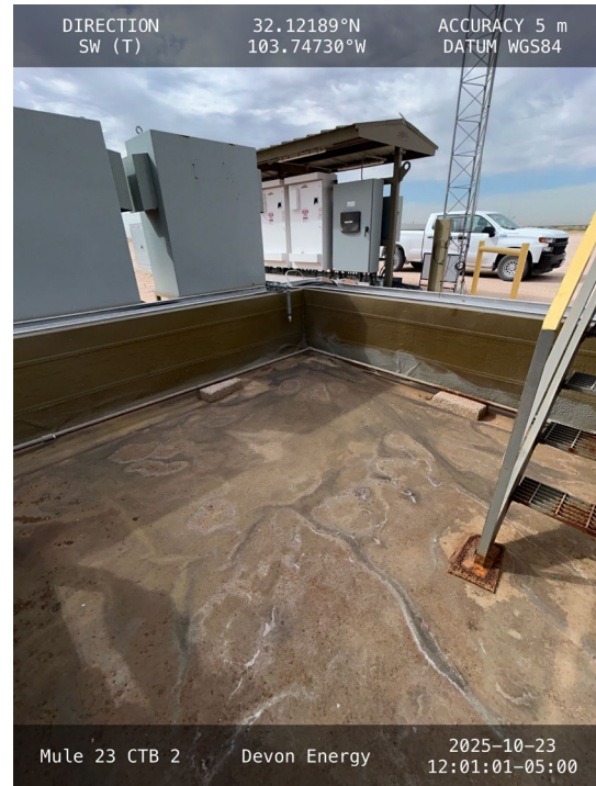
Photo 2 View of southwest corner of containment.
