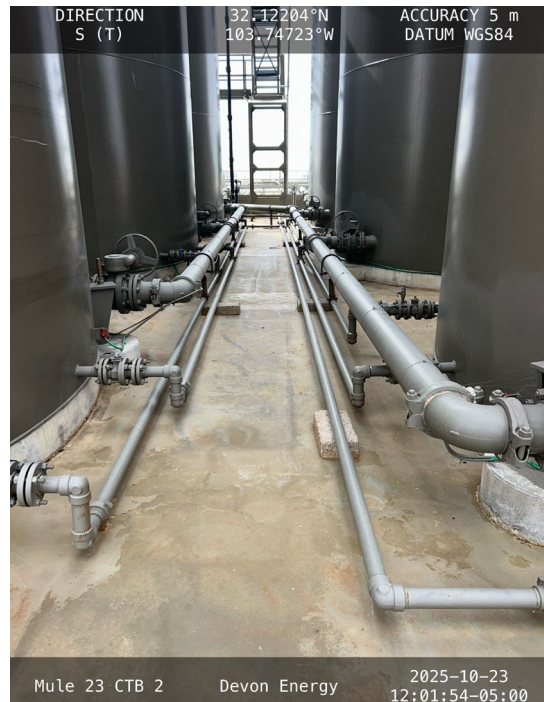
Photo 8 View of central portion of containment towards south.
