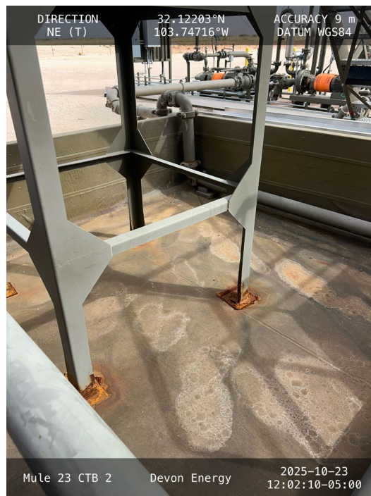
Photo 10 View of northeast corner of containment.
