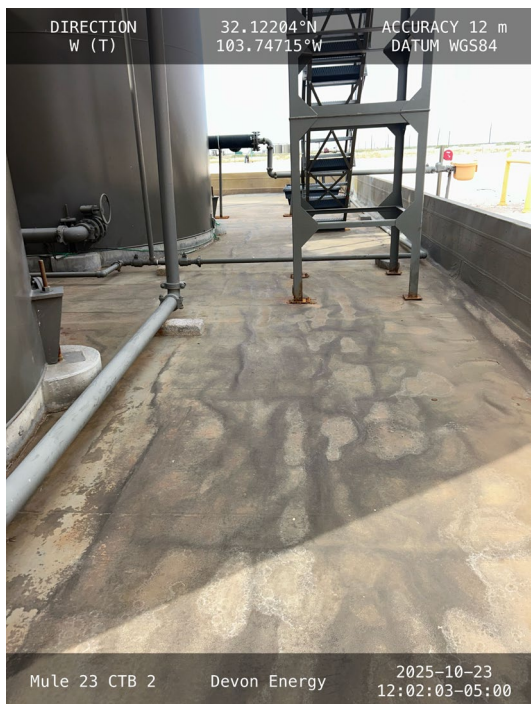
Photo 9 View of north side containment towards west.
