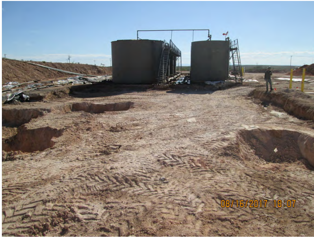
Final Excavation Area Viewing West, August 16, 2017
