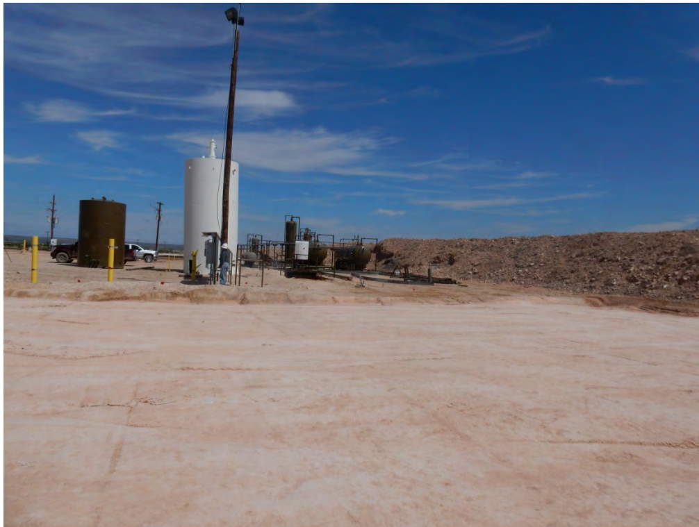
Final Backfill Viewing North, August 23, 2017
