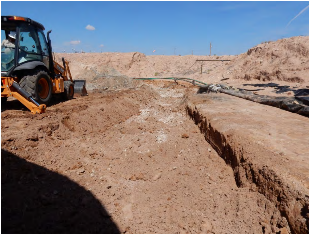
Soil Excavation along South Side of Spill Area Viewing East, August 10, 2017
