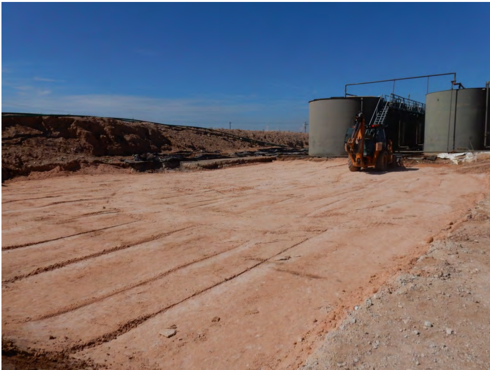
Backfill of Excavation Viewing Southwest, August 22, 2017
