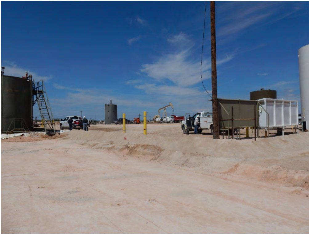
New Firewall Viewing Northwest, August 23, 2017
