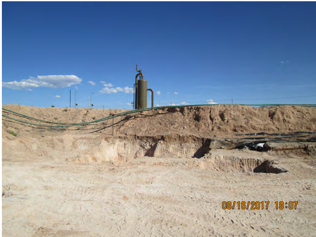
Final Excavation Area Viewing South, August 16, 2017
