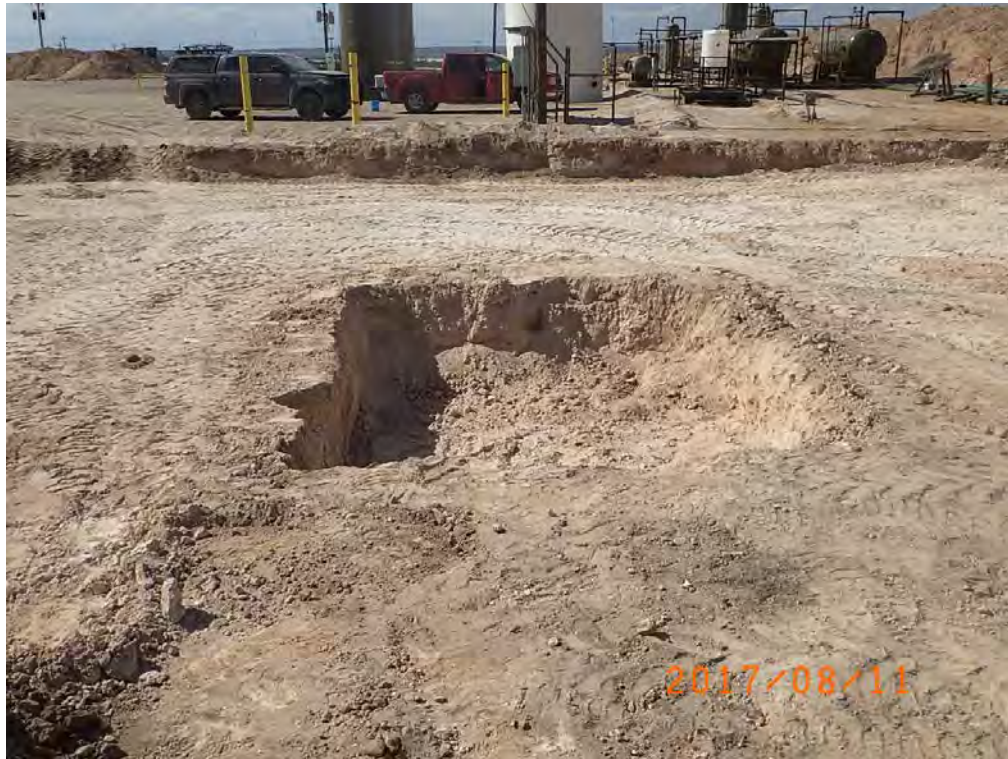
Soil Excavation at S-15 Viewing North, August 11, 2017
