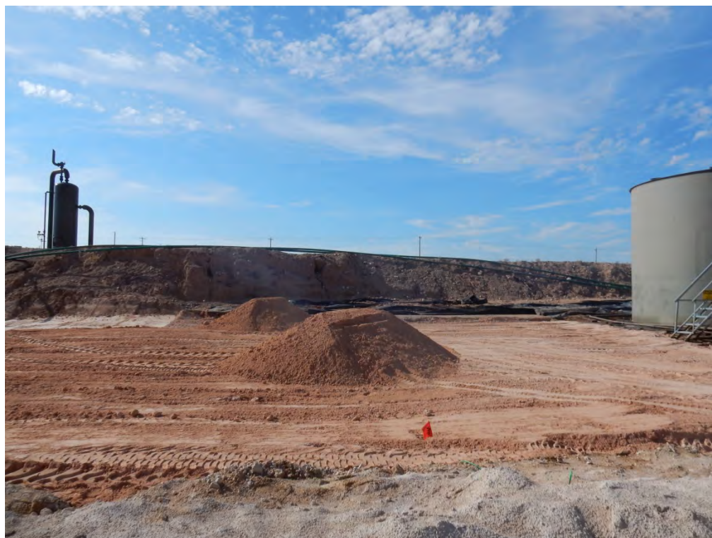
Backfill of Excavation Viewing South, August 23, 2017
