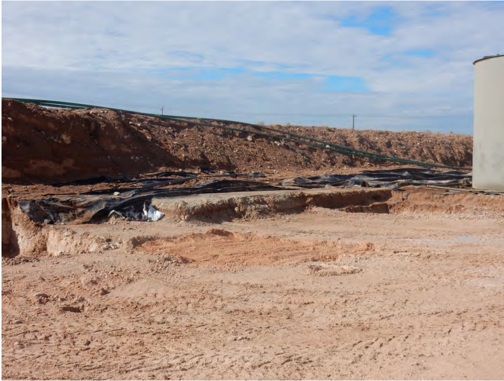
Backfill of Excavation Viewing Southwest, August 21, 2017
