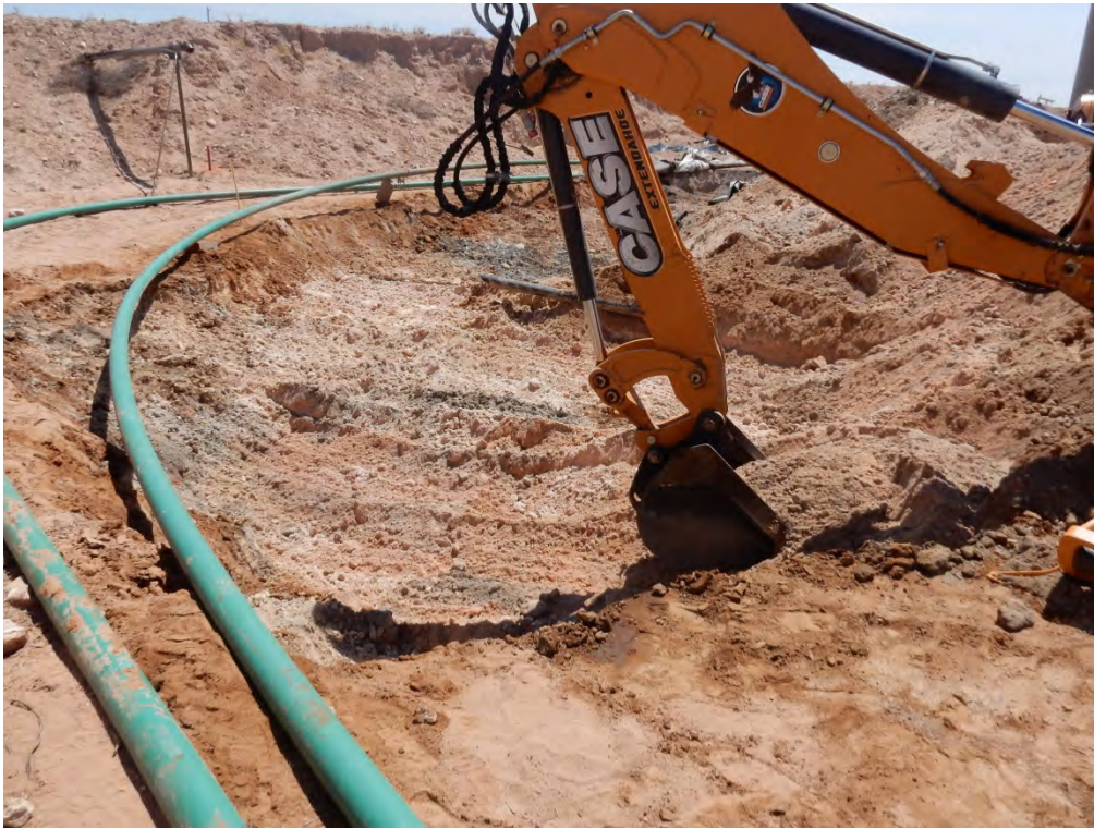
Soil Excavation near DP-7 Viewing Southwest, August 10, 2017
