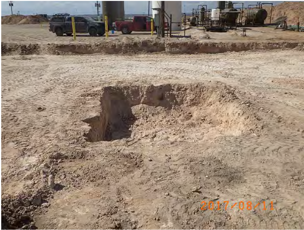
Soil Excavation at S-15 Viewing North, August 11, 2017
