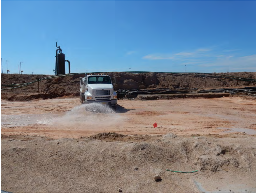
Water Packing of Excavation Viewing South, August 22, 2017
