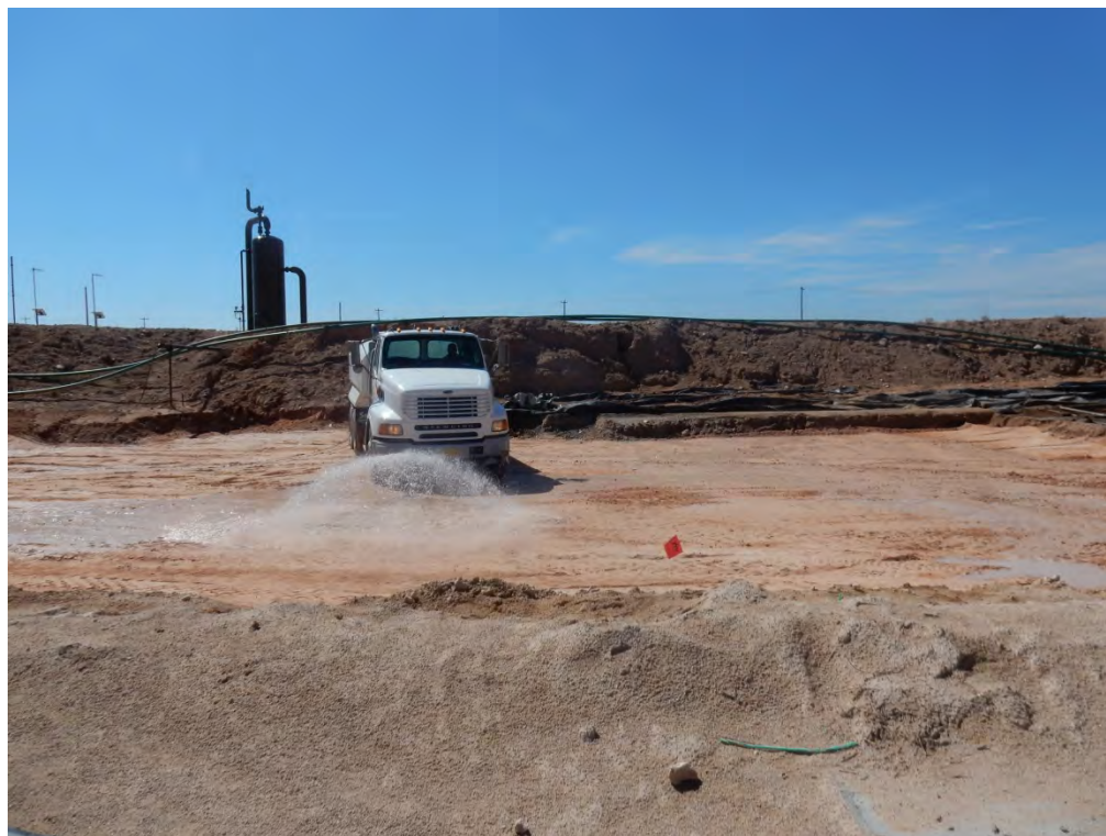
Water Packing of Excavation Viewing South, August 22, 2017
