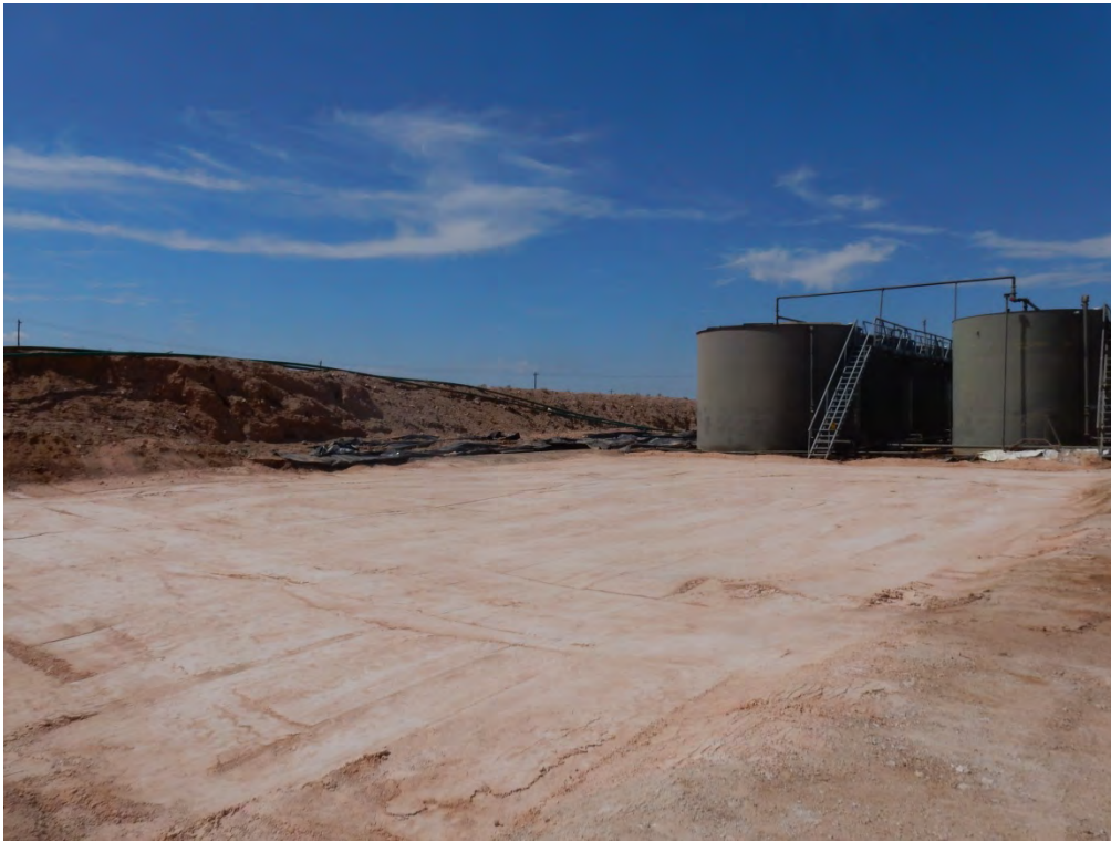
Final Backfill Viewing Southwest, August 23, 2017
