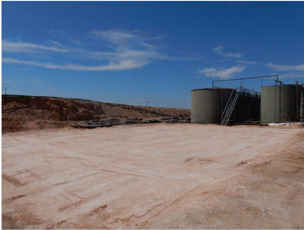
Final Backfill Viewing Southwest, August 23, 2017
