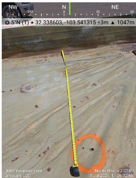
Photograph 11 Date: 7/18/2025 Description: BH02 hole in liner View: North
