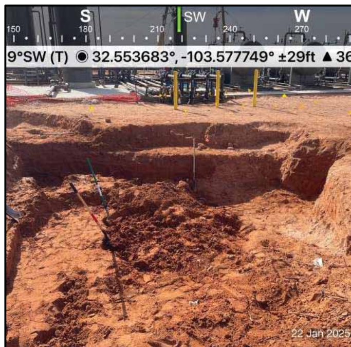
Photo 9. View of sub-areas CS-03 and CS-04 after remediation activities were performed and prior to backfilling (restoration) activities.
