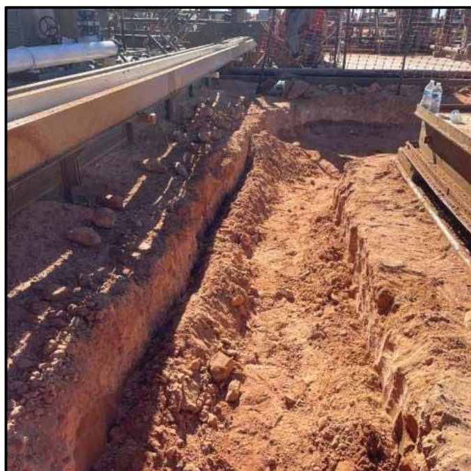
Photo 10. View of sub-areas CS-01 and CS-02 after remediation activities were performed and prior to backfilling (restoration) activities.
