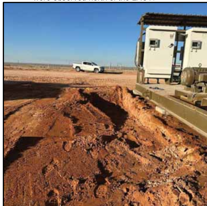
Photo 4. Excavating the extent of CS-06 during initial remediation activities. The excavation by backhoe was limited to a depth of 1.0 ft due to subsurface utilities.
