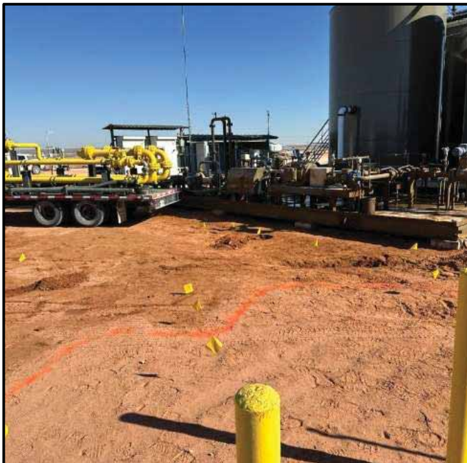
Photo 7. Orange spray paint used to demarcate the lateral extents (the perimeter) of impacted soil at the ground surface with an additional 1.0-ft capture zone.
