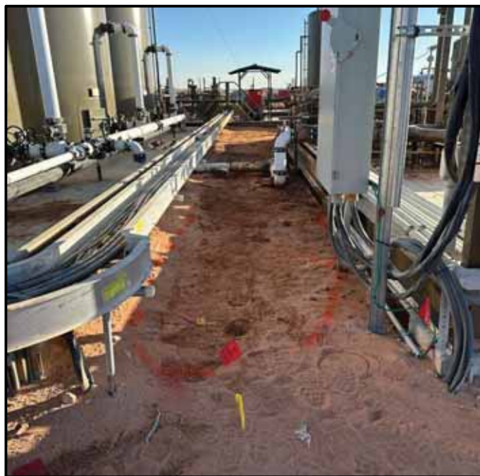
Photo 9. Collecting confirmation samples at the extent of CS-01 during initial remediation activities. No excavation was initially done at CS-01 due to the backhoe not being able to access the area.
