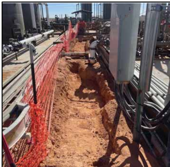
Photo 11. Excavation to a depth of 1.5 ft by hand and hydrovac methods at CS-01 until PID readings for the remaining soil indicated no or only minimal organic vapors were present.
