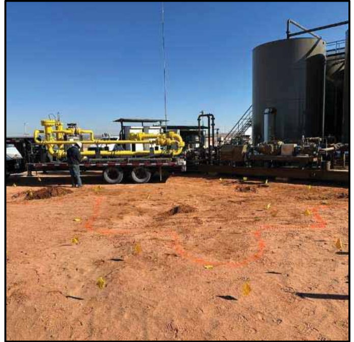
Photo 6. Orange spray paint used to demarcate the lateral extents (the perimeter) of impacted soil at the ground surface with an additional 1.0-ft capture zone.
