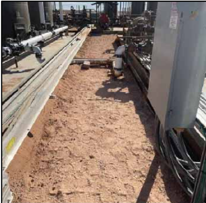
Photo 15. View of sub-area CS-01 at the conclusion of backfilling, watering, and compaction activities.
