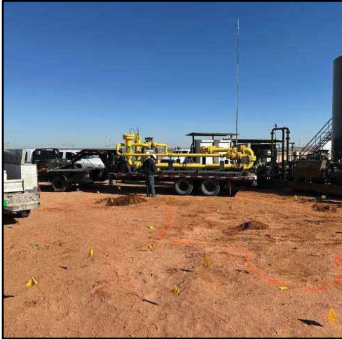
Photo 5. Orange spray paint used to demarcate the lateral extents (the perimeter) of impacted soil at the ground surface with an additional 1.0-ft capture zone.
