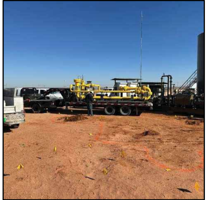
Photo 2. The visual extent of surface impacts outlined with orange spray paint at sub-areas CS-04 and CS-05; prior to remediation activities.
