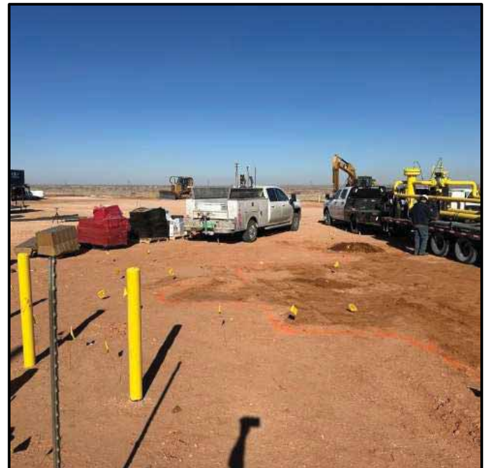
Photo 8. Orange spray paint used to demarcate the lateral extents (the perimeter) of impacted soil at the ground surface with an additional 1.0-ft capture zone.
