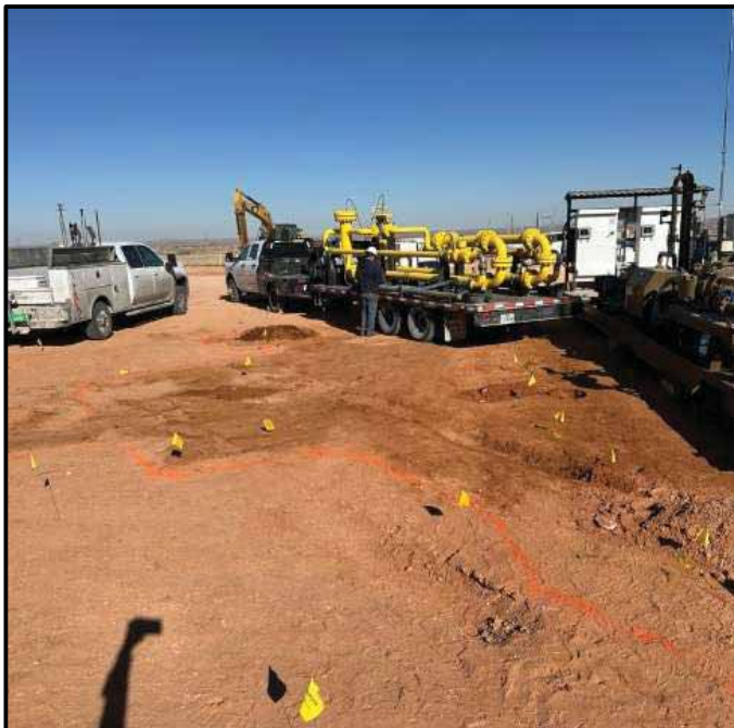
Photo 3. The visual extent of surface impacts outlined with orange spray paint at sub-areas CS-05 and CS-06; prior to remediation activities.
