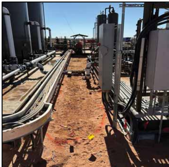
Photo 3. The northeast side (CS-01) of the LACT, after release and prior to remediation. Yellow pin flags and orange spray paint outlining the extent of the release are visible. No wet or discolored areas of soil were observed north of the LACT.
