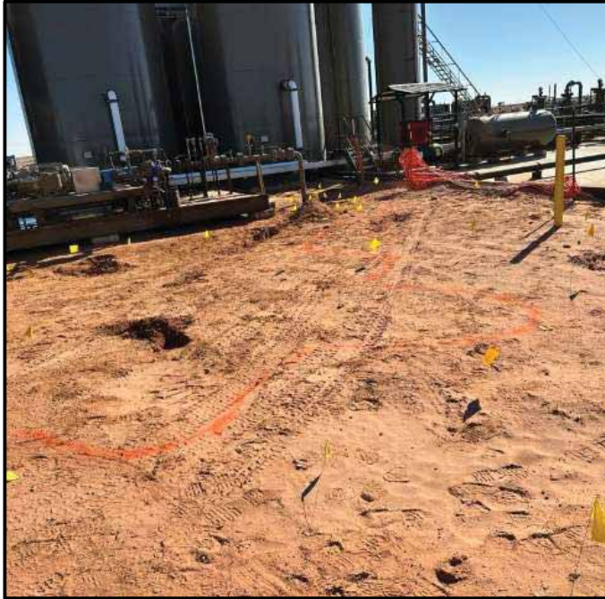
Photo 1. The visual extent of surface impacts outlined with orange spray paint at sub-areas CS-03 and CS-04; prior to remediation activities.
