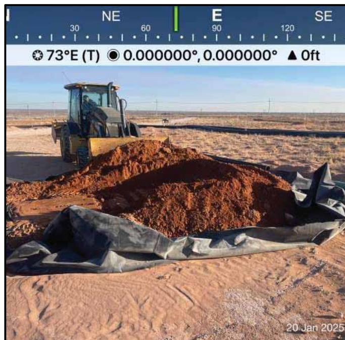
Photo 7. The temporary waste staging area where waste soil was deposited as remediation activities were being performed.
