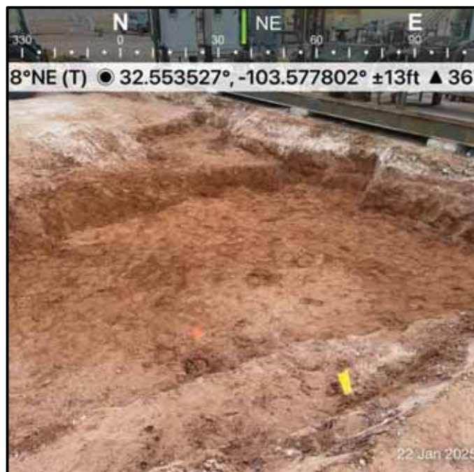
Photo 10. Excavation to a depth of 1.25 ft by hand and hydrovac methods at CS-06 until PID readings for the remaining soil indicated no or only minimal organic vapors were present.
