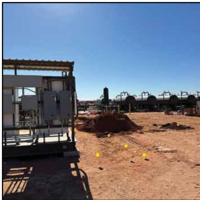
Photo 2. The northwest side (CS-06) of the LACT, after release and shortly after excavation commenced. Yellow pin flags and orange spray paint outlining the extent of the release are visible. No wet or discolored areas of soil were observed north of the LACT.
