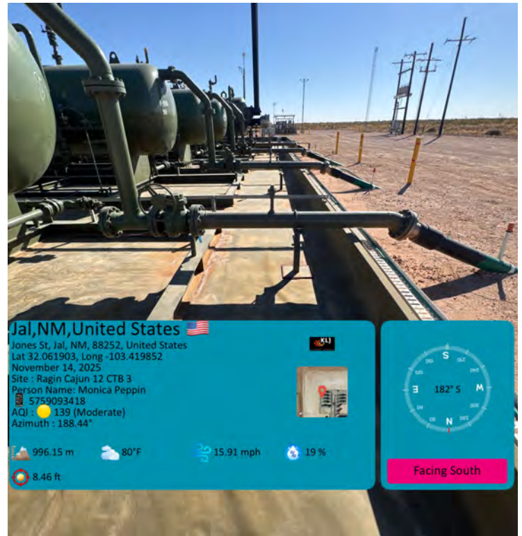
West wall of liner.
