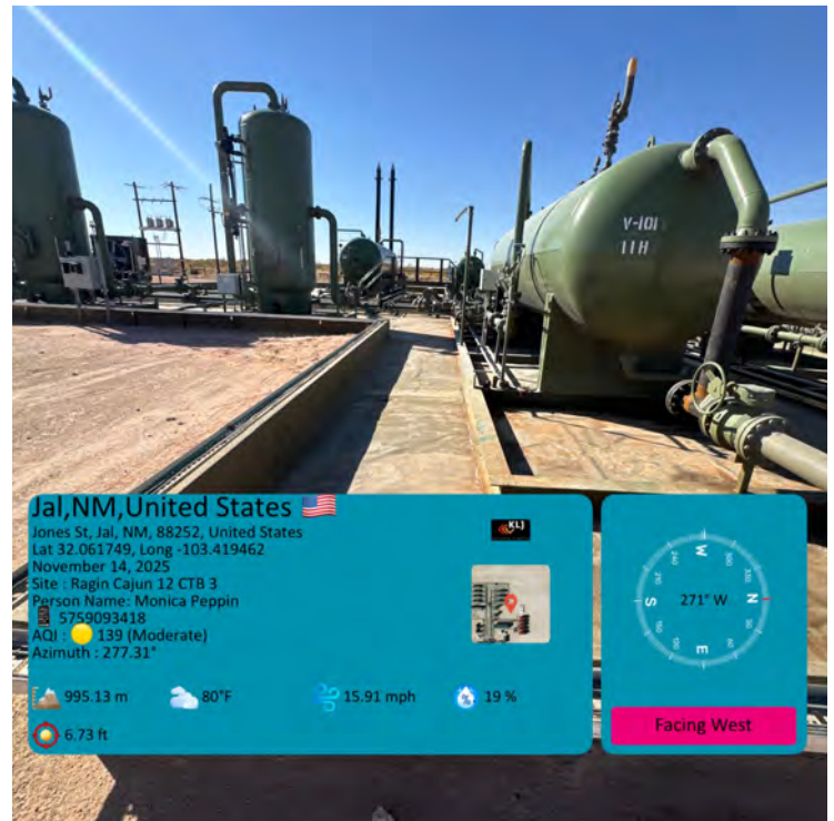
southeast corner of liner.
