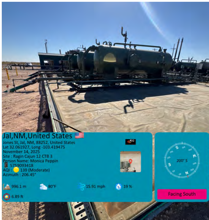
Northeast area of containment.
