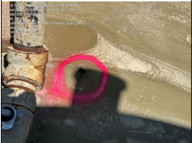
Photograph: 8 Date: 8/26/2025 Description: Identified hole in liner near BH01 View: Direct
