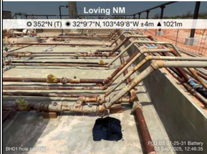
Photograph: 10 Date: 9/3/2025 Description: Liner patching activities View: North
