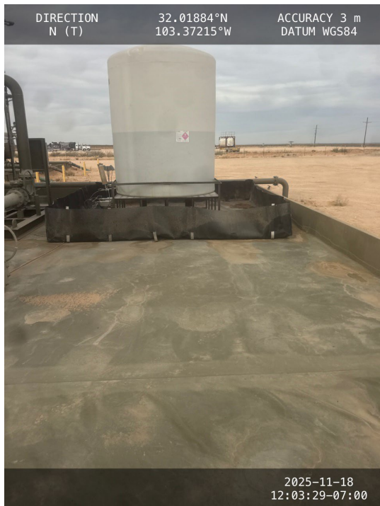
Photo 3 View of containment facing north.
