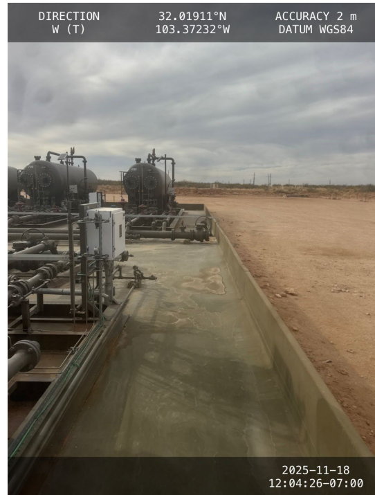
Photo 2 View of containment facing west.
