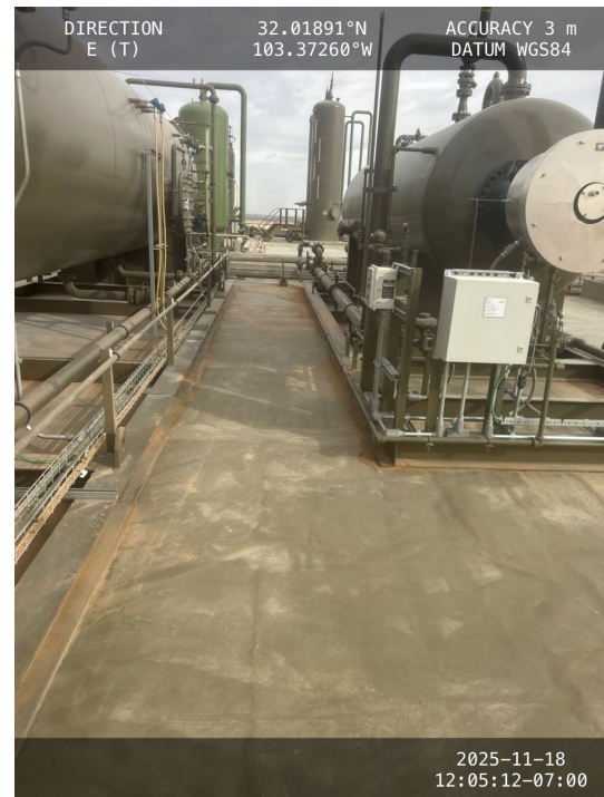
Photo 4 View of containment facing east.
