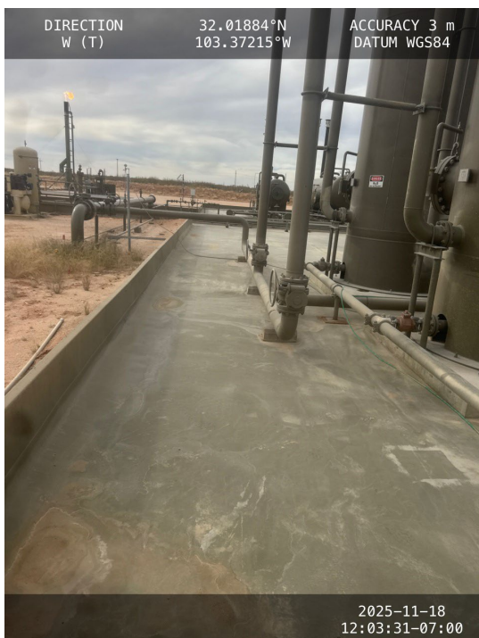
Photo 7 View of containment facing west.
