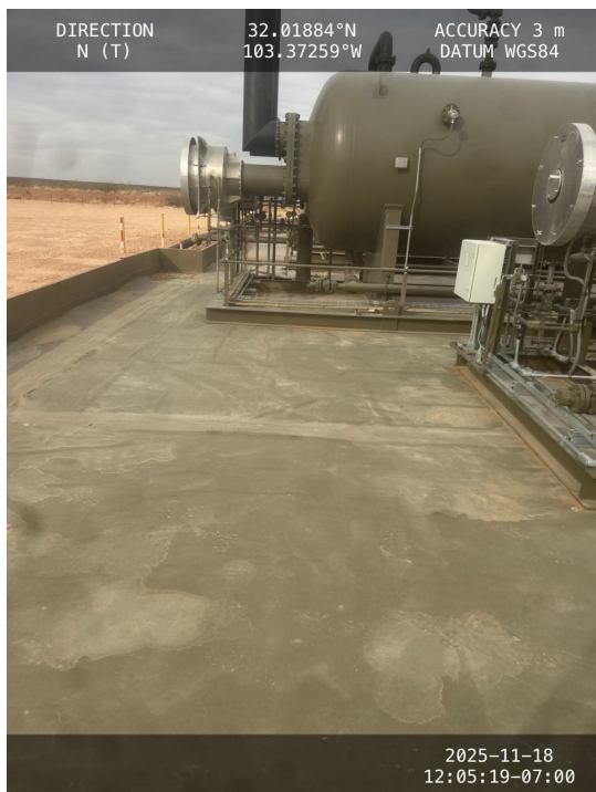
Photo 5 View of containment facing north.
