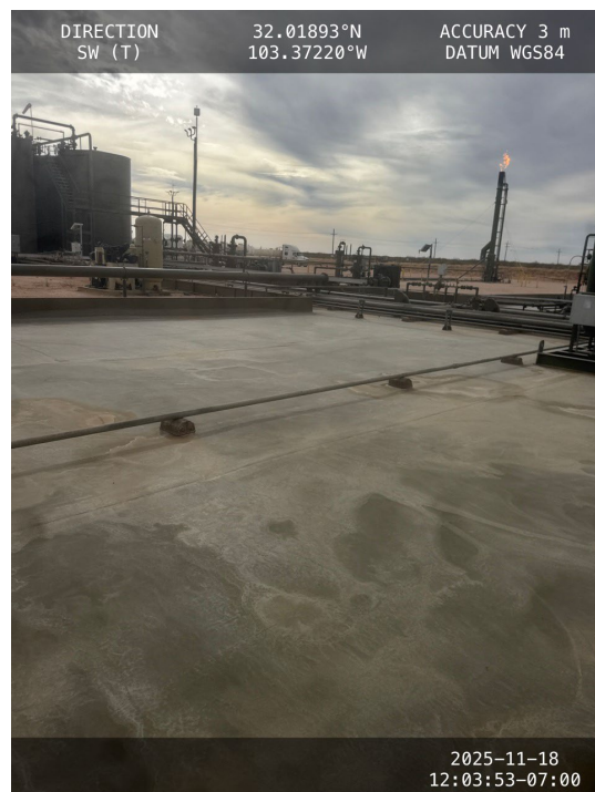
Photo 8 View of containment facing southwest.
