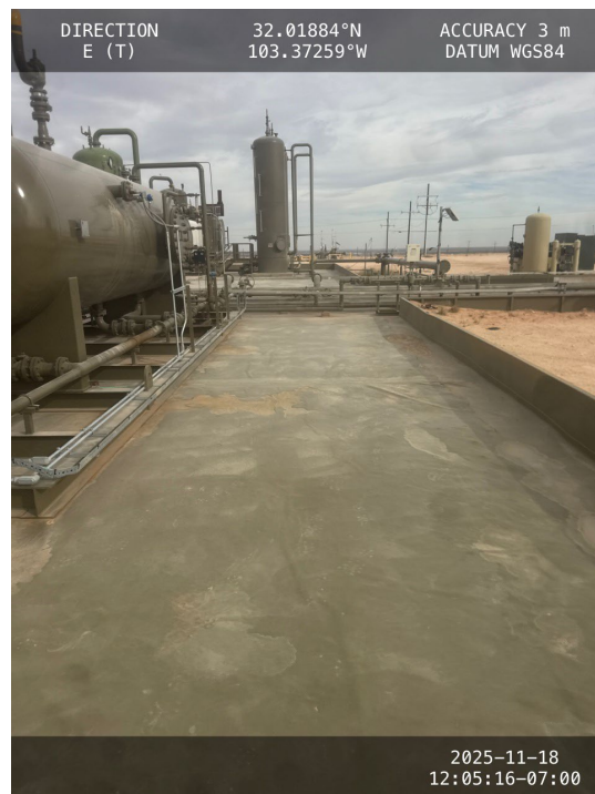
Photo 6 View of containment facing east.
