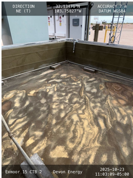
Photo 13 View of northeast corner of secondary containment.
