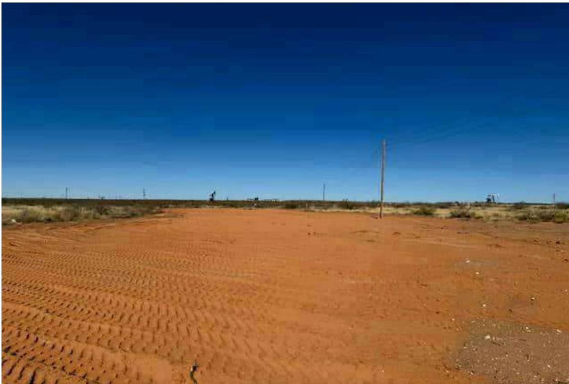
Photo 3 View after backfilling looking north toward release point.
