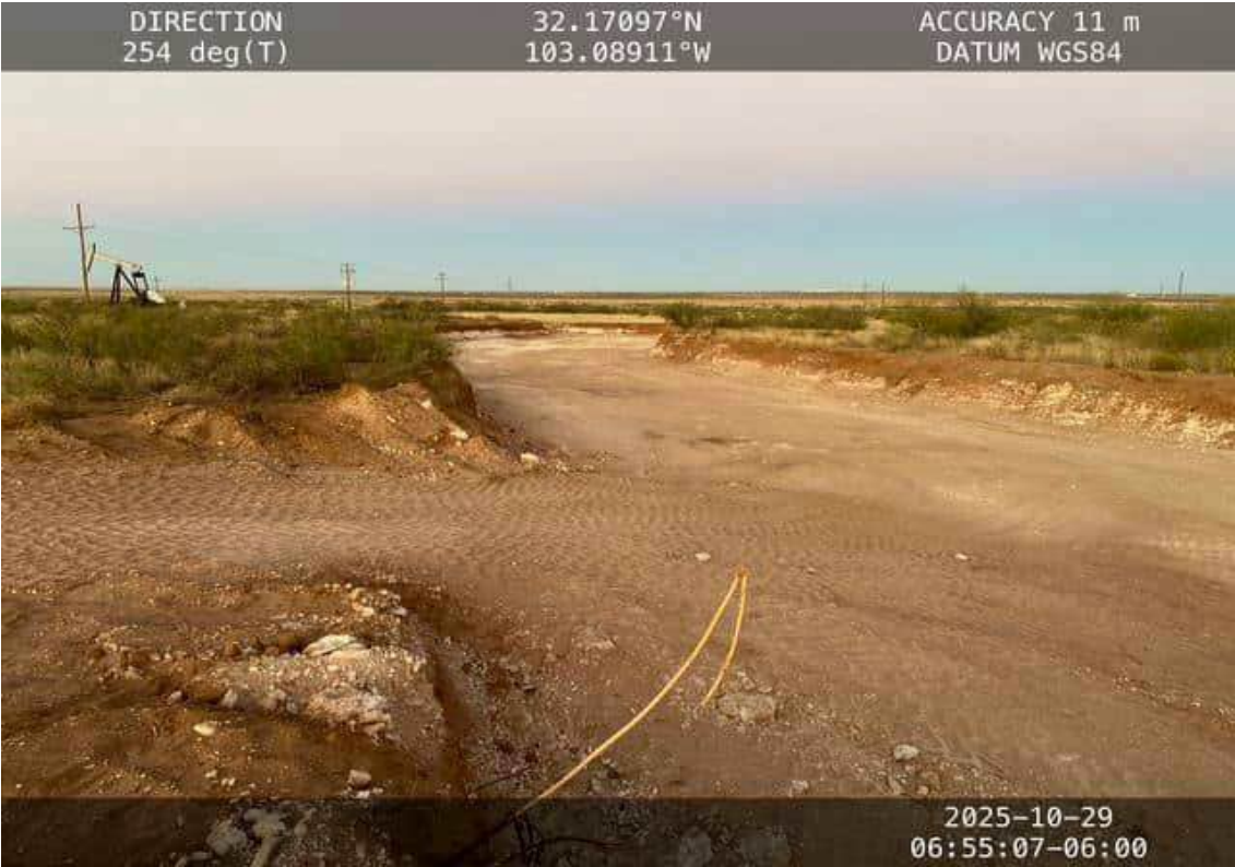
Photo 5 View of excavation looking west from southern turn.
