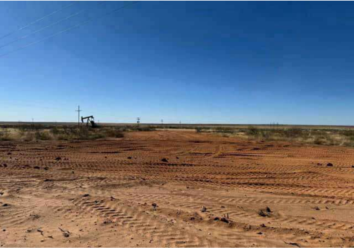
Photo 6 View after backfilling looking west from southern turn.
