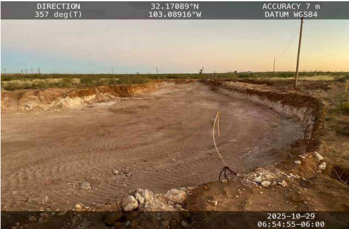
Photo 2 View of Excavation looking north toward release point.
