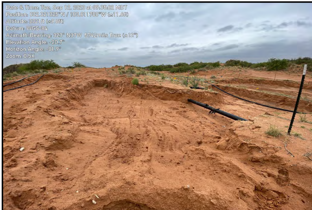
View of initial excavation activities, facing northwest.
