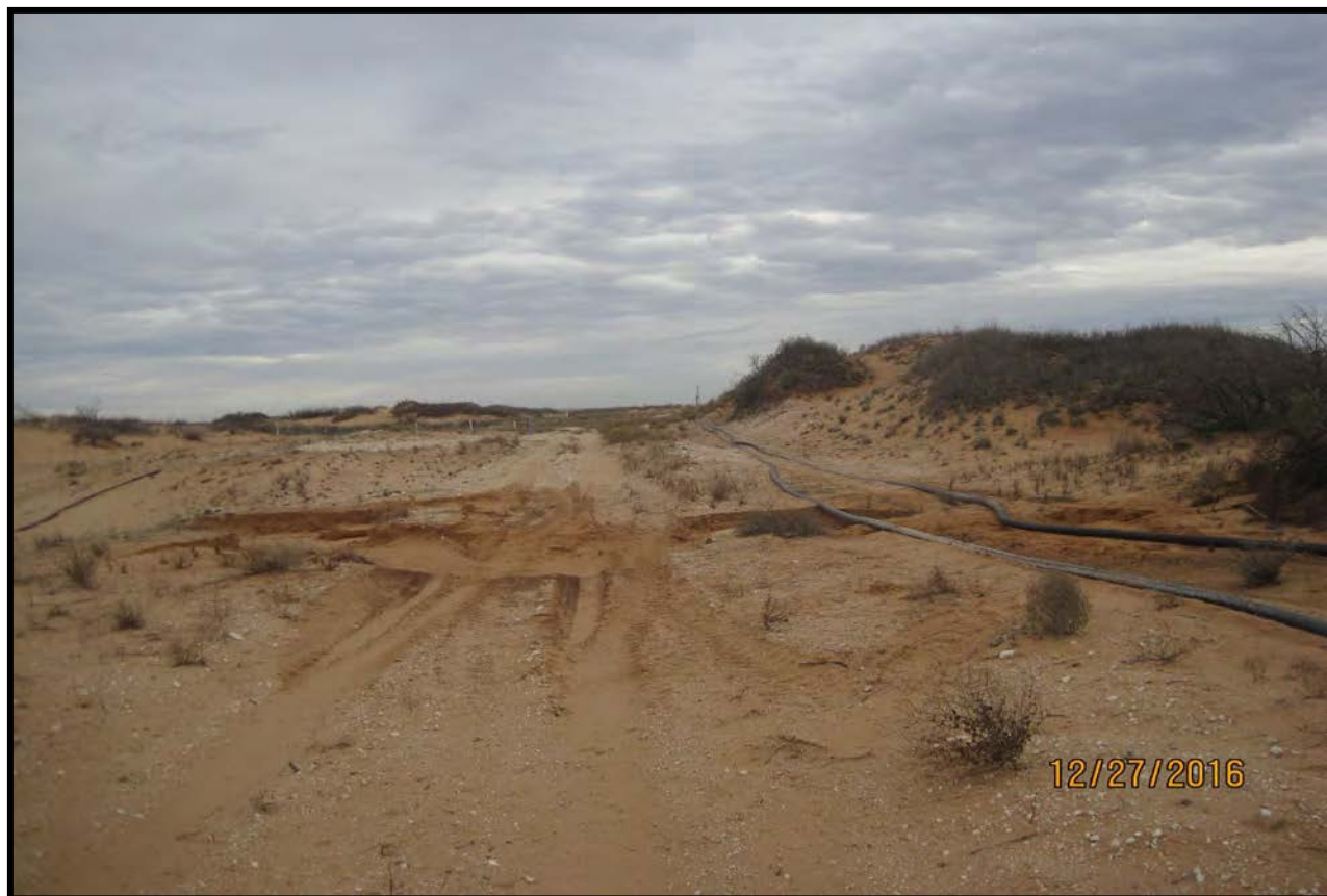
View of initial spill, facing southeast.
