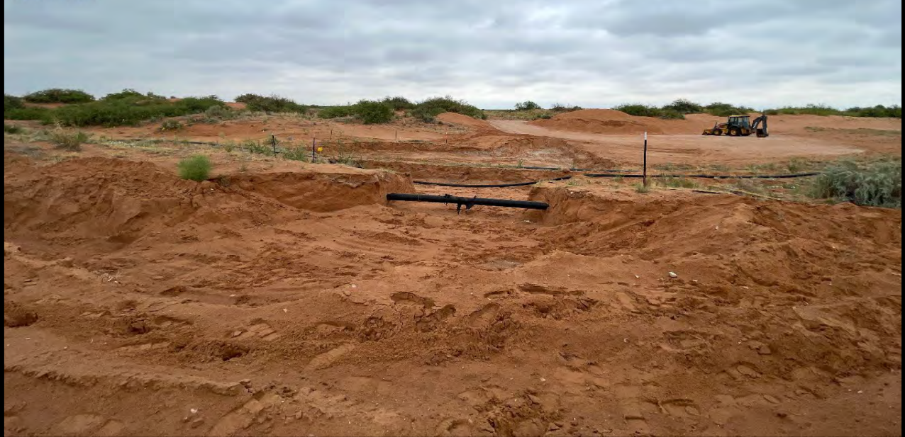
View of initial excavation activities, facing northeast.
