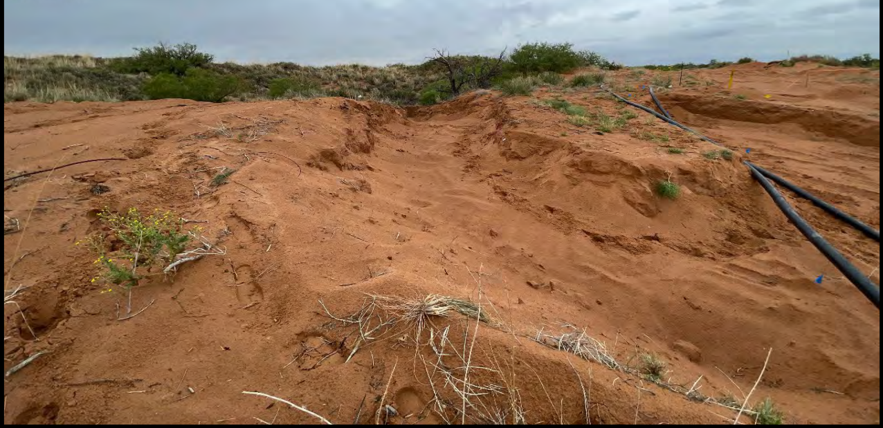
View of initial excavation activities, facing northwest.
