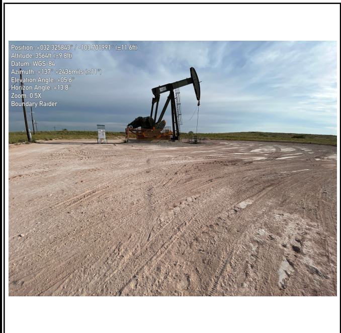
Photograph 7 Date: 09/17/2025 Description: View of completed restoration activities.
