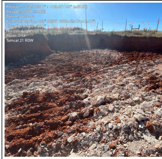
Photograph 2 Date: 11/03/2025 Description: Southwestern view of northern excavation.
