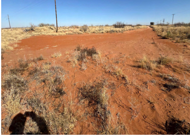
Photograph 5 Date: 12/16/2025 Description: Northeastern view of the backfilled northern excavation.
