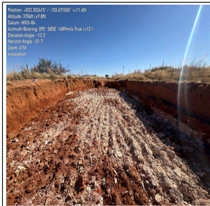
Photograph 4 Date: 11/04/2025 Description: Southeastern view of southern excavation.
