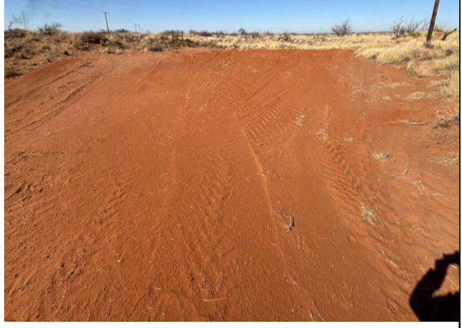
Photograph 6 Date: 12/16/2025 Description: Northwestern view of the backfilled southern excavation.
