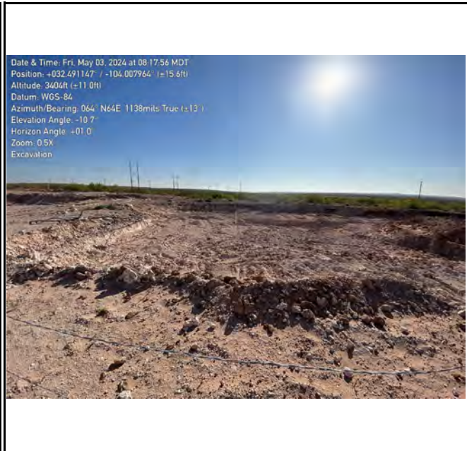
Photograph 4 Date :5/3/2024 Description: Southern excavation View: Northeast
