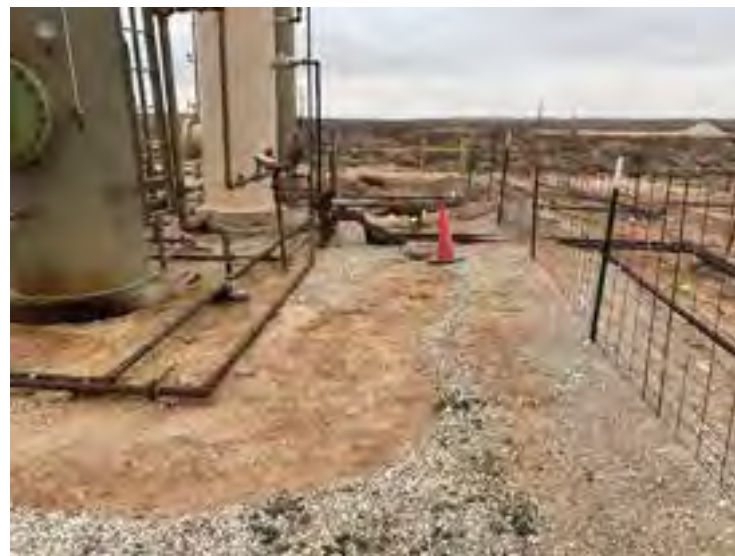
Photograph 4: View of equipment after hand shoveling activities.
