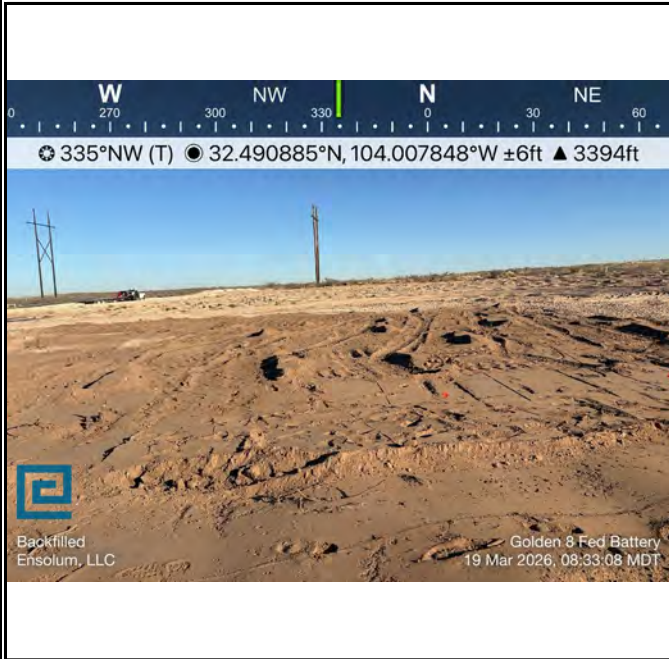
Photograph 1 Date :3/19/2026 Description: Backfilled excavation area View: Northwest
