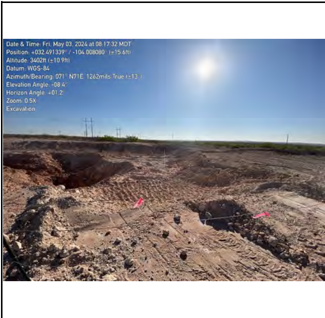
Photograph 3 Date :5/3/2024 Description: South portion of northern excavation View: Northeast
