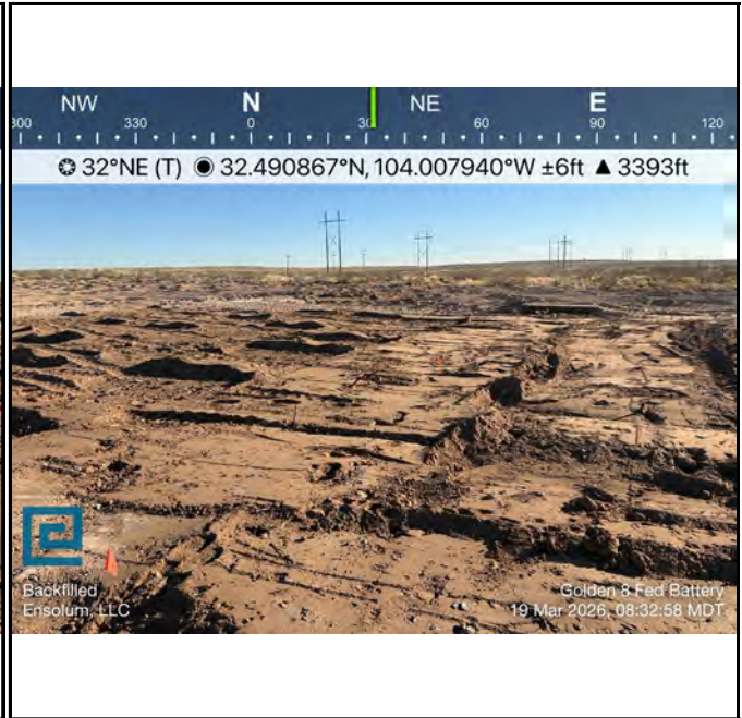
Photograph 2 Date :3/19/2026 Description: Backfilled excavation area View: Northeast
