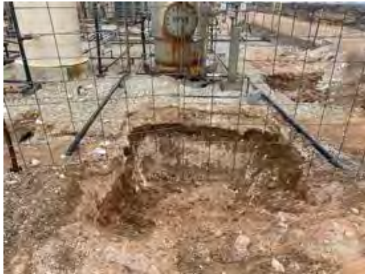
Photograph 7: View north of southern excavation activities.
