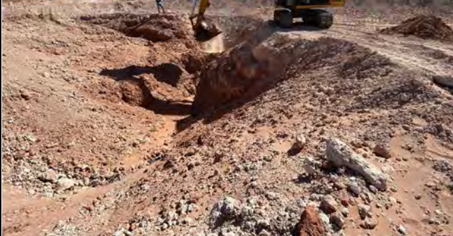
Photograph : 6 Date :6/3/2024 Description: Northern excavation View: Northeast
