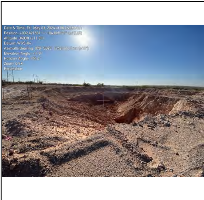
Photograph 1 Date :5/3/2024 Description: North portion of northern excavation View: East
