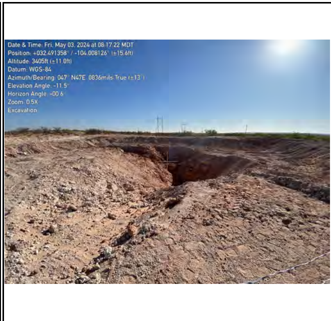
Photograph 2 Date :5/3/2024 Description: Northern excavation View: Northeast
