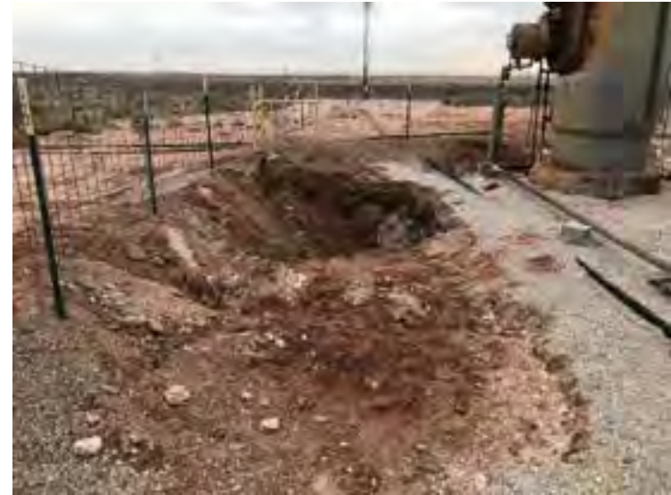
Photograph 6: Southern view of eastern excavation activities.
