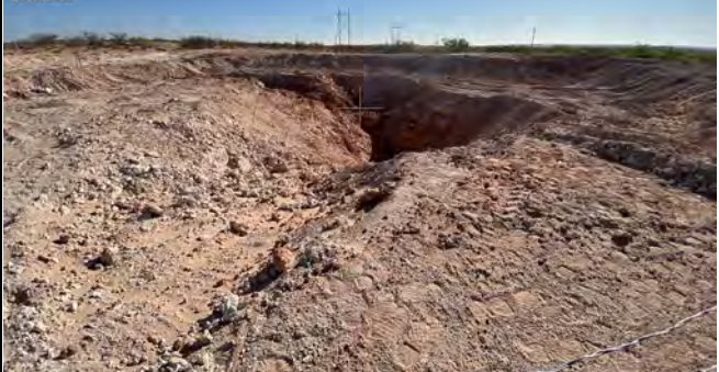
Photograph 2 Date :5/3/2024 Description: Northern excavation View: Northeast
