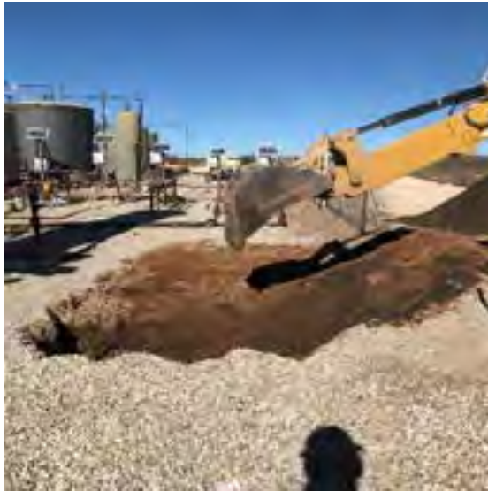
Photograph 5: Northern view of eastern excavation activities.
