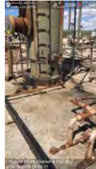
Photograph 2: Northern view of surficial staining within release extent.
