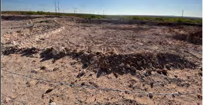
Photograph 4 Date :5/3/2024 Description: Southern excavation View: Northeast
