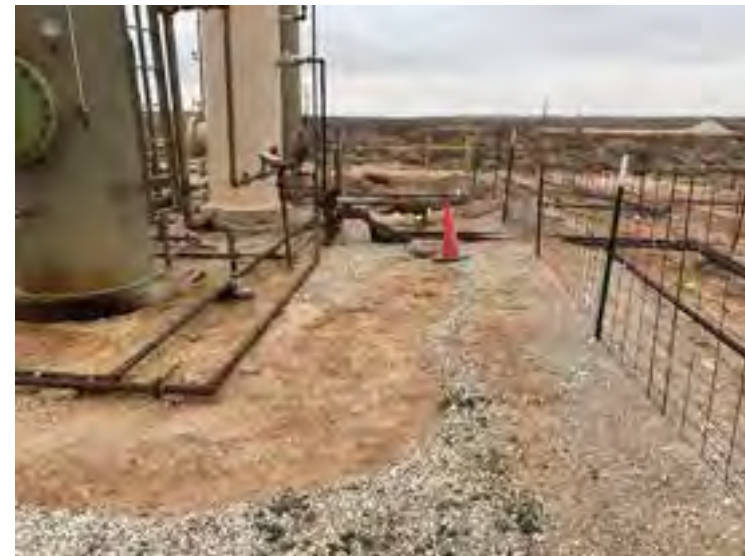
Photograph 4: View of equipment after hand shoveling activities.
