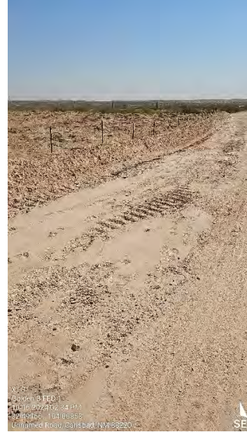
Photograph : 12 Date :10/16/2024 Description: Bermed and fenced well pad View: Southeast
