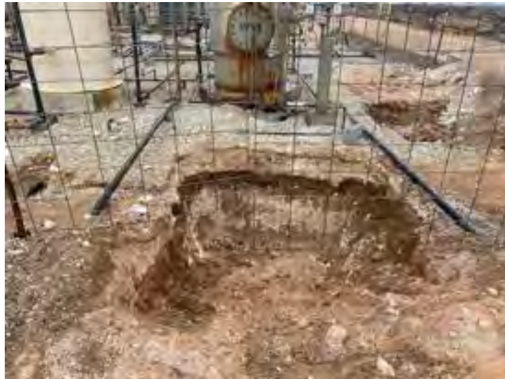
Photograph 7: View north of southern excavation activities.
