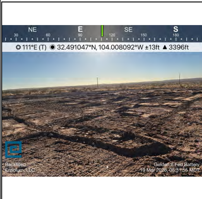
Photograph 3 Date :3/19/2026 Description: Backfilled excavation area View: East
