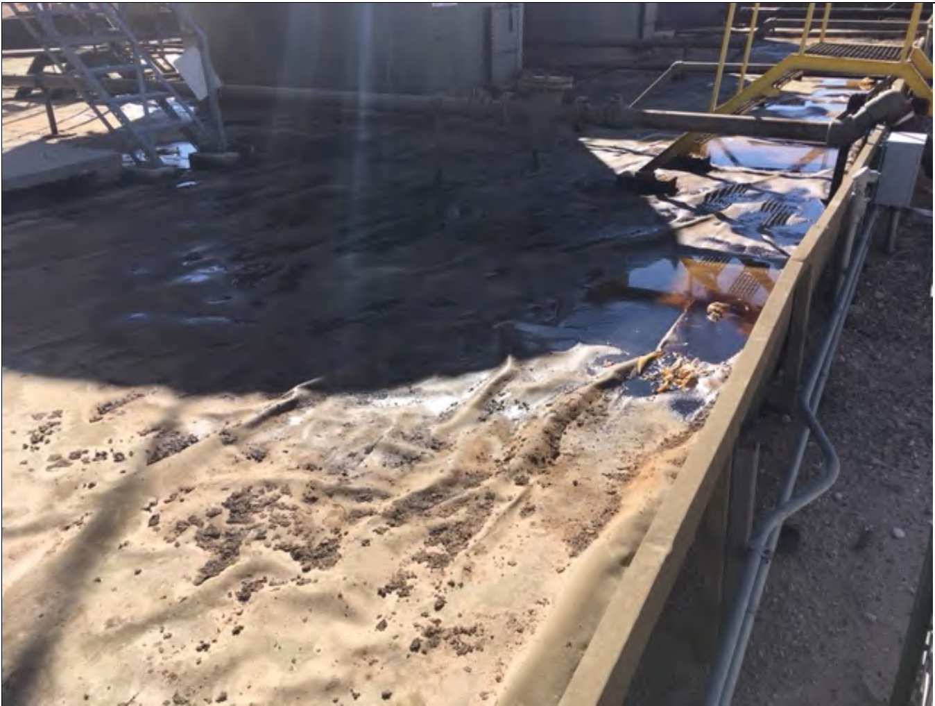
View of lined tank battery containment and liner hole during soil sampling activities.
