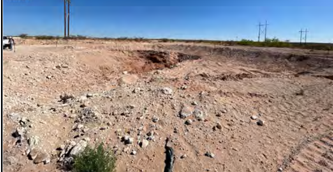
Photograph : 5 Date :6/3/2024 Description: Northern excavation View: North
