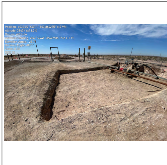
Photograph 10 Date: 02/26/2026 Description: Southwestern view of excavation confirmation activities.
