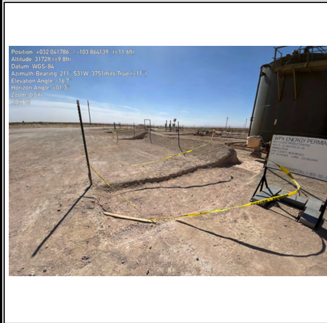
Photograph 9 Date: 02/20/2026 Description: Southwestern view of excavation activities.
