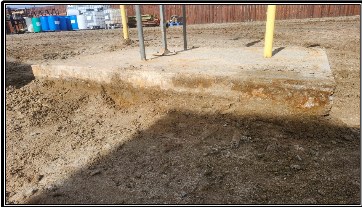
Photo 2: Excavated soil around concrete pad
