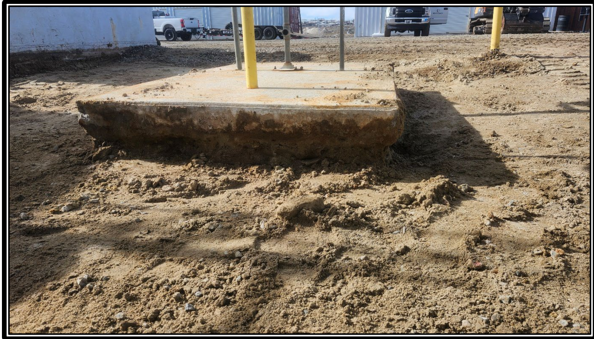
Photo 3: Excavated area around concrete
