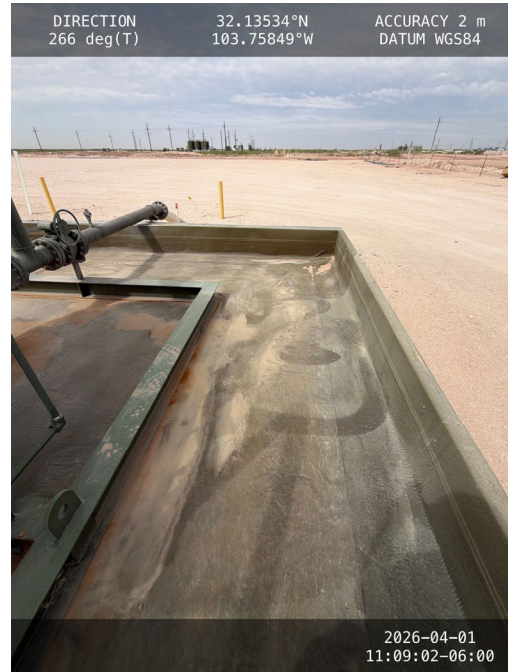
Photo 2 Photo of southwest corner of containment.
