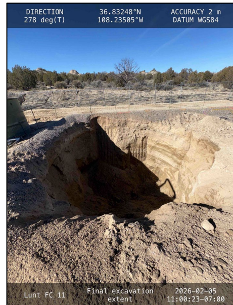
Photograph: 8 Date: 02/05/2026 Description: Final Excavation Extent View: West
