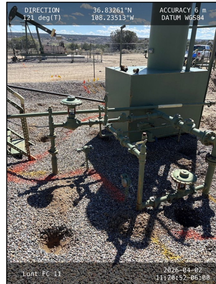
Photograph: 10 Date: 04/02/2026 Description: Composite Soil Sampling Activities View: Southeast
