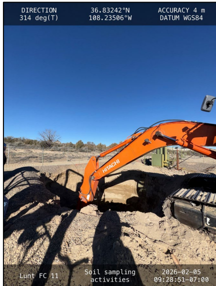
Photograph: 5 Date: 02/05/2026 Description: Composite Soil Sampling Activities View: North-West
