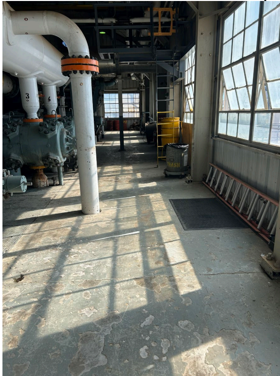
Photo 4: View of concrete floor below the compressor.
