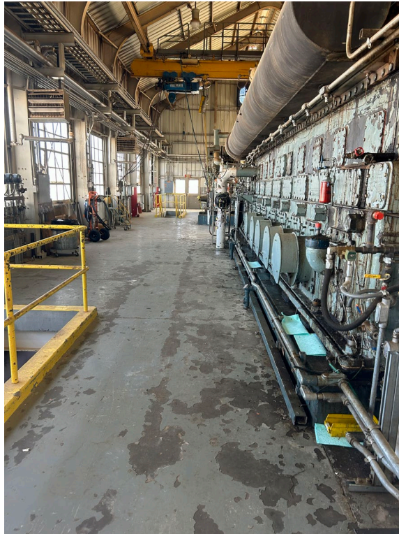
Photo 3: View of concrete floor below the compressor.
