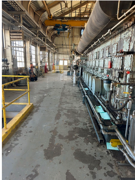
Photo 3: View of concrete floor below the compressor.
