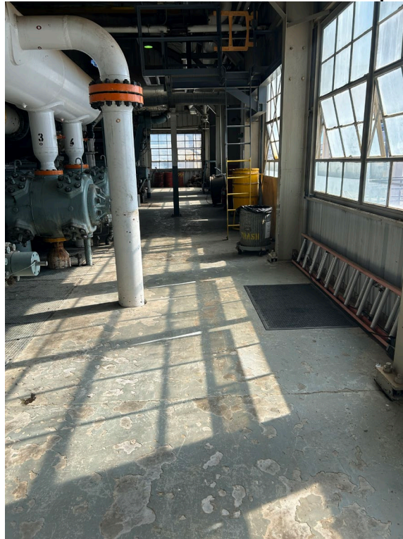
Photo 4: View of concrete floor below the compressor.
