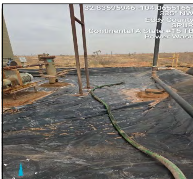
Photograph taken post powerwash facing northwest.
