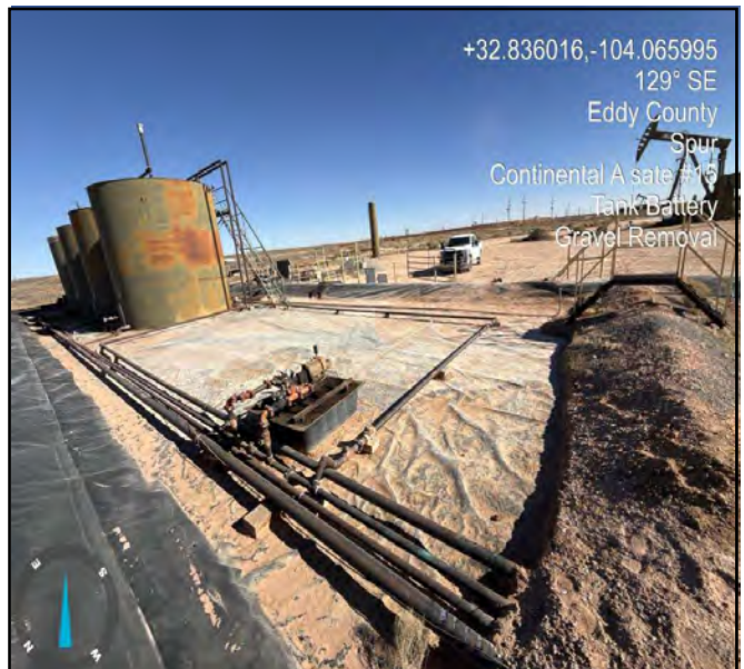
Photograph taken during the gravel removal process facing southeast.
