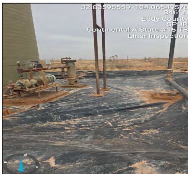
Photograph taken during liner inspection facing north.
