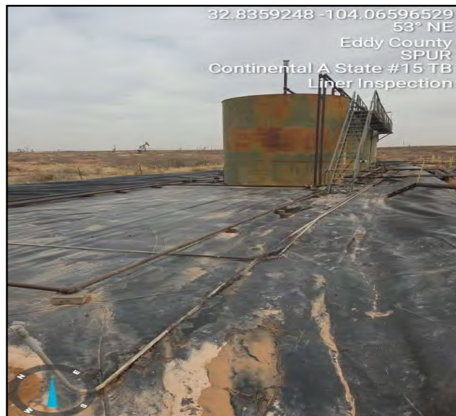
Photograph taken during liner inspection facing northeast.
