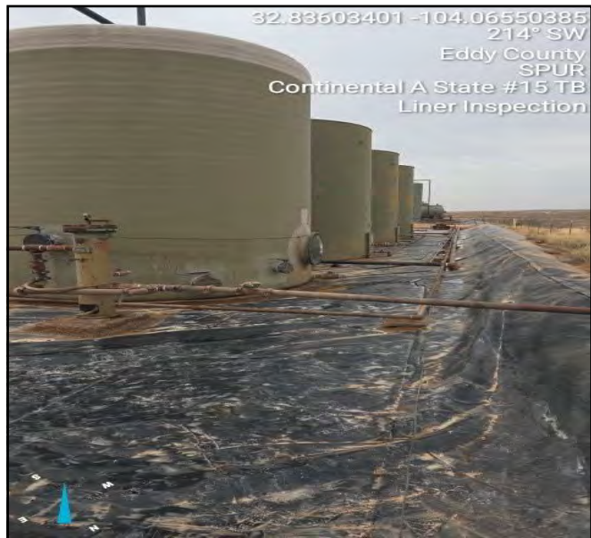
Photograph taken during liner inspection facing southwest.
