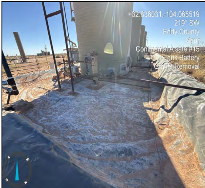
Photograph taken during the gravel removal process facing southwest.
