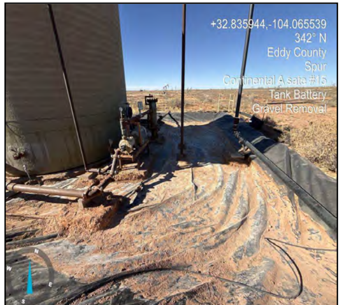
Photograph taken during the gravel removal process facing north.
