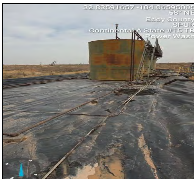
Photograph taken post powerwash facing northeast.
