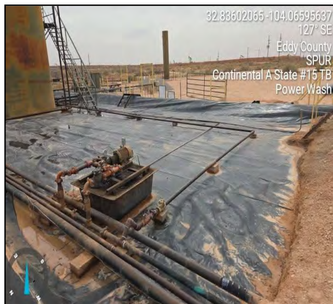
Photograph taken post powerwash facing southeast.
