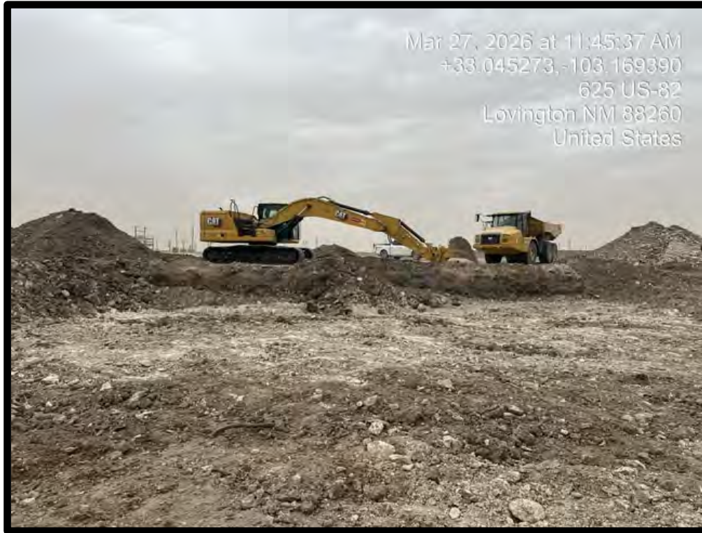
PHOTOGRAPH NO. 3 – A view of the ongoing excavation activities.
