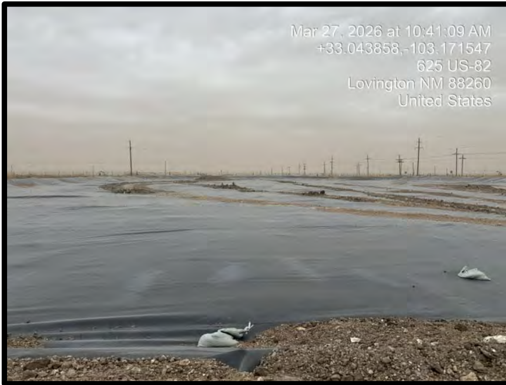
PHOTOGRAPH NO. 5 – A view of the southern treatment cell awaiting the placement of soils for treatment. The view is towards the south.
