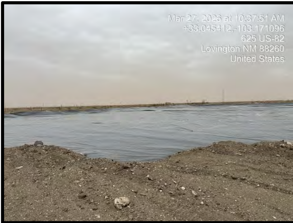
PHOTOGRAPH NO. 6 – A view of the completed Northern Treatment Cells with excavated material pending treatment. The view is towards the northwest.
