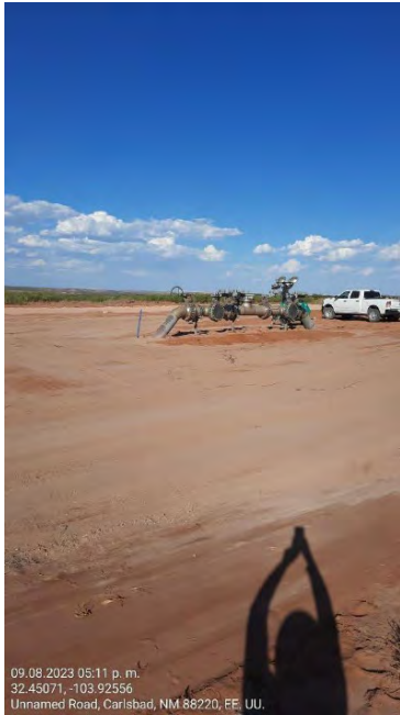
Photograph 5 Date: 09/08/2023 Description: Excavation backfilled. View: Southeast
