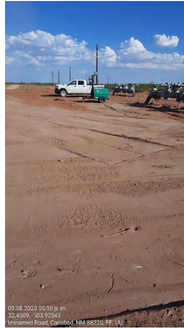
Photograph 6 Date: 09/08/2023 Description: Excavation backfilled. View: East
