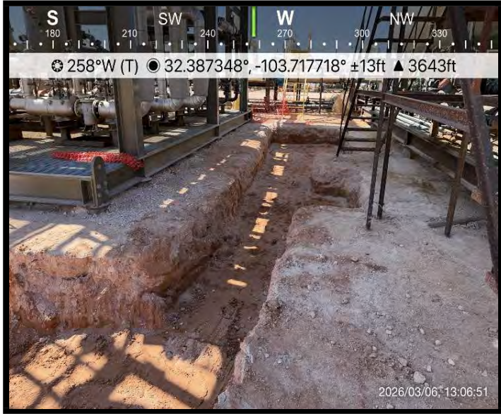
View of Excavation
