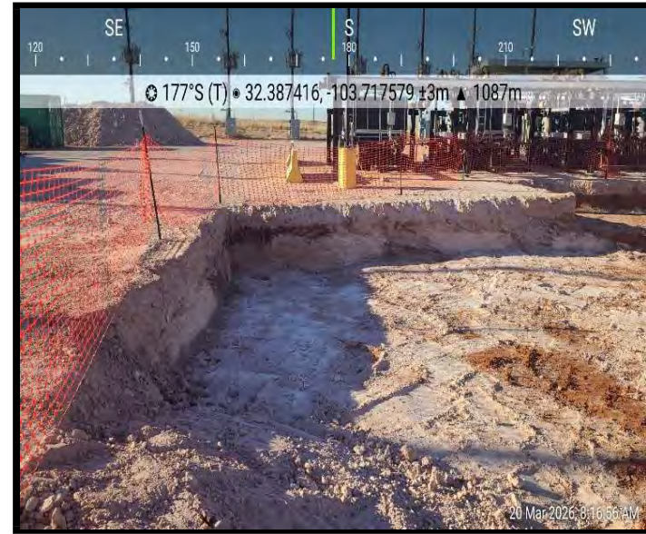
View of Excavation
