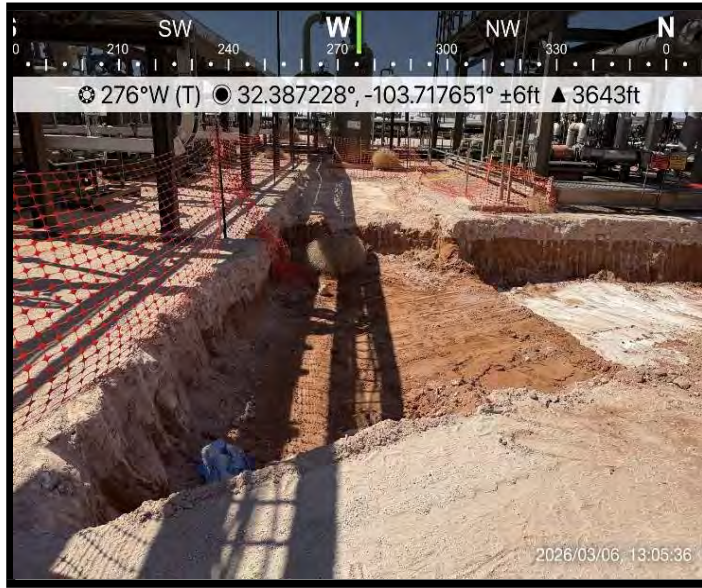
View of Excavation
