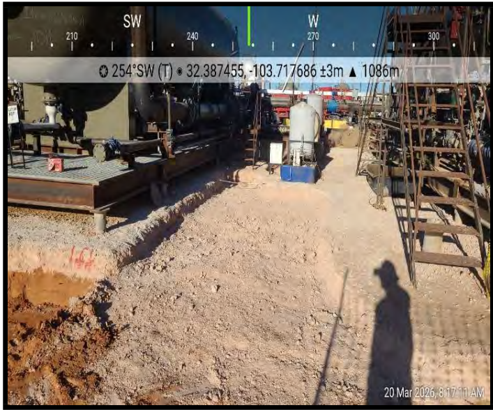
View of Excavation
