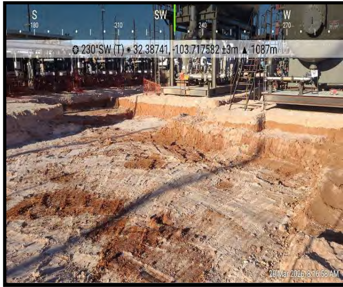
View of Excavation
