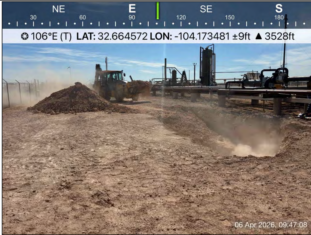
PHOTO 17: Southeastern view during restoration activities. 4/6/2026
