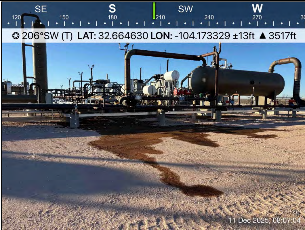
PHOTO 2: Southwestern view during initial site assessment activities. 12/11/2025
