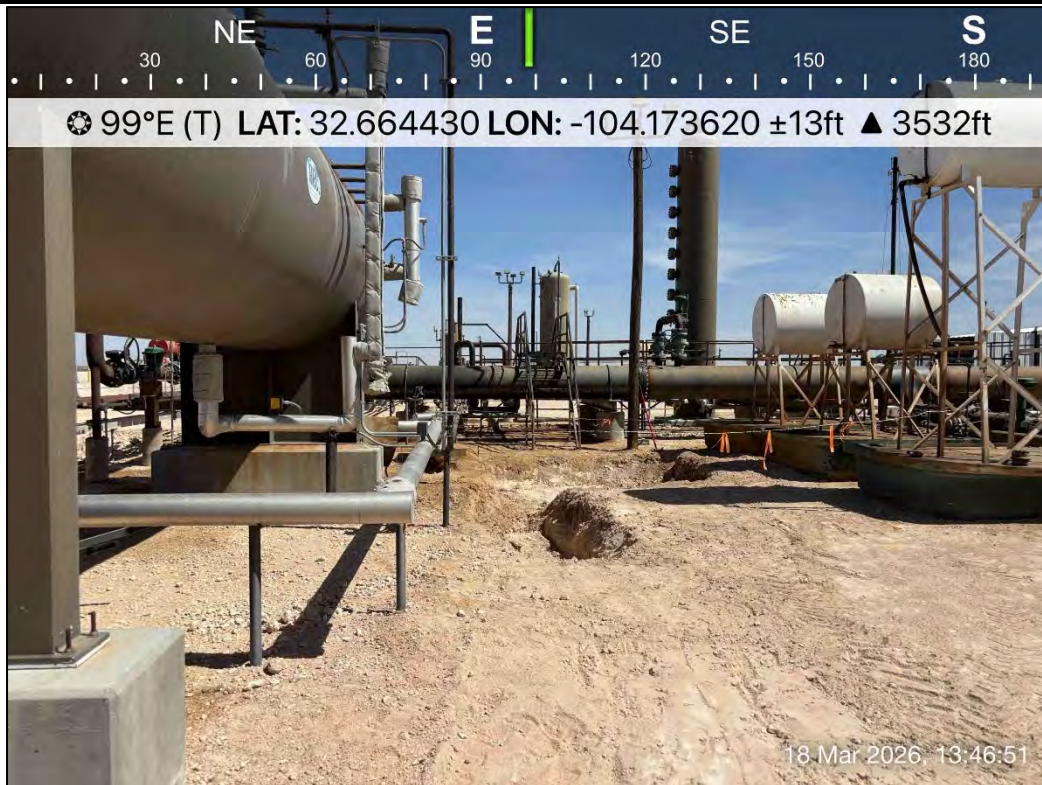
PHOTO 14: Eastern view of excavation extent. 3/18/2026
