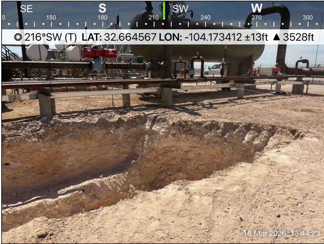
PHOTO 13: Southwestern view of excavation extent. 3/18/2026
