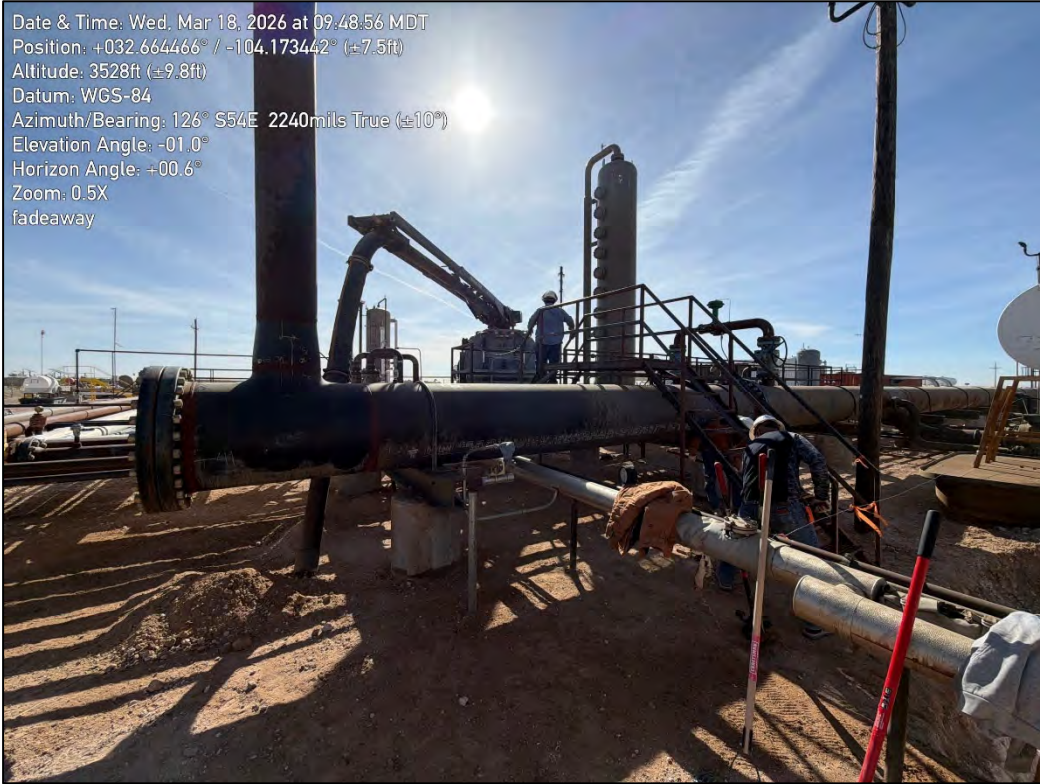
PHOTO 7: Southeastern view during excavation activities. 3/18/2026
