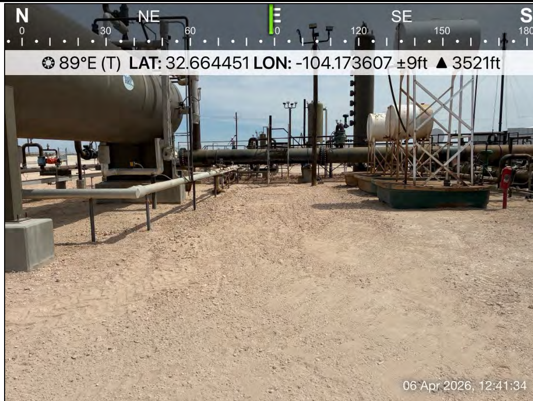
PHOTO 18: Eastern view following restoration activities. 4/6/2026
