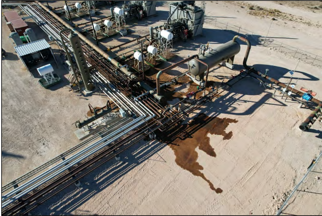
PHOTO 1: Southwestern aerial view during initial site assessment activities. 12/11/2025
