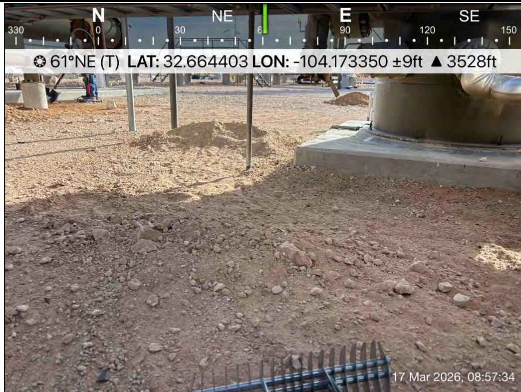
PHOTO 6: Northeastern view of excavation extent. 3/17/2026
