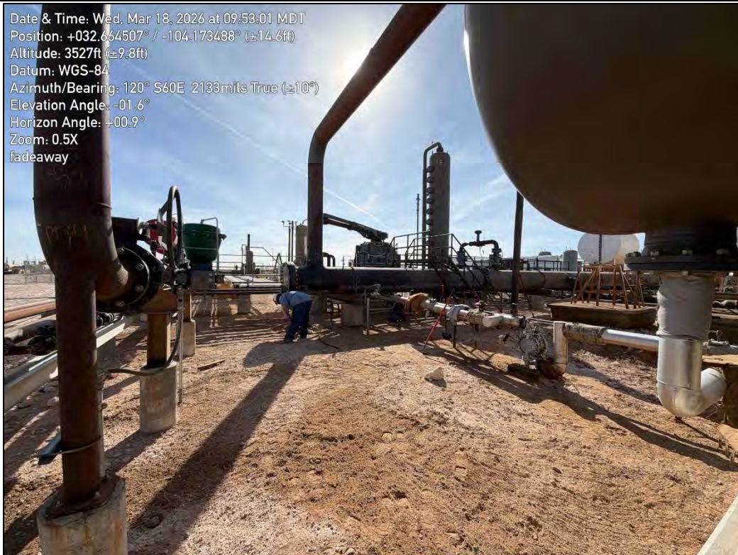
PHOTO 12: Southeastern view of excavation extent. 3/18/2026
