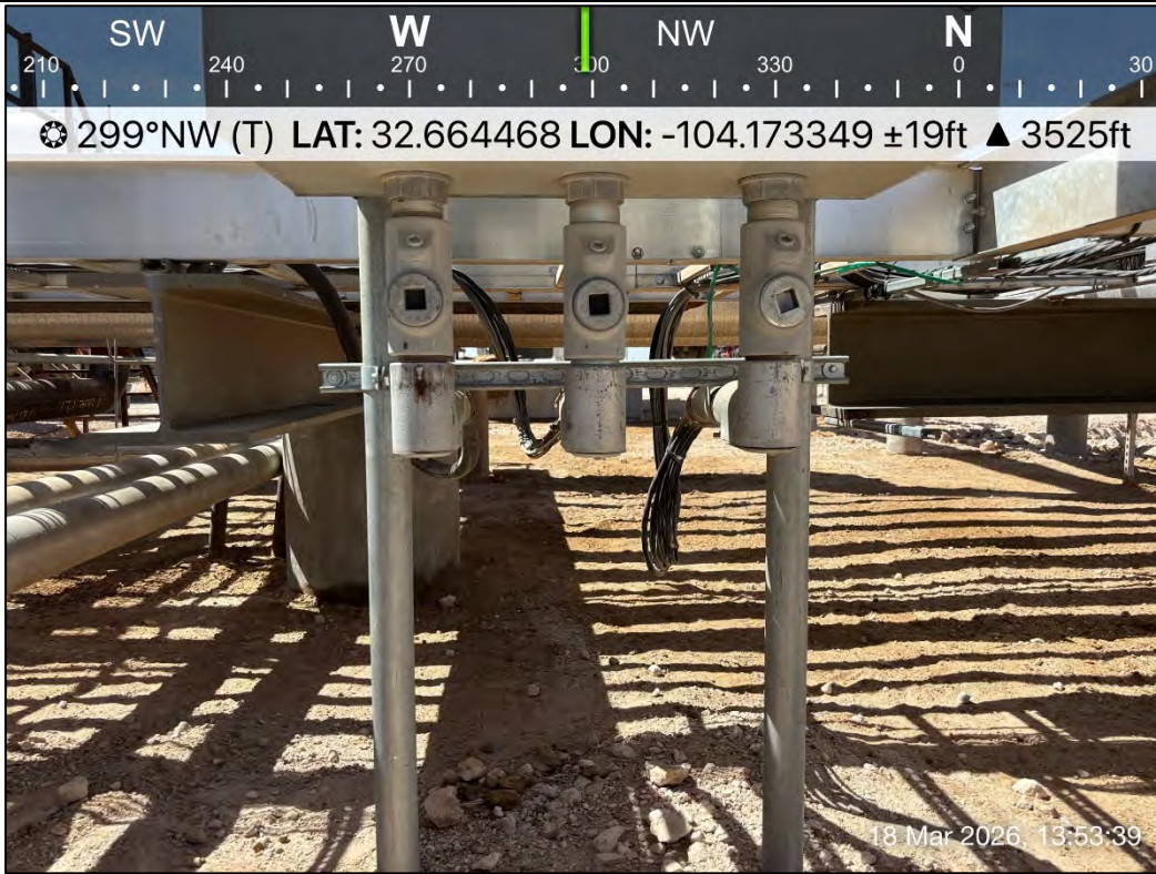
PHOTO 15: Northwestern view of excavation extent. 3/18/2026
