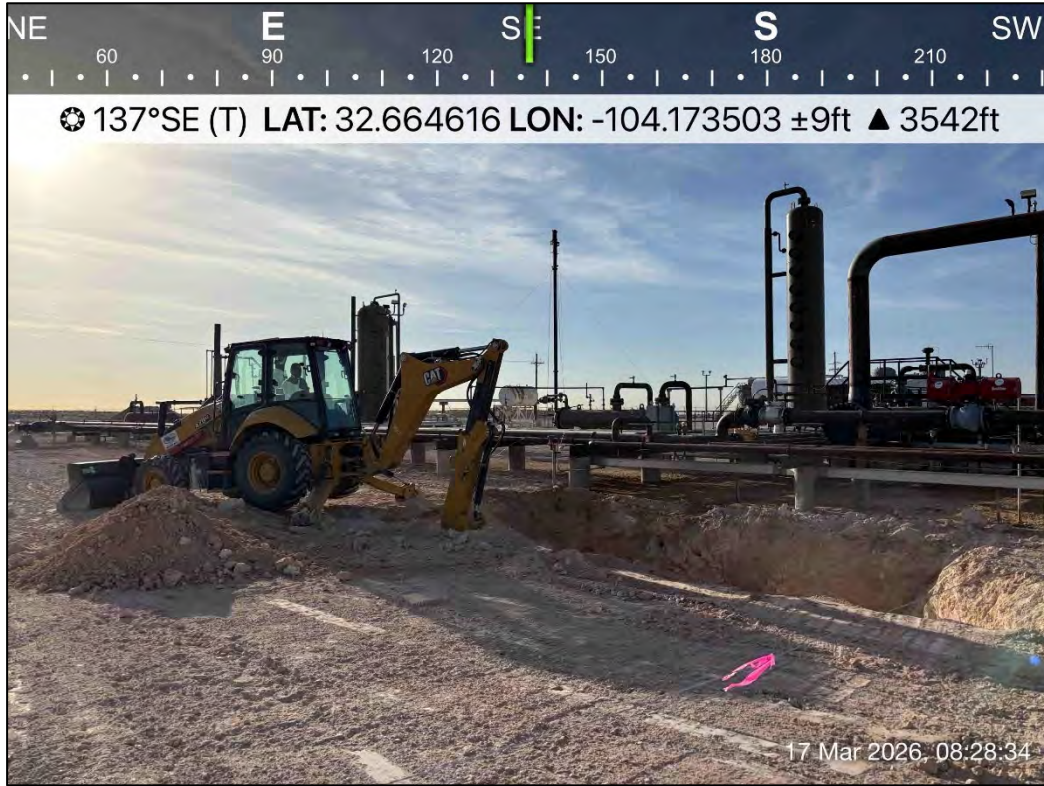
PHOTO 5: Southeastern view during excavation activities. 3/17/2026
