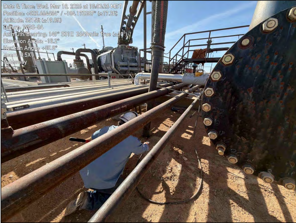
PHOTO 9: Southeastern view during excavation activities. 3/18/2026
