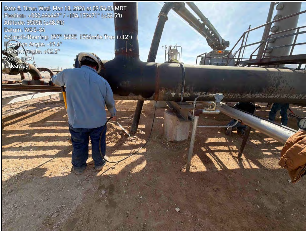
PHOTO 10: Southeastern view during excavation activities. 3/18/2026
