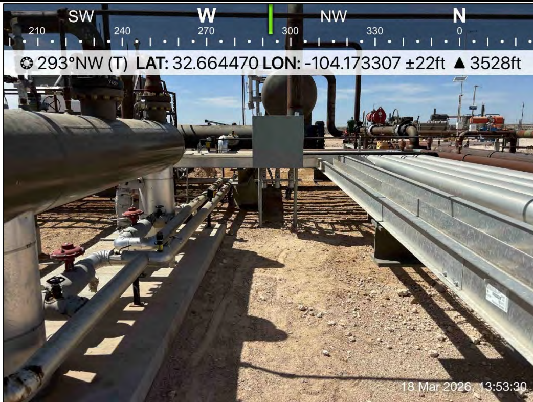
PHOTO 16: Northwestern view of excavation extent. 3/18/2026
