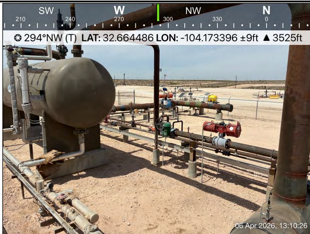
PHOTO 20: Northwestern view following restoration activities. 4/6/2026
