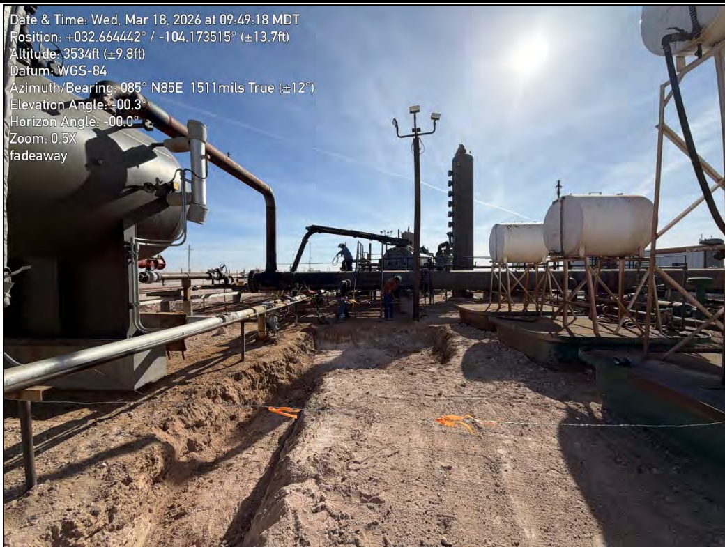
PHOTO 8: Northeastern view during excavation activities. 3/18/2026
