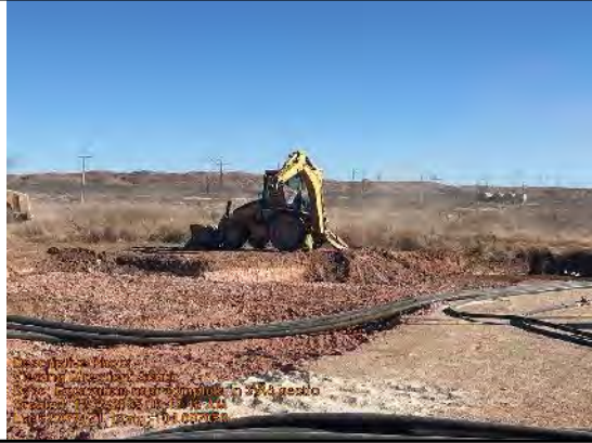
Excavation near complete in 3' section
