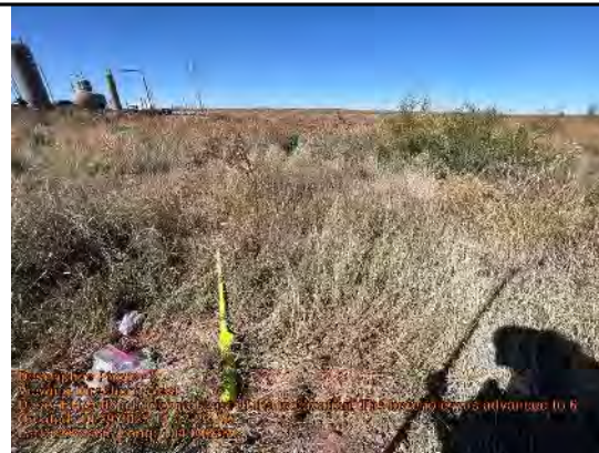
BH25-07 a horizontal east of the excavation. The borehole was advanced to 6ft to confirm no shallow karst features
