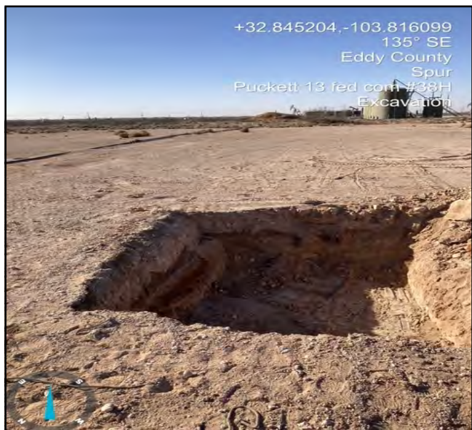
Photo taken during excavation process facing southeast.
