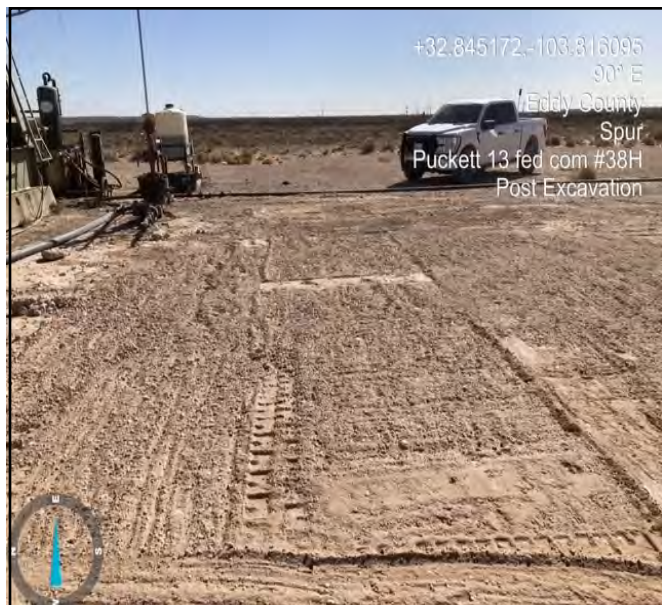
Photograph taken post excavation facing east.
