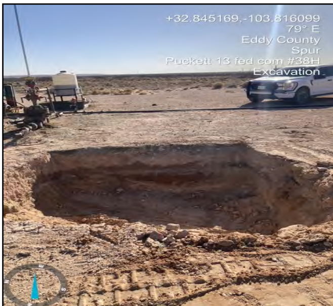
Photo taken during excavation process facing east.
