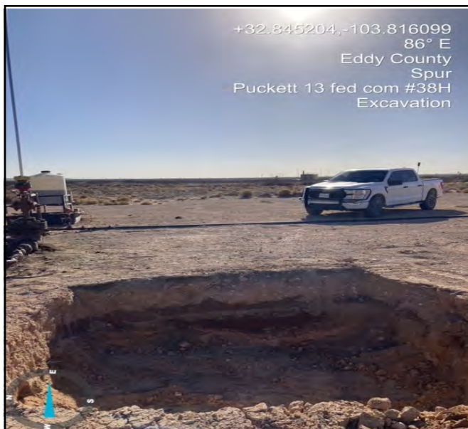
Photo taken during excavation process facing east.
