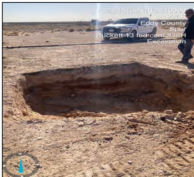
Photo taken during excavation process facing east.
