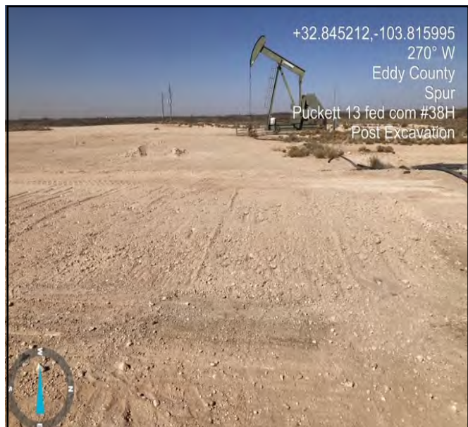
Photograph taken post excavation facing west.
