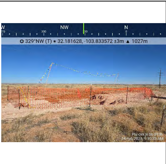
Photograph 4 Date: 2/24/2025 Description: Excavation extent, southern release area. View: Northwest
