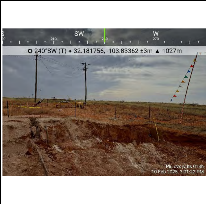
Photograph 1 Date: 2/10/2025 Description: Excavation extent, area of SW02/FS03. View: Southwest
