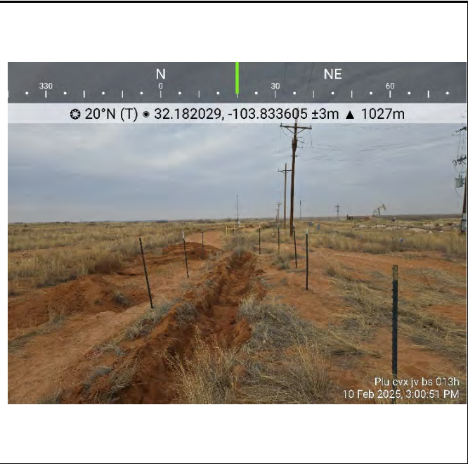
Photograph 2 Date: 2/10/2025 Description: Excavation extent, area of FS09. View: Northeast
