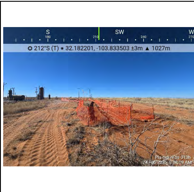
Photograph 3 Date: 2/24/2025 Description: Excavation extent, northern release area. View: South
