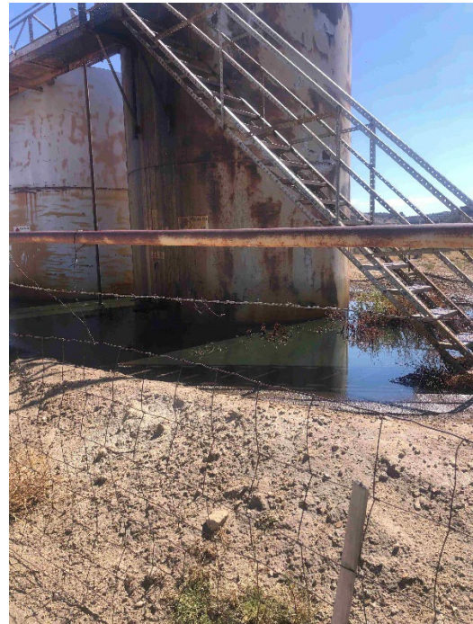
Initial release within secondary containment.
