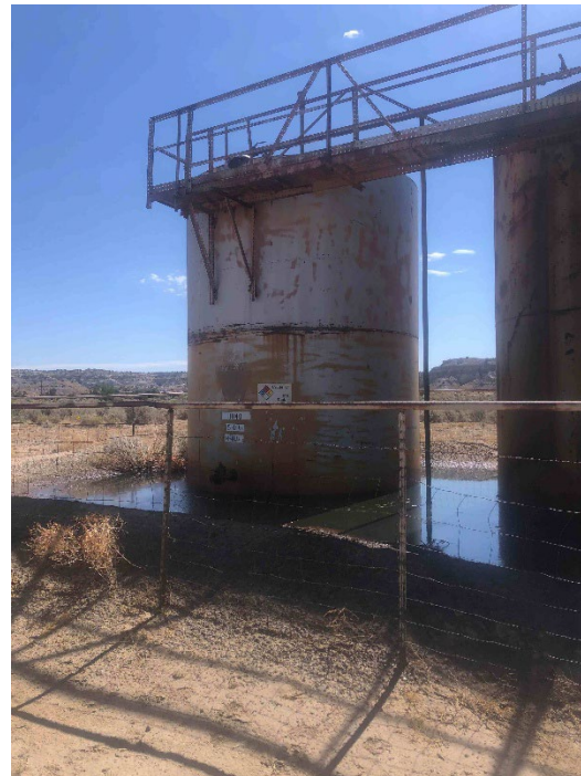
Initial release within secondary containment.
