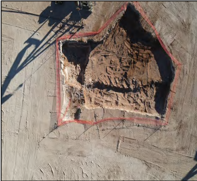
Aerial photo taken of excavation.
