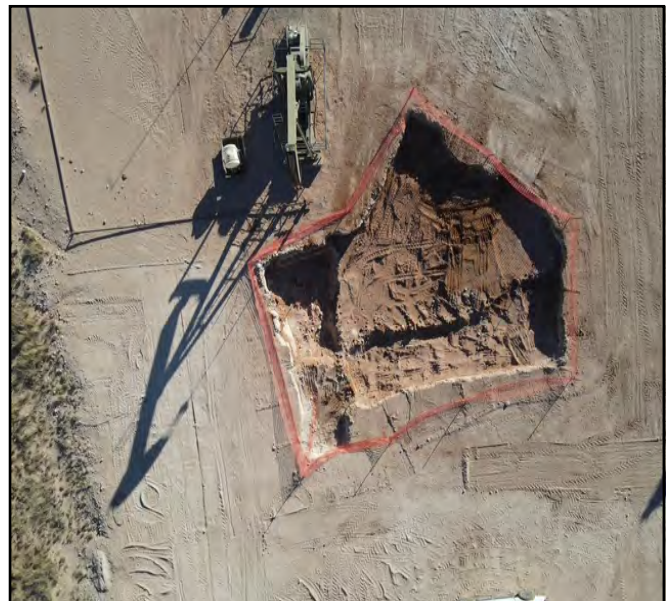
Aerial photo taken of excavation.
