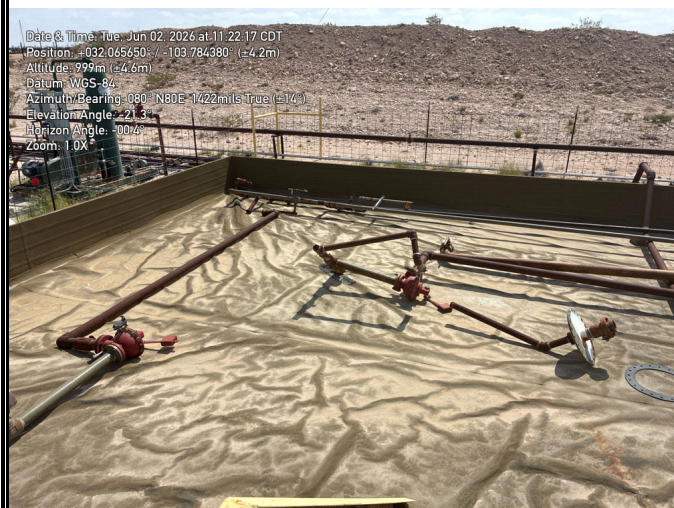
Photograph: 19 Date: 6/2/2026 Description: Liner deconstruction activities View: East
