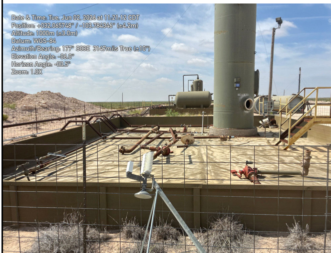
Photograph: 18 Date: 6/2/2026 Description: Liner deconstruction activities View: South
