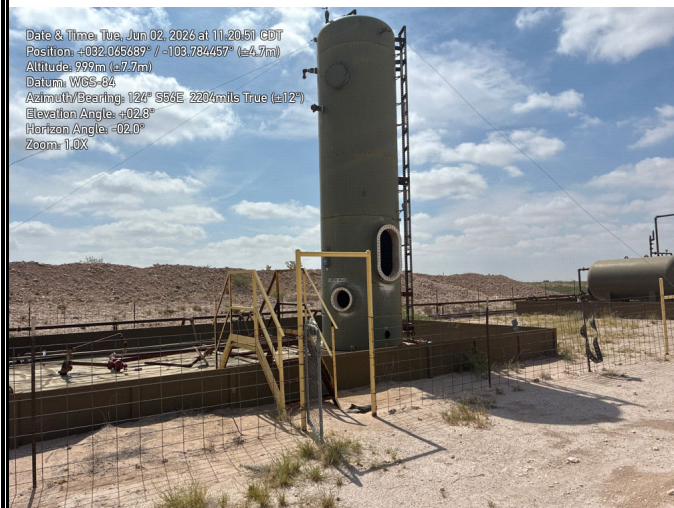
Photograph: 17 Date: 6/2/2026 Description: Liner deconstruction activities View: Southeast
