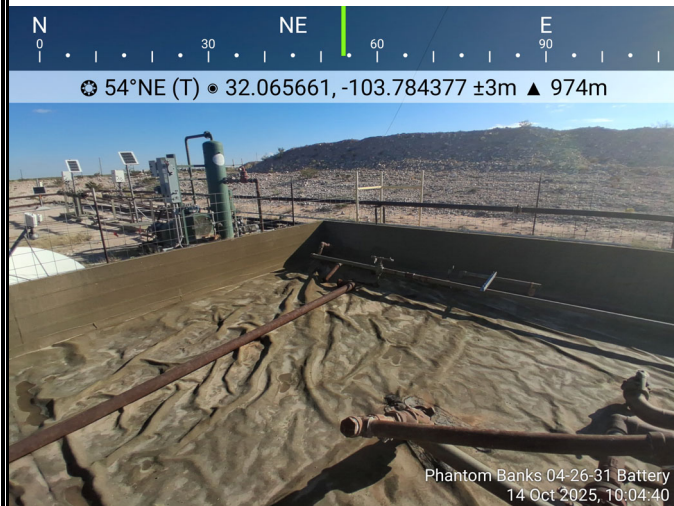
Photograph: 7 Date: 10/14/2025 Description: Liner inspection activities near northwest corner View: Northeast
