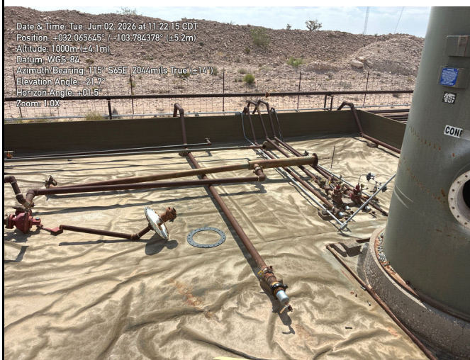
Photograph: 20 Date: 6/2/2026 Description: Liner deconstruction activities View: East
