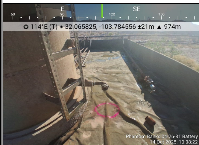
Photograph: 3 Date: 10/14/2025 Description: Liner inspection activities near identified holes (BH01) View: Southeast
