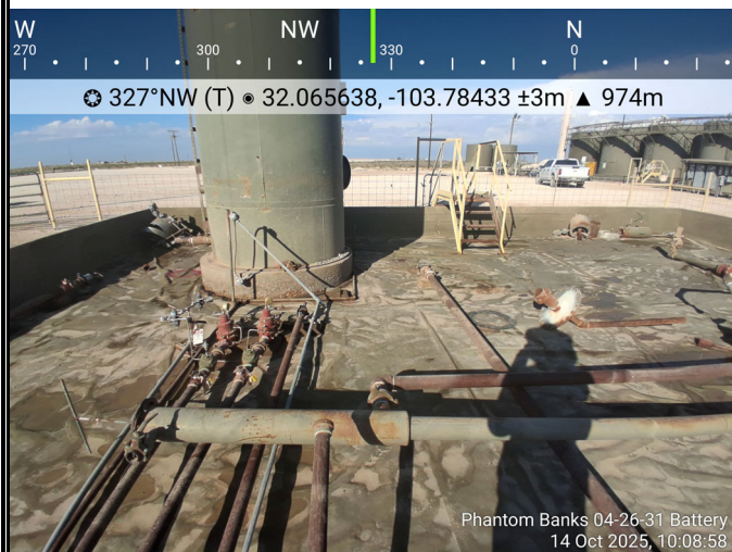
Photograph: 5 Date: 10/14/2025 Description: Liner inspection activities near central portion of liner View: Northwest
