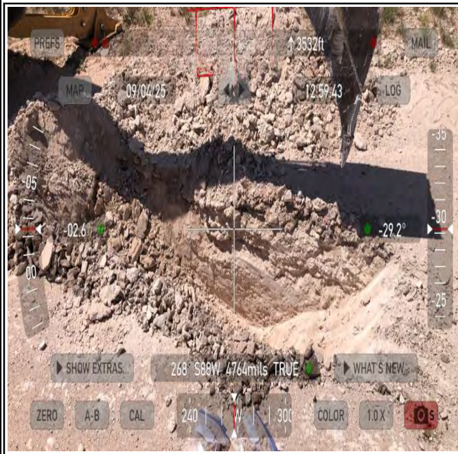
Photograph 7 Date: 09/04/2025 Description: Southwestern view of delineation activities near CR 245.
