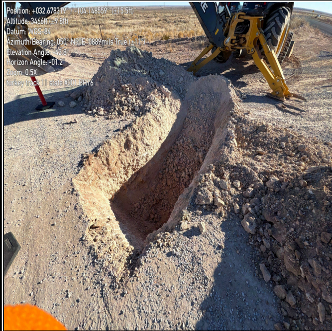
Photograph 9 Date: 02/06/2026 Description: Northeastern view of delineation activities near CR 245.
