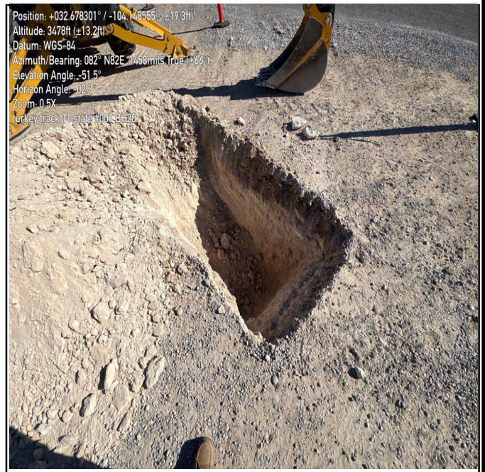
Photograph 12 Date: 02/06/2026 Description: Northeastern view of delineation activities near CR 245.
