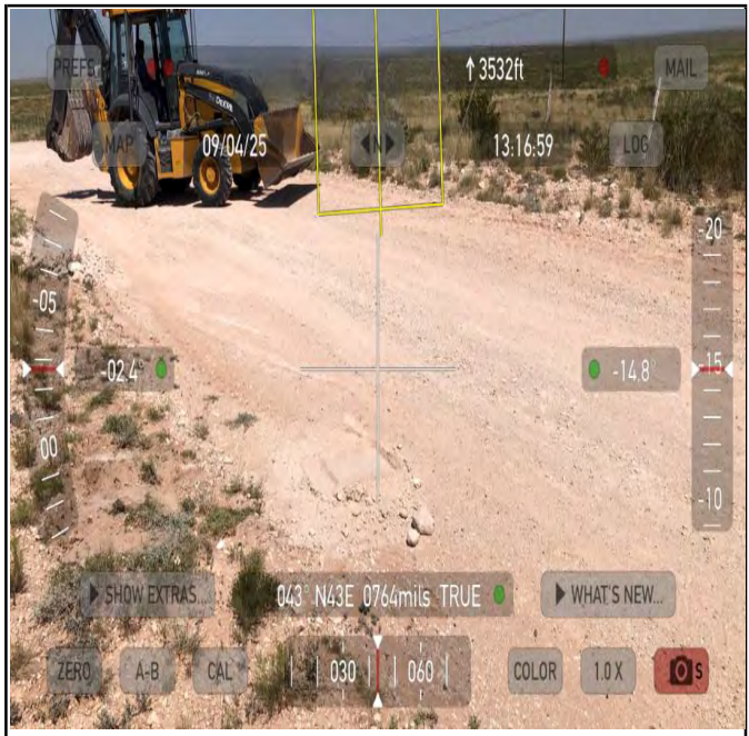
Photograph 8 Date: 09/04/2025 Description: Northeastern view of delineation activities on CR 245.
