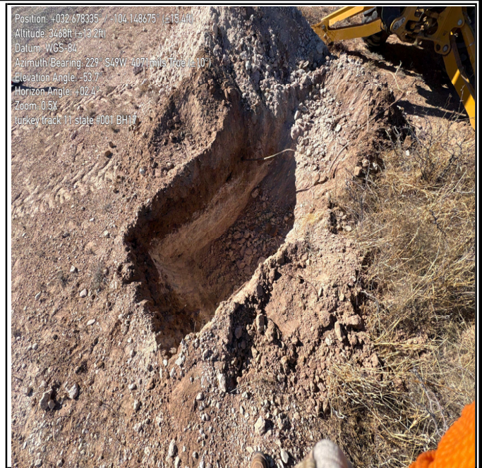
Photograph 10 Date: 02/06/2026 Description: Southwestern view of delineation activities near CR 245.
