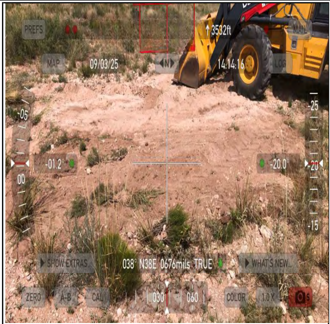
Photograph 6 Date: 09/03/2025 Description: Northeastern view of delineation activities on reclaimed pad.
