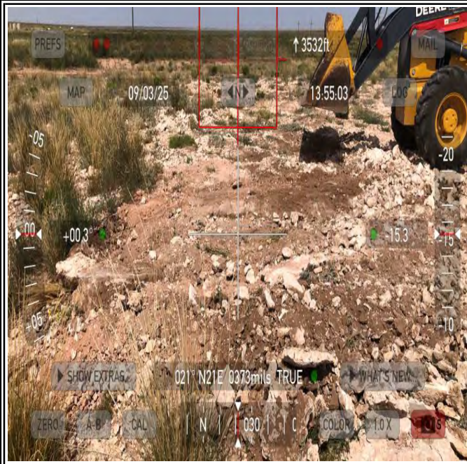
Photograph 5 Date: 09/03/2025 Description: Northeastern view of delineation activities on reclaimed pad.
