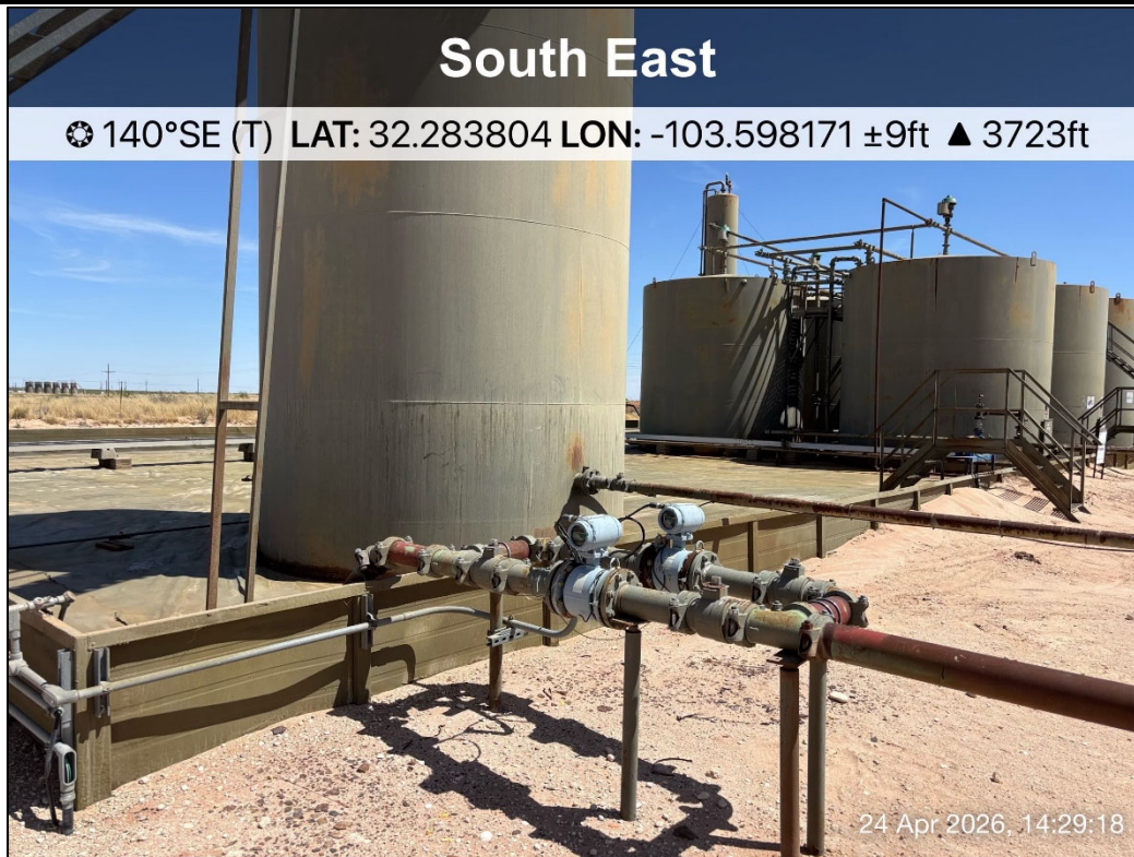
PHOTO 6: Southeastern view outside of containment during liner inspection activities. 4/24/2026
