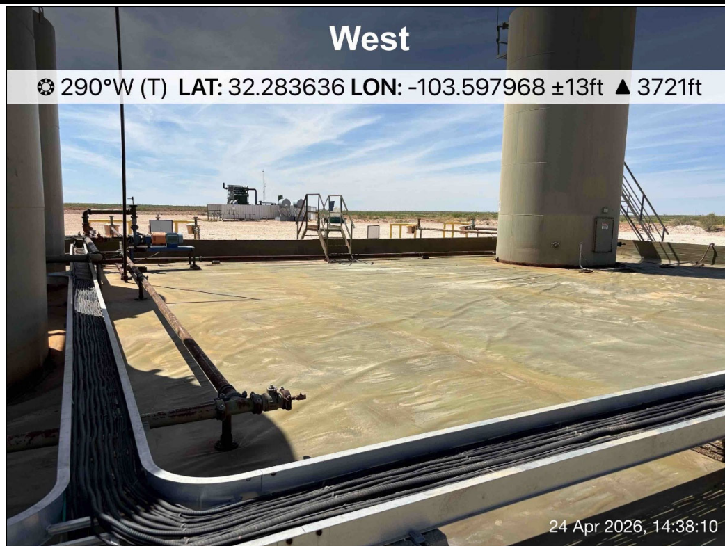
PHOTO 16: Western view during liner inspection activities. 4/24/2026
