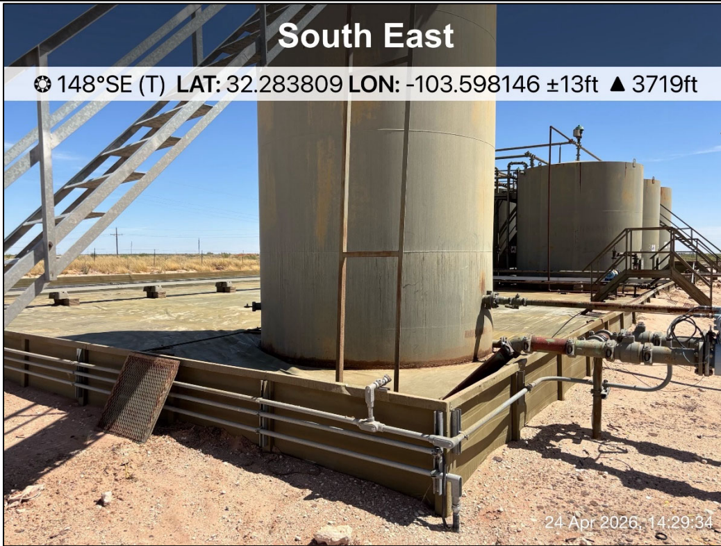
PHOTO 7: Southeastern view outside of containment during liner inspection activities. 4/24/2026
