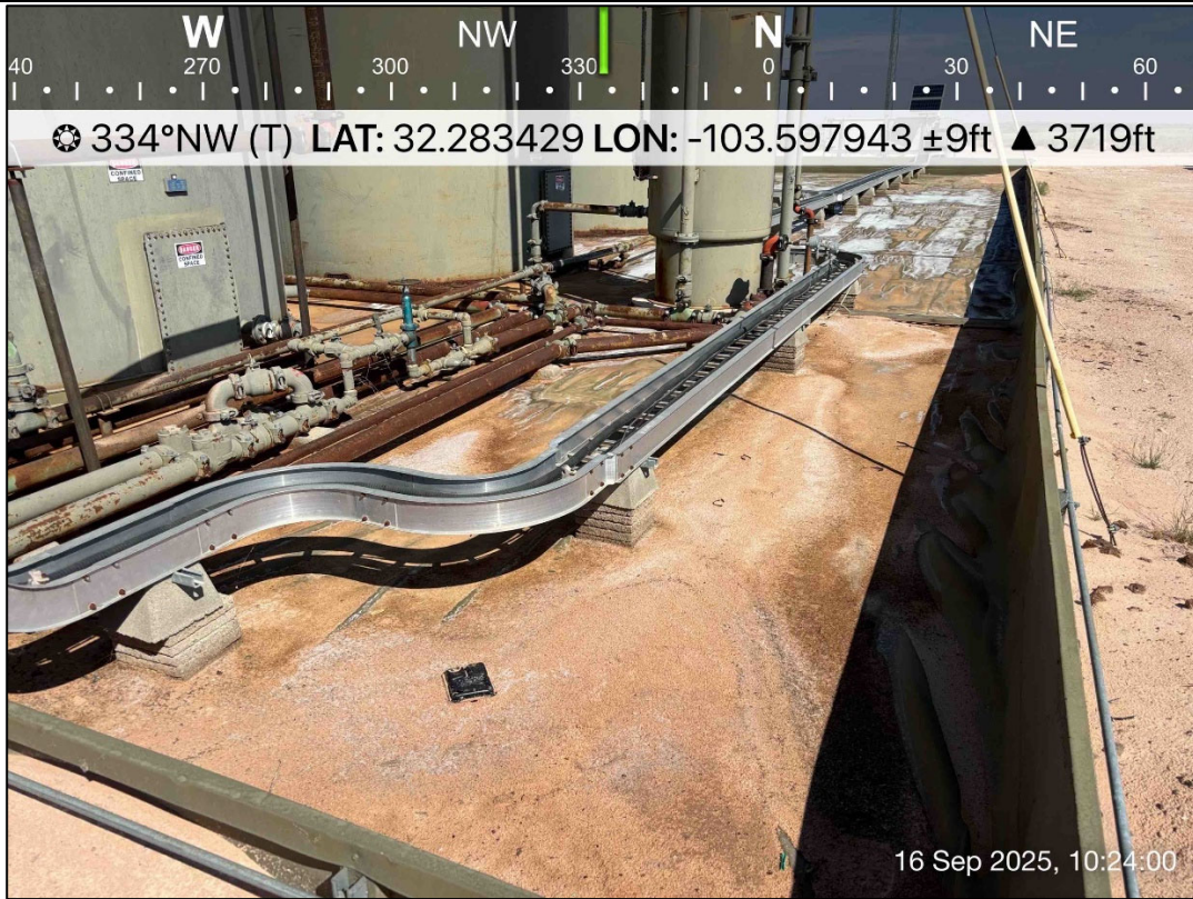
PHOTO 1: Northwestern view during initial site assessment. 9/16/2025
