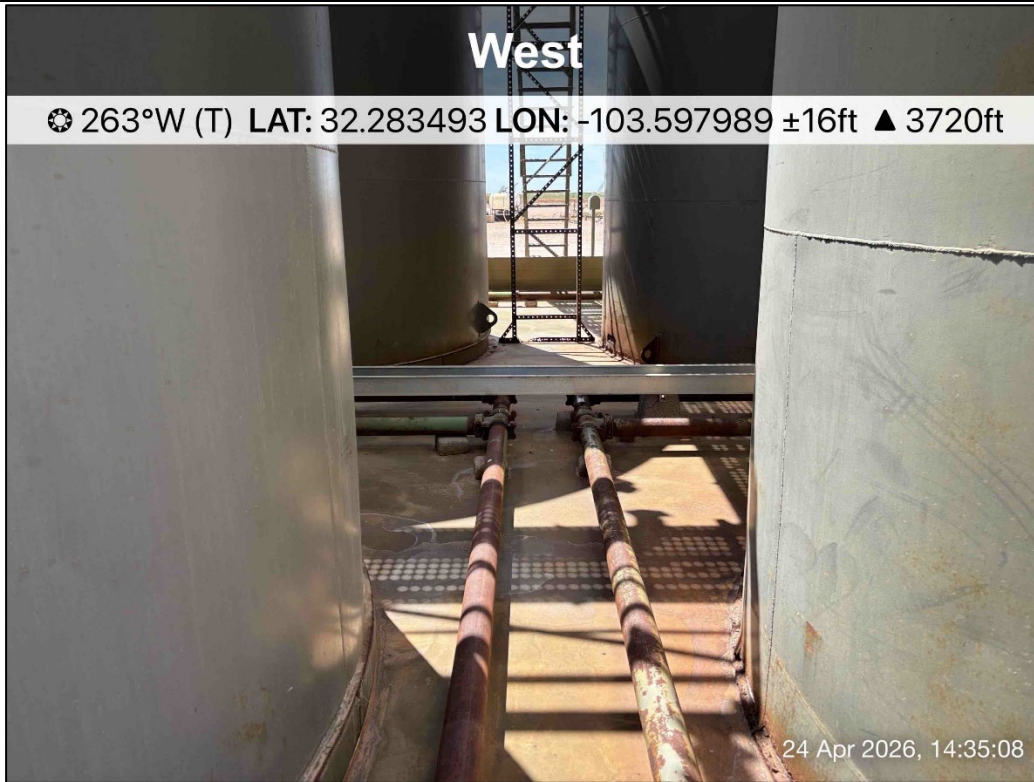
PHOTO 13: Western view during liner inspection activities. 4/24/2026
