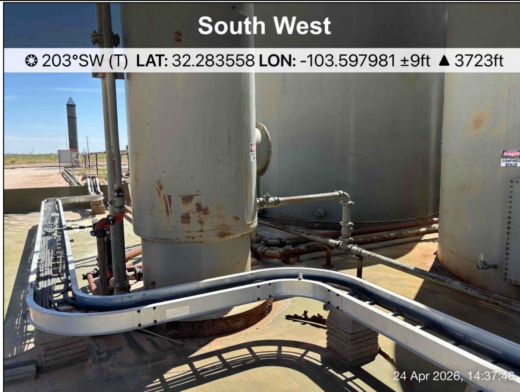
PHOTO 15: Southwestern view during liner inspection activities. 4/24/2026
