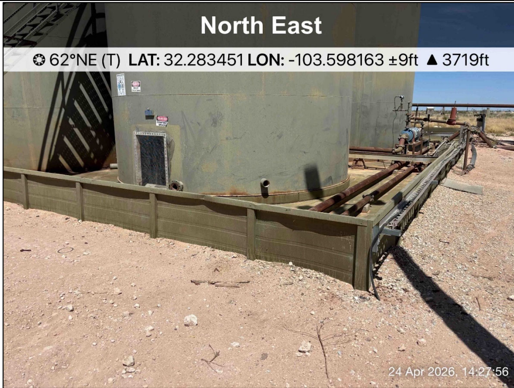
PHOTO 3: Northeastern view outside of containment during liner inspection activities. 4/24/2026
