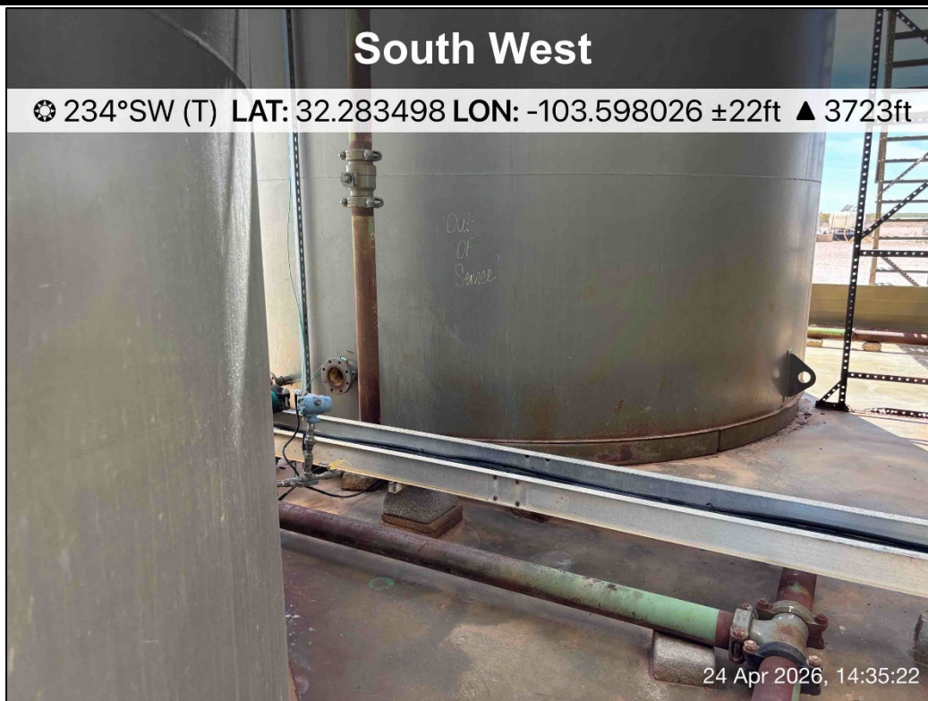
PHOTO 14: Southwestern view during liner inspection activities. 4/24/2026
