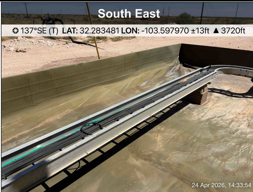
PHOTO 10: Southeastern view during liner inspection activities. 4/24/2026
