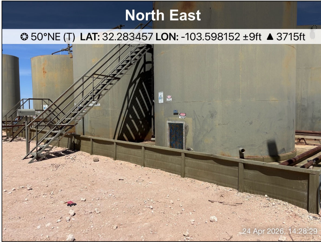
PHOTO 5: Northeastern view outside of containment during liner inspection activities. 4/24/2026
