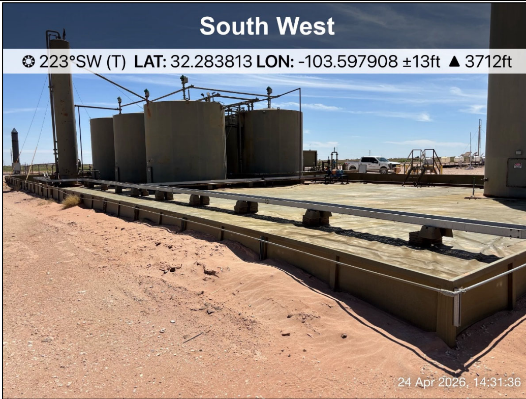
PHOTO 9: Southwestern view outside of containment during liner inspection activities. 4/24/2026
