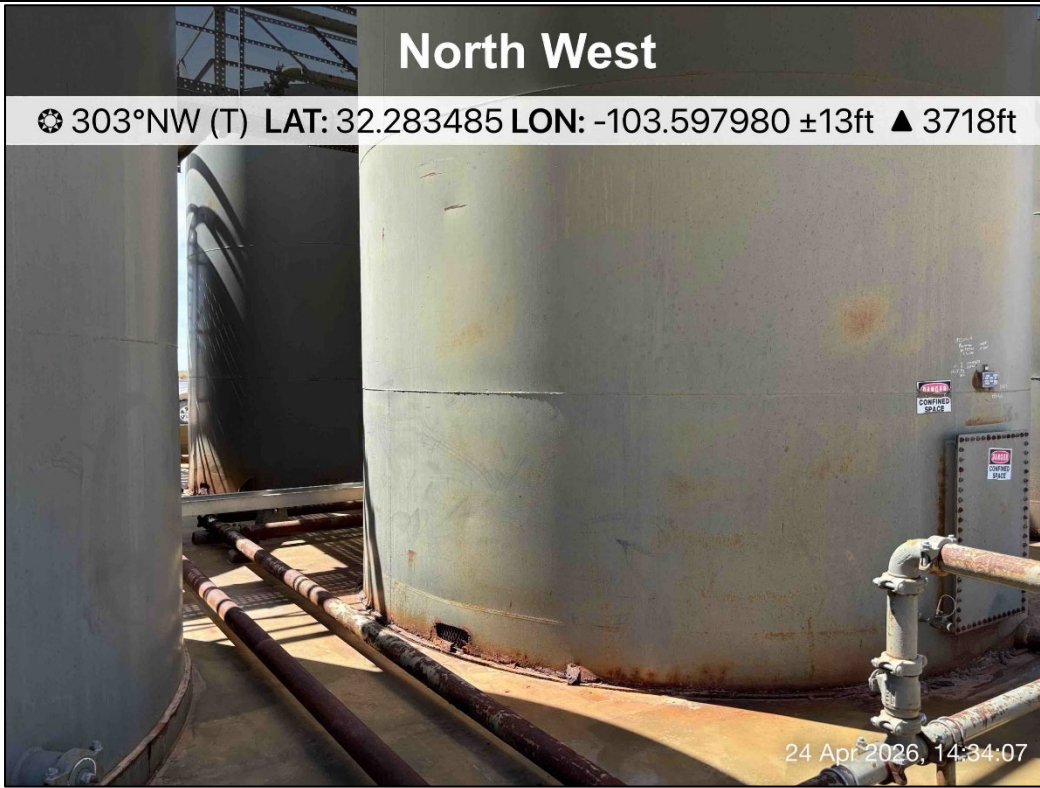
PHOTO 11: Northwestern view during liner inspection activities. 4/24/2026
