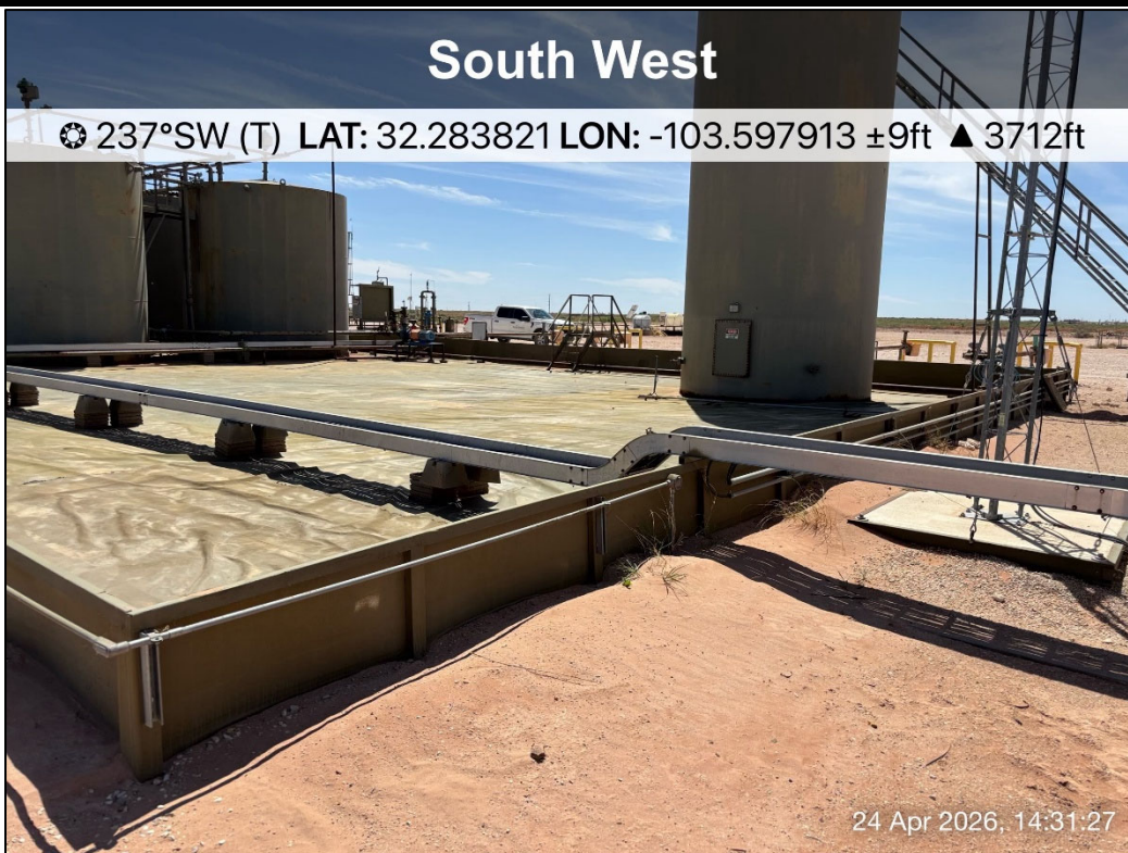
PHOTO 8: Southwestern view outside of containment during liner inspection activities. 4/24/2026
