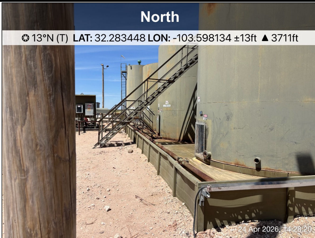
PHOTO 4: Northern view outside of containment during liner inspection activities. 4/24/2026
