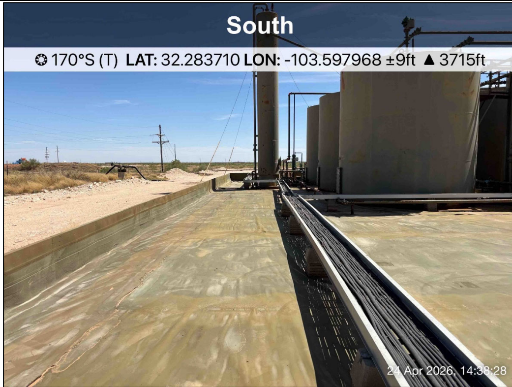
PHOTO 17: Southern view during liner inspection activities. 4/24/2026
