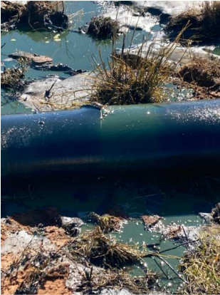
Cut on top of lay flat
