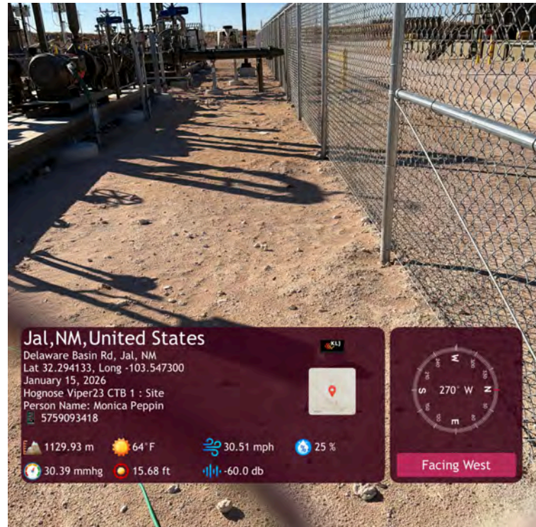
Visual staining along fence line.
