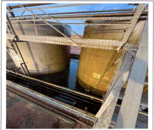
Initial photos provided by Devon Energy on 03/18/2026
