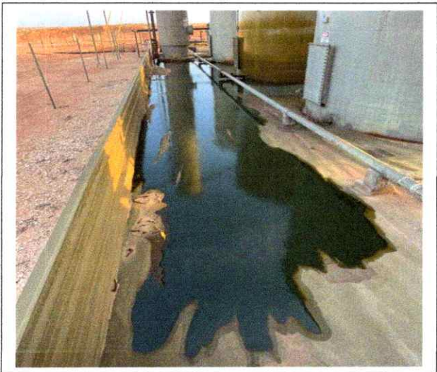
Initial photos provided by Devon Energy on 03/18/2026
