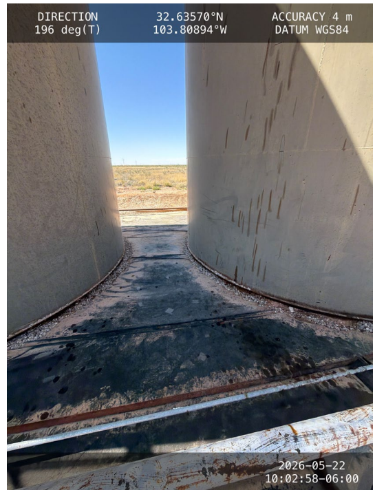
Photo 8 View between storage tanks within containment towards south.
