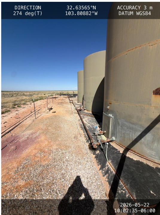
Photo 3 View of containment and site boundary towards west.
