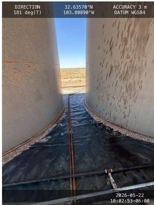
Photo 7 View between storage tanks within containment towards south.
