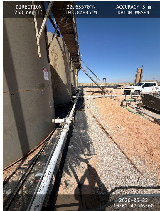
Photo 6 View of containment towards east.
