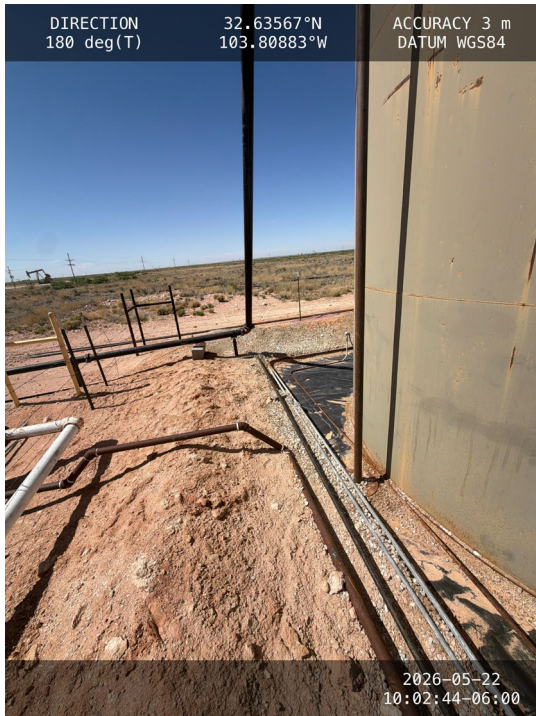
Photo 5 View of containment towards south.
