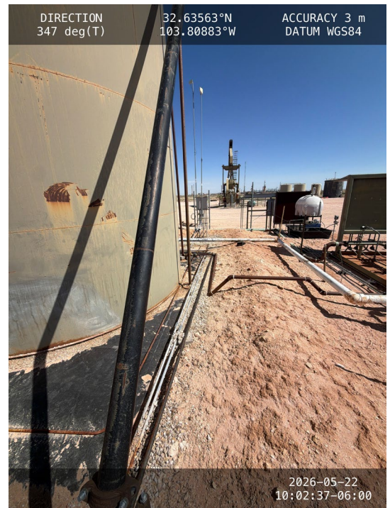
Photo 4 View of containment towards north.
