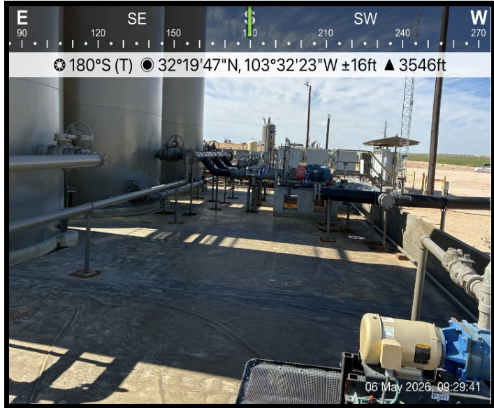
View of Liner
