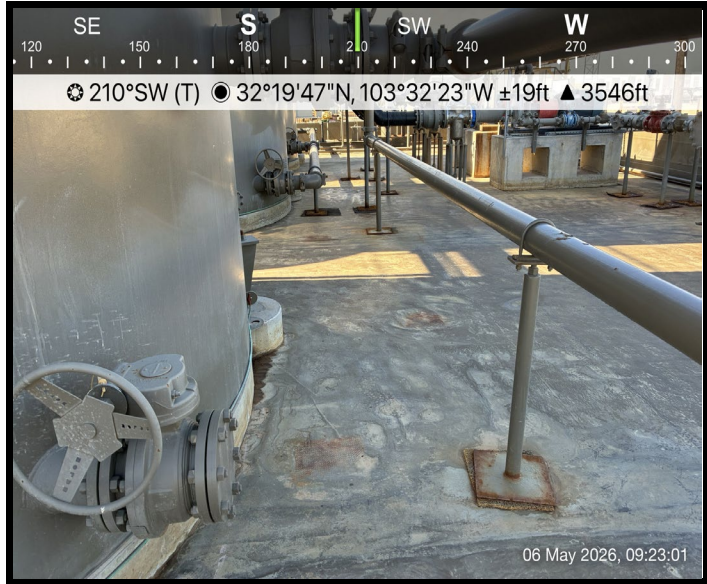
View of Liner
