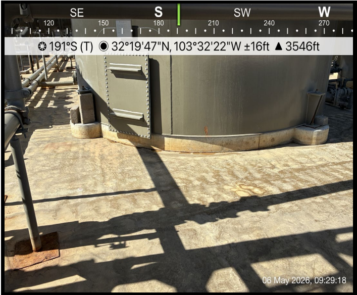
View of Liner
