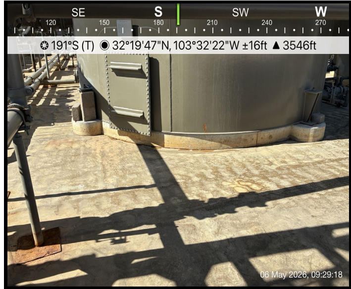
View of Liner
