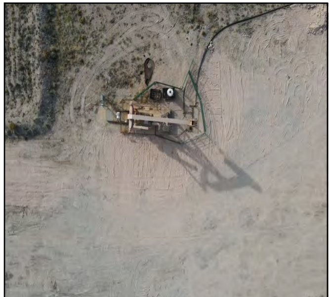
Aerial photo taken post excavation.
