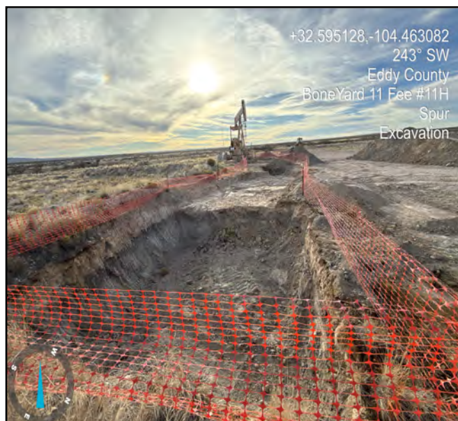
Photograph taken during the excavation process facing southwest.
