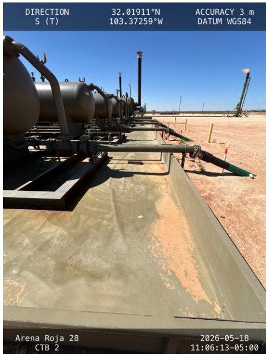
Photo 3 View of west side secondary containment towards south.
