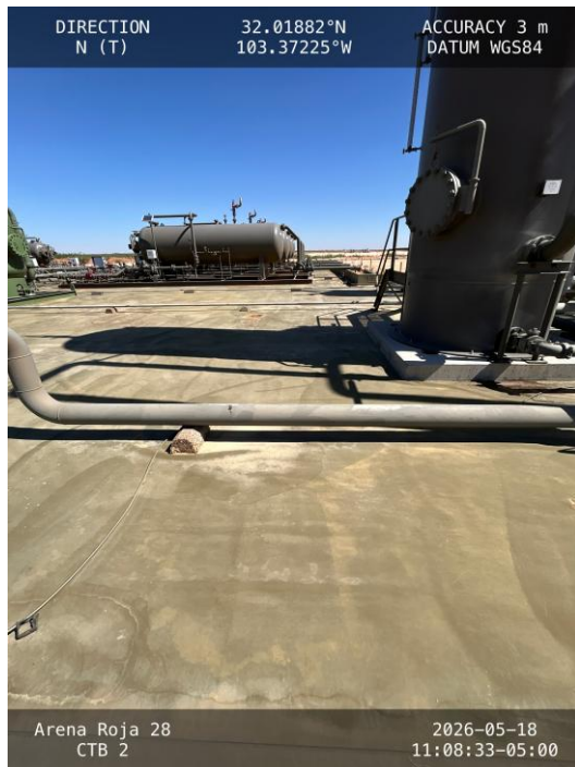
Photo 13 View of east side of secondary containment towards north.
