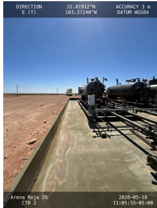
Photo 2 View of northern side containment area towards east.
