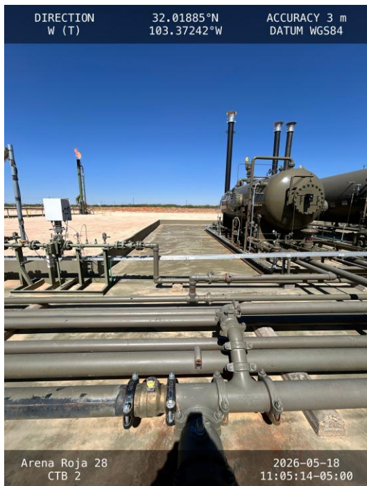
Photo 7 View of south side of containment towards west.
