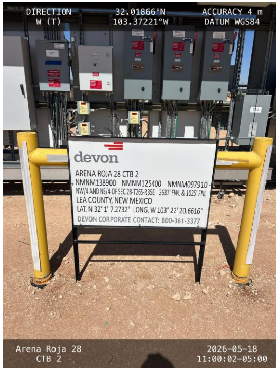
Photo 1 View of facility sign.
