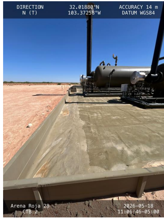
Photo 10 View of west side of secondary containment towards north.
