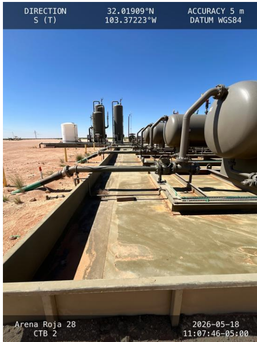
Photo 11 View of east side of secondary containment areas towards south.
