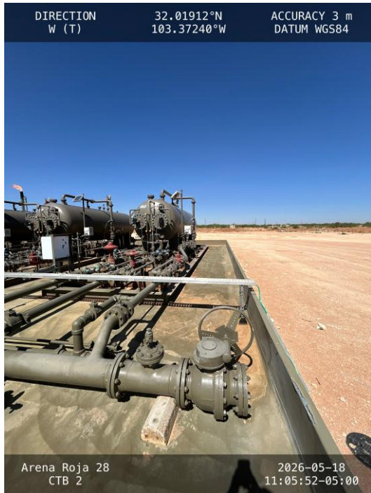
Photo 9 View of north side of secondary containment towards west.
