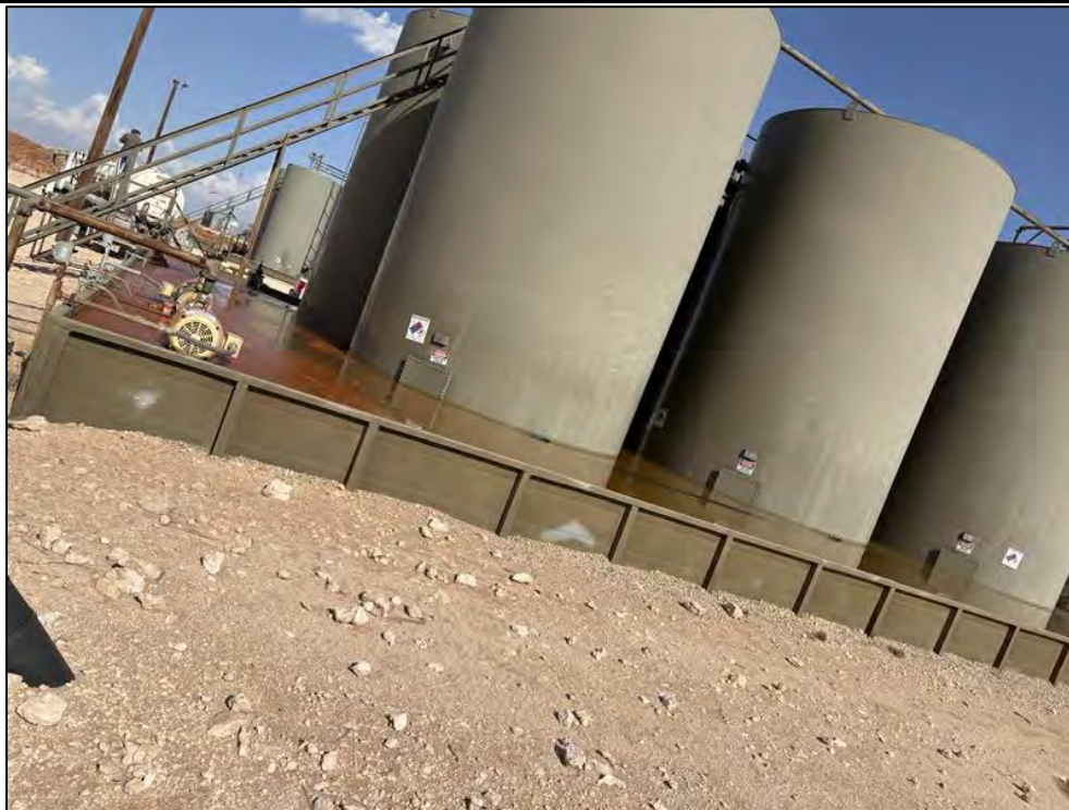
PHOTO 1: Eastern view during initial site assessment by Devon. 4/25/2025
