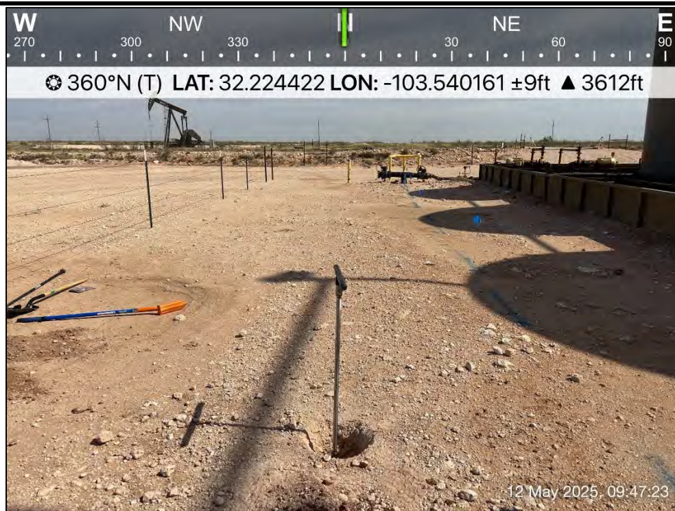
PHOTO 5: Northern view during initial delineation activities. 5/12/2025
