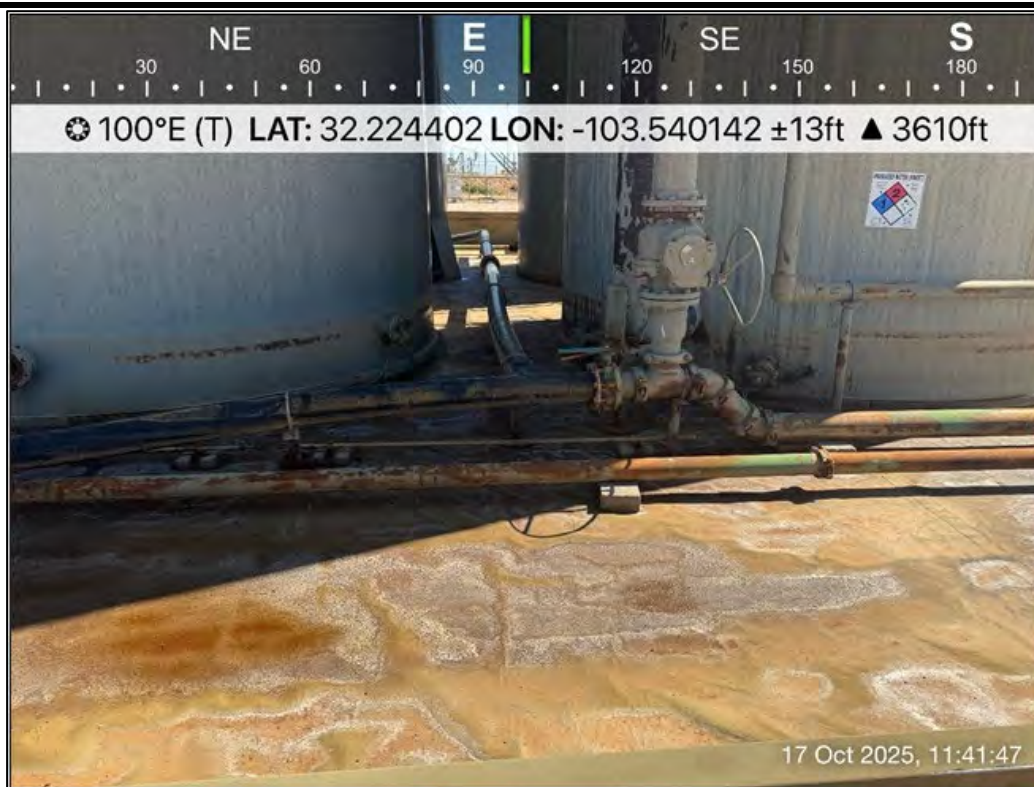
PHOTO 23: Eastern view during liner inspection activities. 10/17/2025
