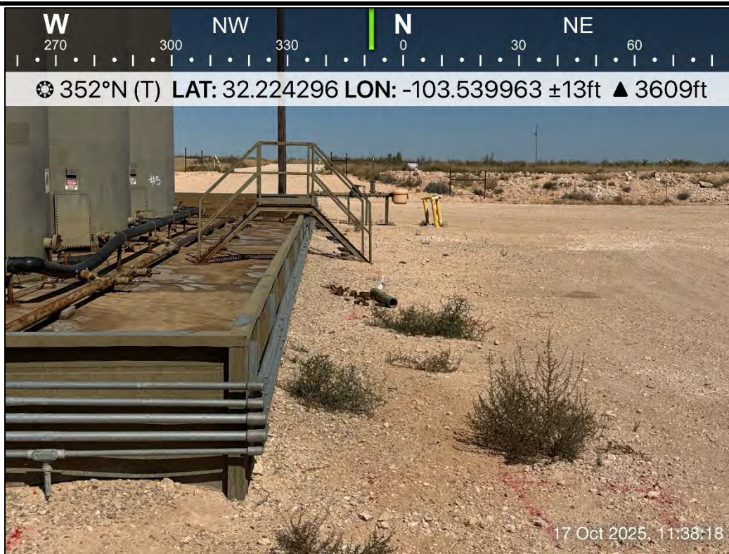
PHOTO 15: Northern view outside of containment during liner inspection activities. 10/17/2025
