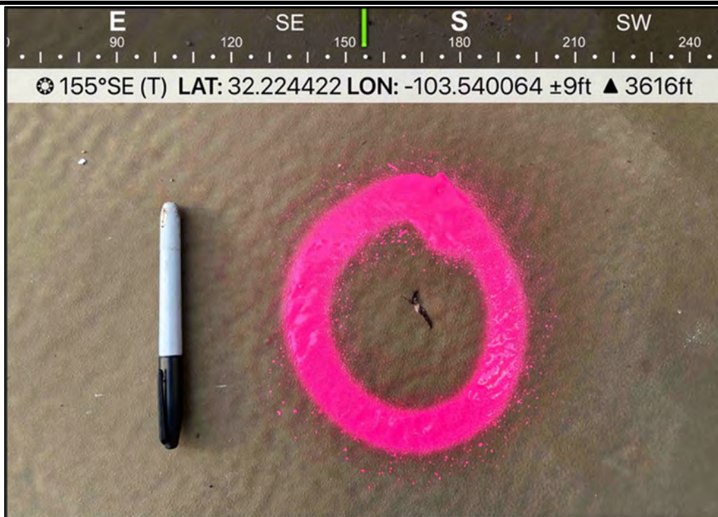
PHOTO 28: Southeastern view during liner inspection activities. 10/17/2025
