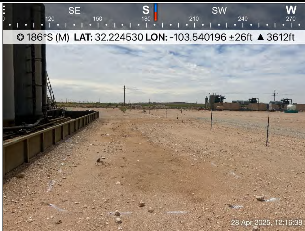
PHOTO 3: Southern view during site assessment by ESRR. 4/28/2025
