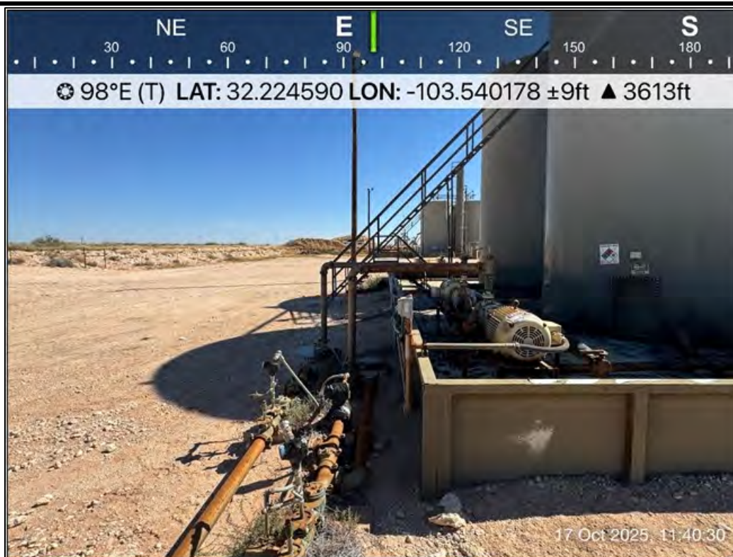
PHOTO 17: Eastern view outside of containment during liner inspection activities. 10/17/2025
