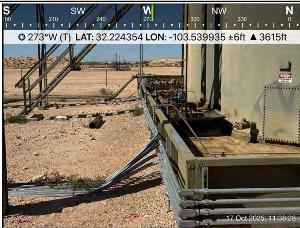
PHOTO 14: Western view outside of containment during liner inspection activities. 10/17/2025
