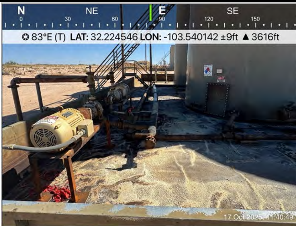
PHOTO 20: Eastern view during liner inspection activities. 10/17/2025
