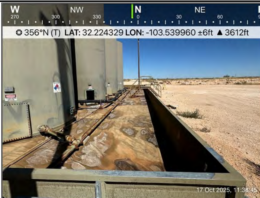
PHOTO 19: Northern view during liner inspection activities. 10/17/2025
