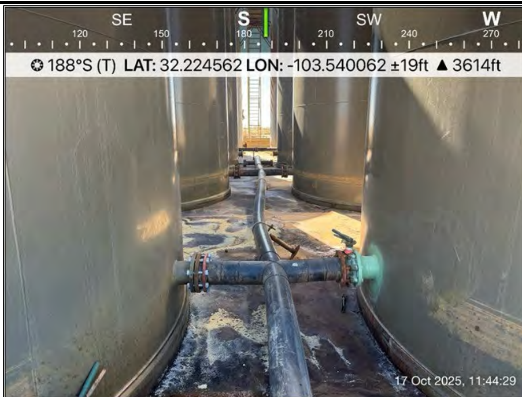
PHOTO 25: Southern view during liner inspection activities. 10/17/2025
