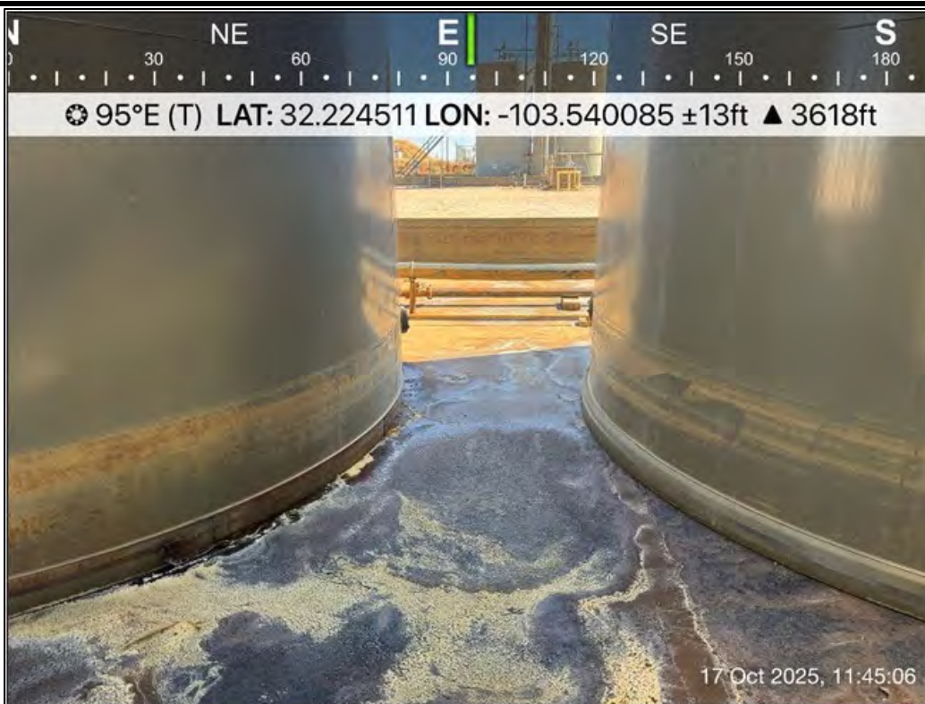
PHOTO 26: Eastern view during liner inspection activities. 10/17/2025
