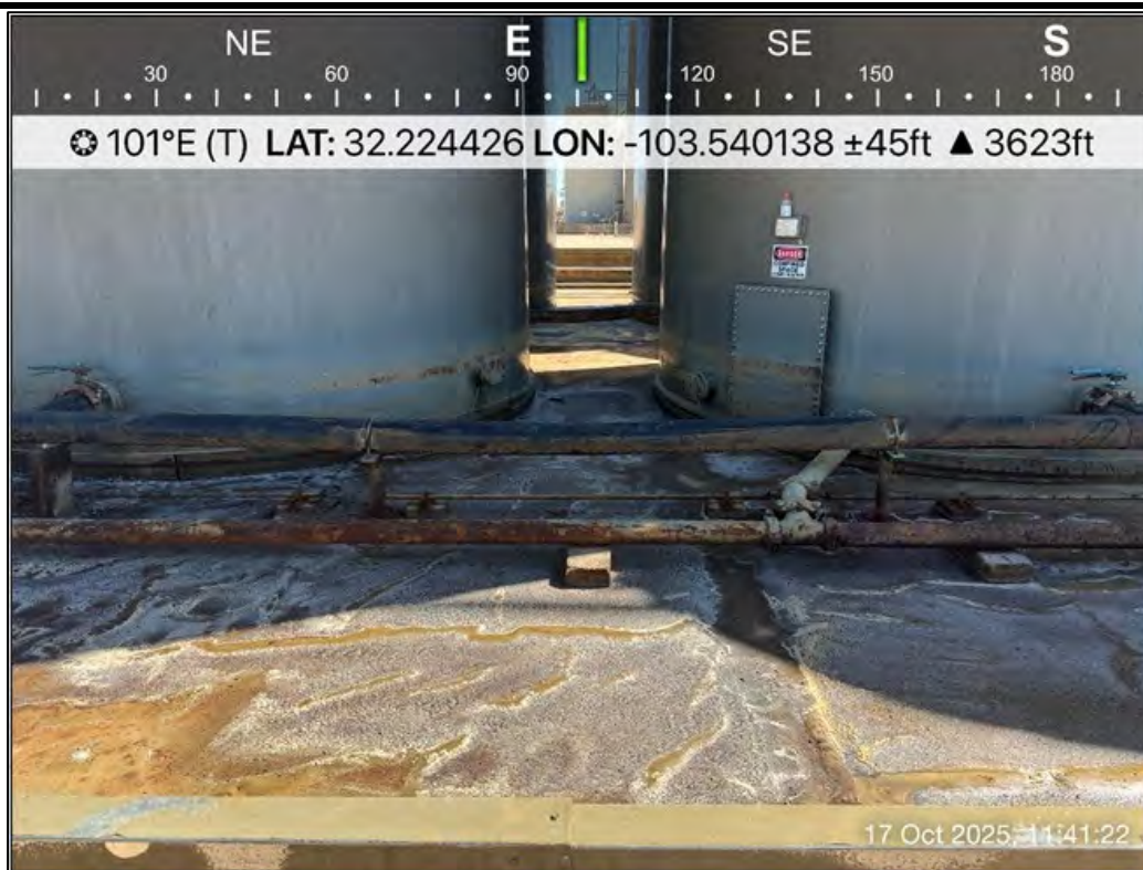
PHOTO 21: Southeastern view during liner inspection activities. 10/17/2025
