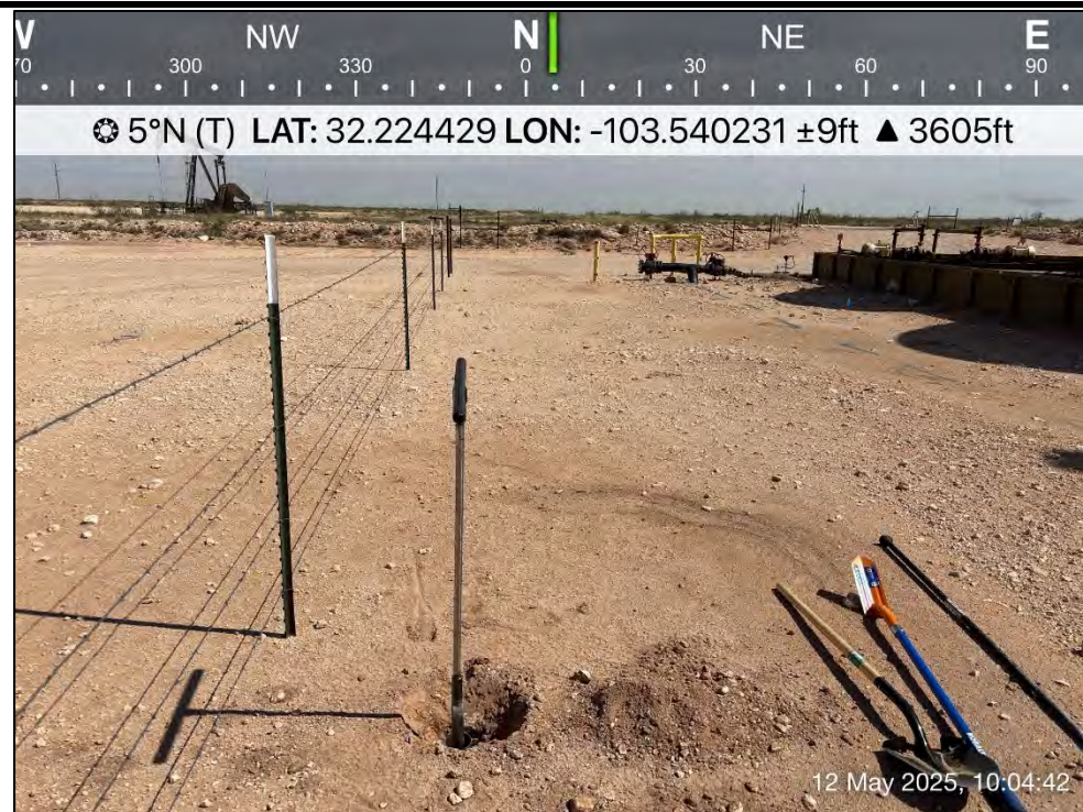
PHOTO 6: Northern view during initial delineation activities. 5/12/2025
