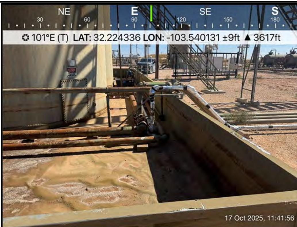
PHOTO 24: Southeastern view during liner inspection activities. 10/17/2025
