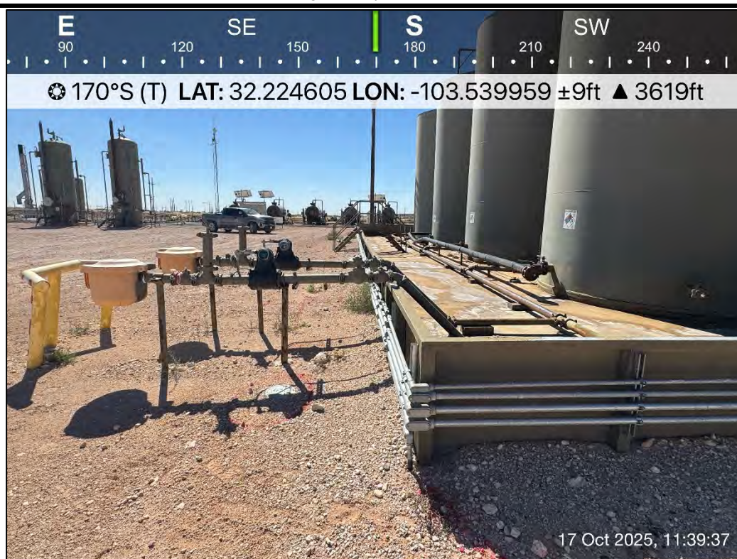
PHOTO 16: Southeastern view outside of containment during liner inspection activities. 10/17/2025
