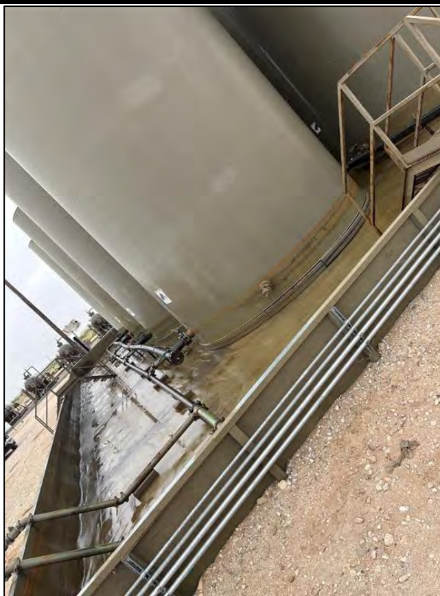
PHOTO 2: Southern view during initial site assessment by Devon. 4/25/2025
