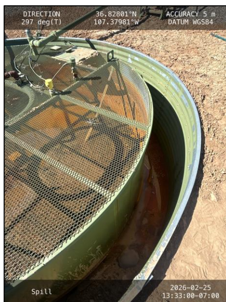
Photograph: 1 Date: 02/25/2026 Description: The source of the release and standing fluid within the BGT containment pit. View: West
