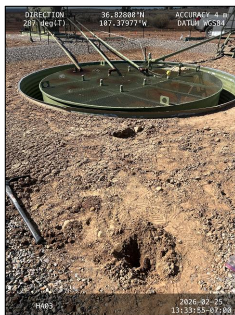
Photograph: 4 Date: 02/25/2026 Description: Hand auger boring HA03, advanced to the east of the source of the release. View: West
