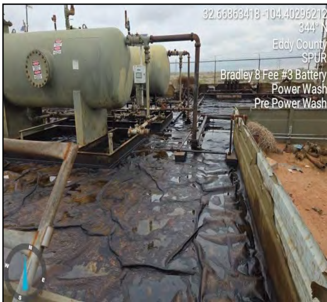
Photograph taken pre powerwash facing north.
