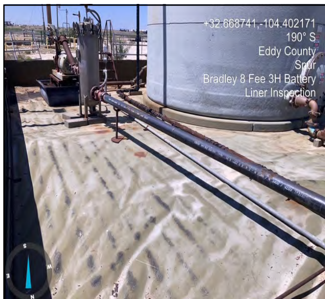
Photograph taken conducting Liner inspection facing south.
