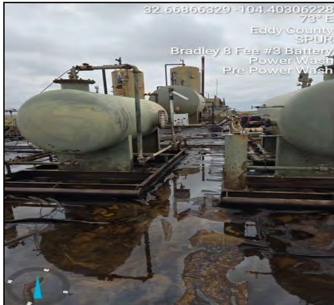
Photograph taken pre powerwash facing east.
