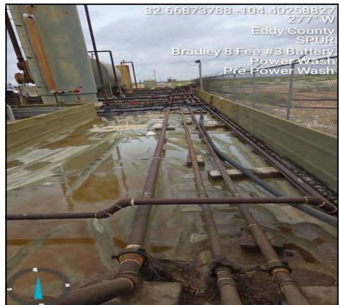
Photograph taken pre powerwash facing west.
