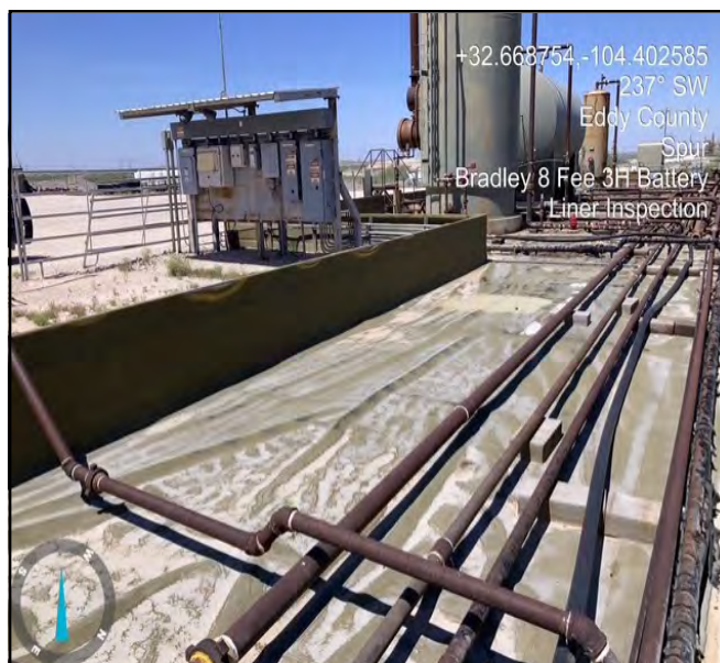
Photograph taken conducting Liner inspection facing southwest.
