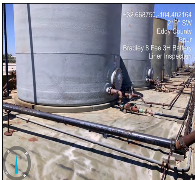
Photograph taken conducting Liner inspection facing southwest.
