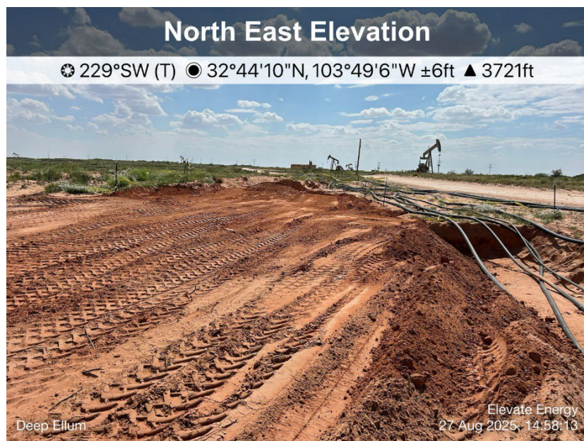
Backfill In Progress
