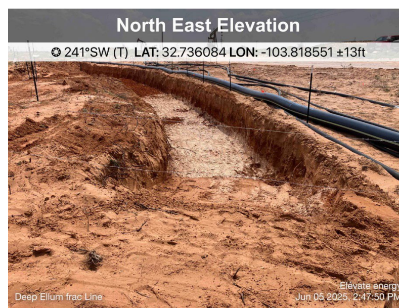
Excavation in Progress
