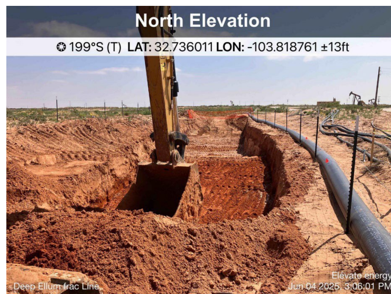
Excavation in Progress
