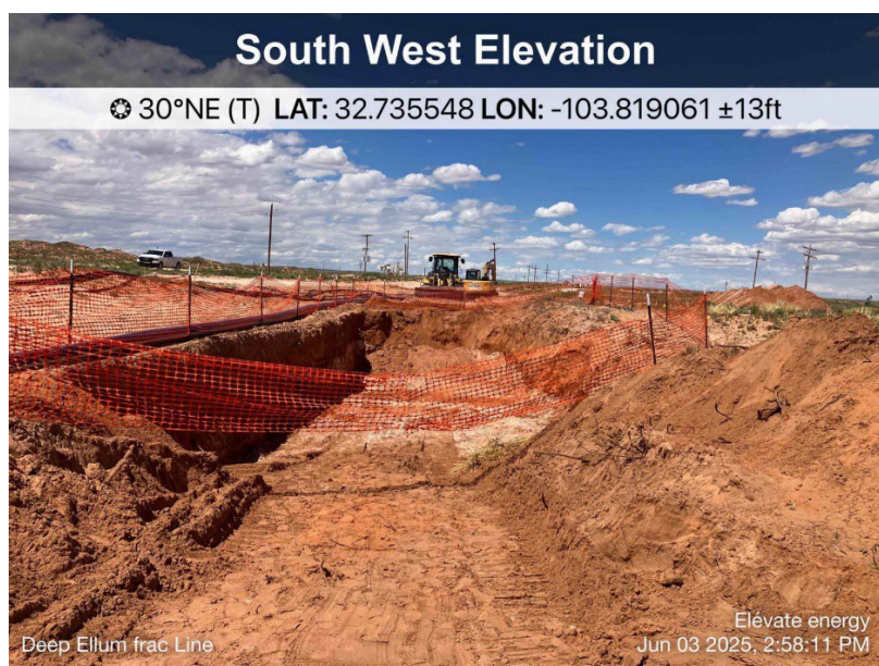
Excavation in Progress
