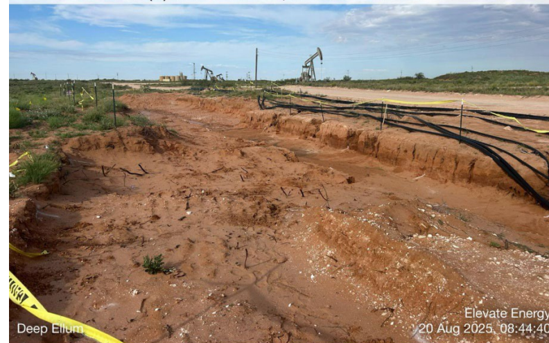
Excavation in Progress
