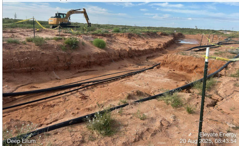
Excavation in Progress
