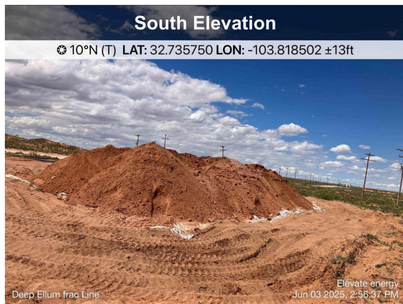
Excavation in Progress
