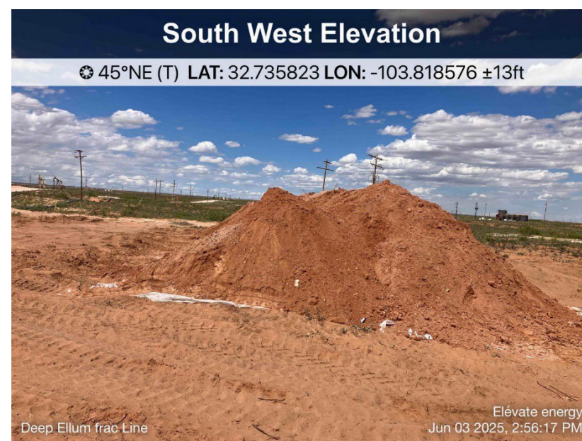
Excavation in Progress
