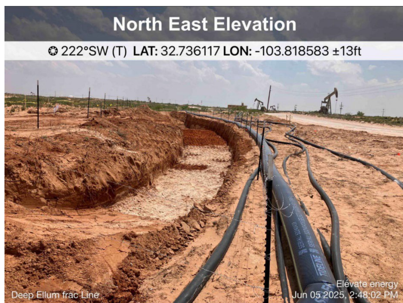
Excavation in Progress
