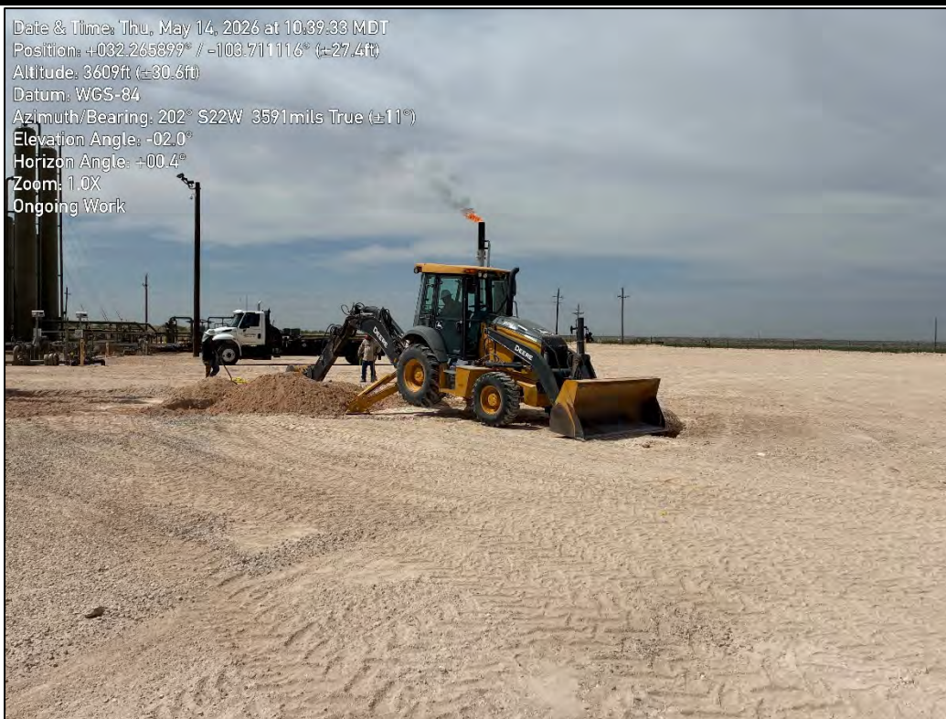
PHOTO 12: Southwestern view during excavation activities. 5/14/2026
