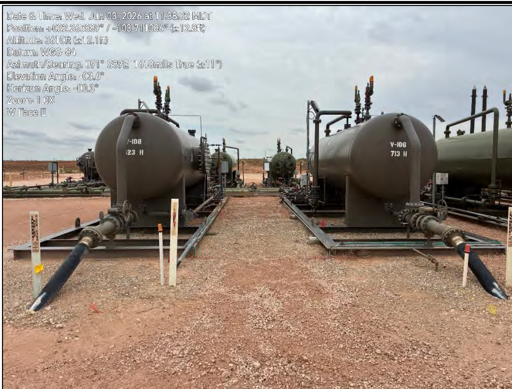
PHOTO 18: Southeastern view following restoration activities. 6/3/2026
