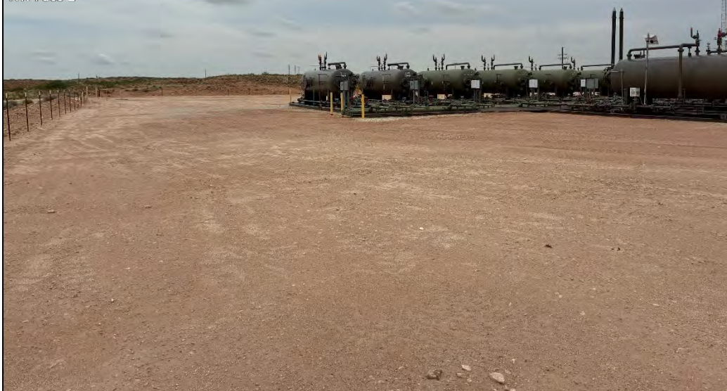
PHOTO 16: Southeastern view following restoration activities. 6/3/2026
