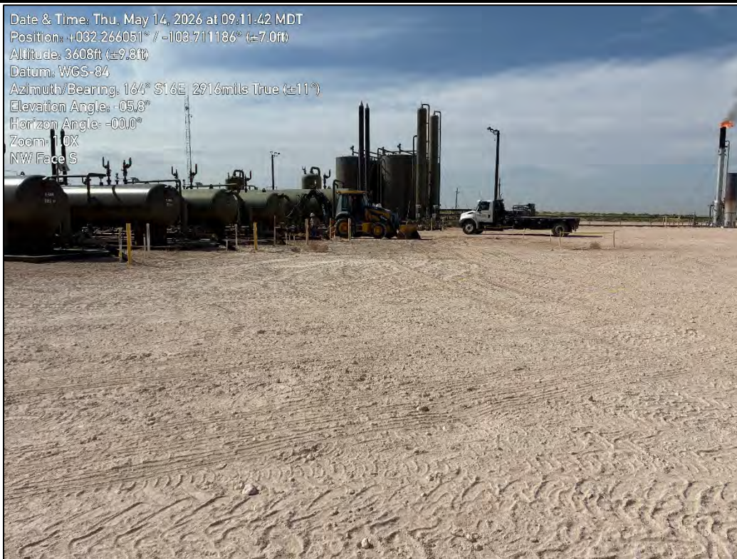
PHOTO 13: Southeastern view during excavation activities. 5/14/2026
